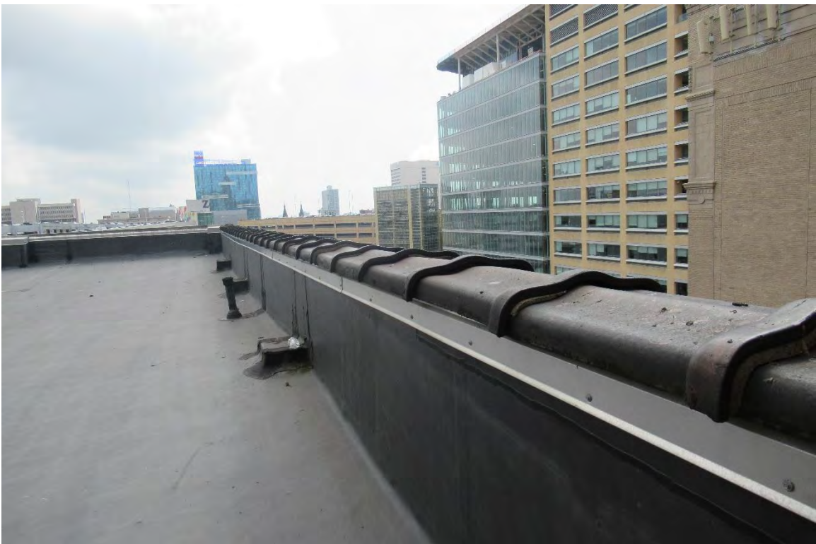
Figure #85: Exterior, Roof, Looking East. 7/17/19
