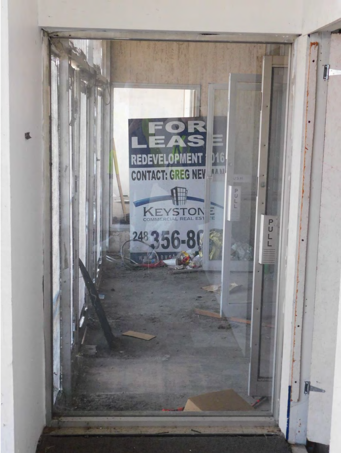
Figure #50: Interior, 1 st Floor Storefront Window into Vestibule, Looking South. 10/15/19
