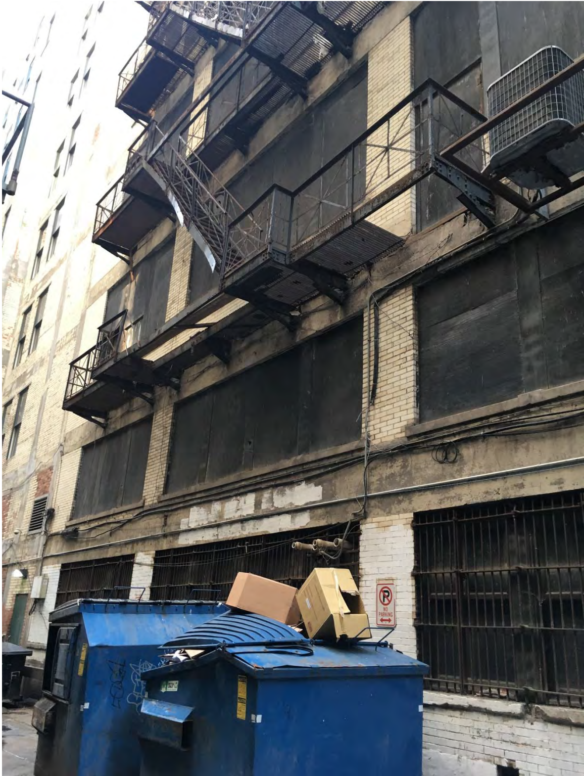
Figure #34: Exterior, Alley, Looking Northeast. 5/31/19
