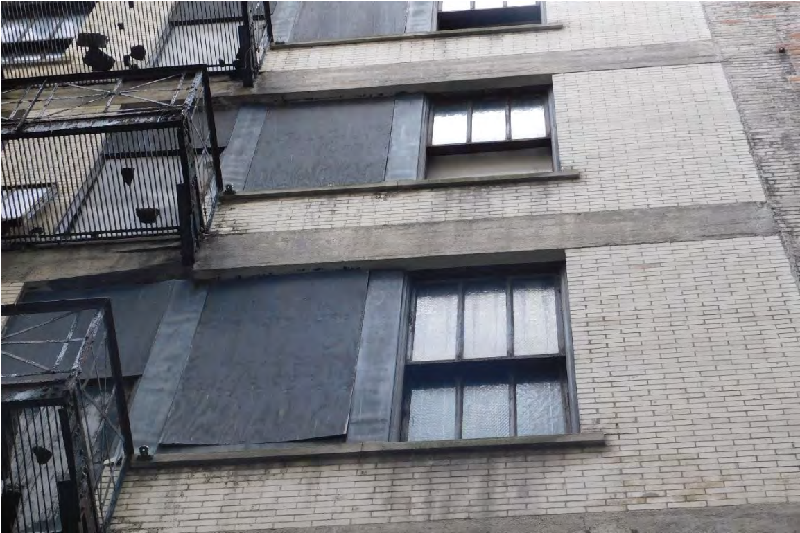
Figure #46: Exterior, Alley Façade, Looking Up. 10/15/19
