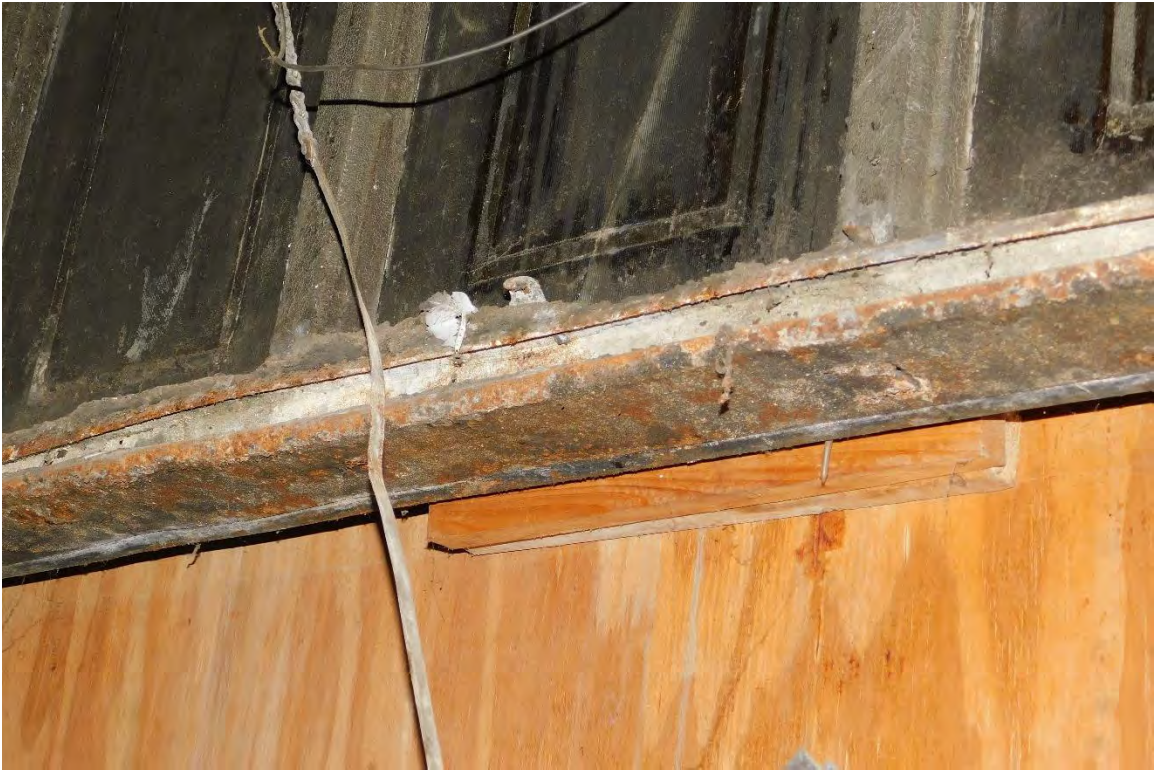
Figure #72: Interior, 4 th floor, Window Detail. 10/15/19
