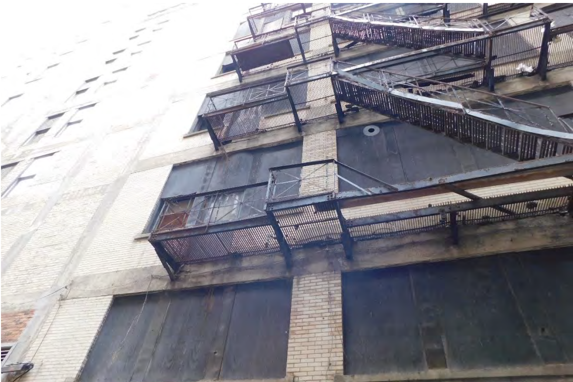
Figure #41: Exterior, Alley Façade, Looking Up. 10/15/19
