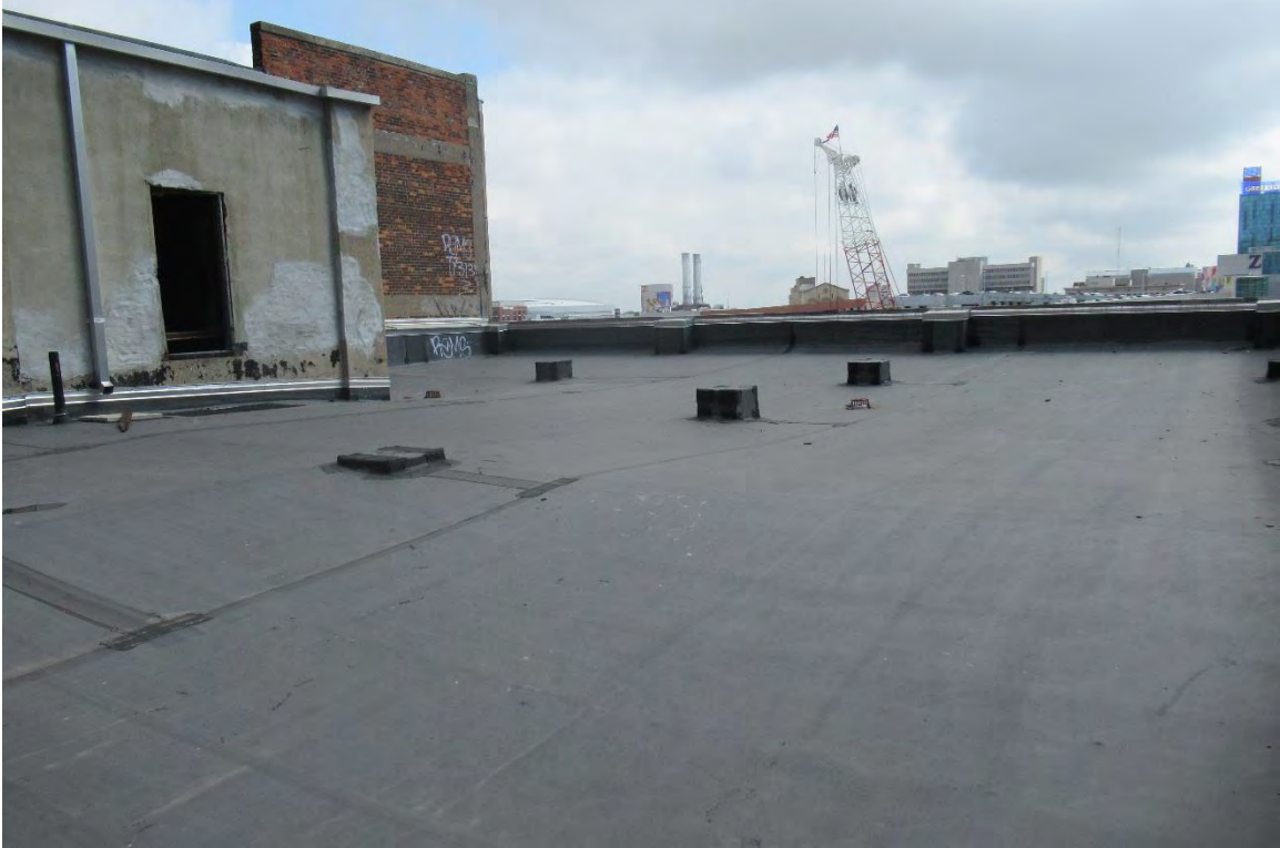
Figure #86: Exterior, Roof, Looking East. 7/17/19
