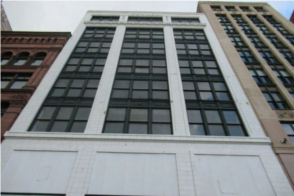
Figure #4: Exterior, Looking up. 7/17/19
