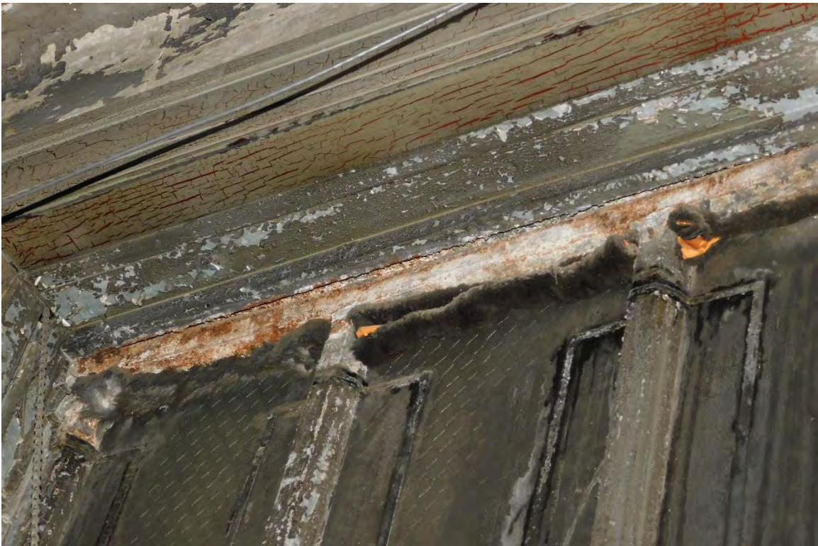
Figure #71: Interior, 4 th floor, Window Detail. 10/15/19
