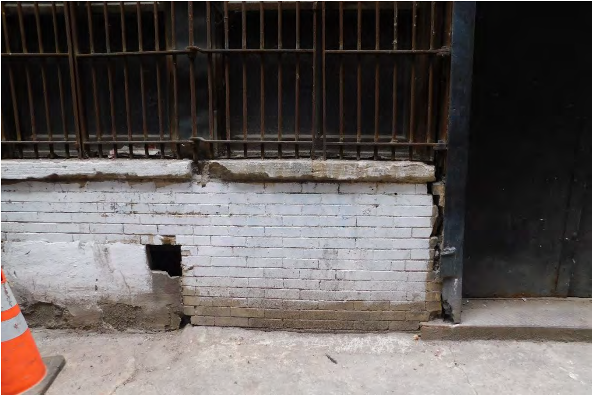
Figure #37: Exterior, Alley Façade Knee Wall, Looking Down. 10/15/19
