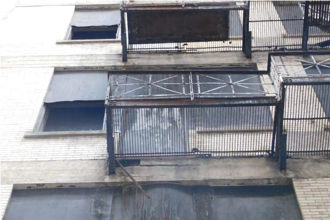
Figure #44: Exterior, Fire Escape, Looking Up. 10/15/19
