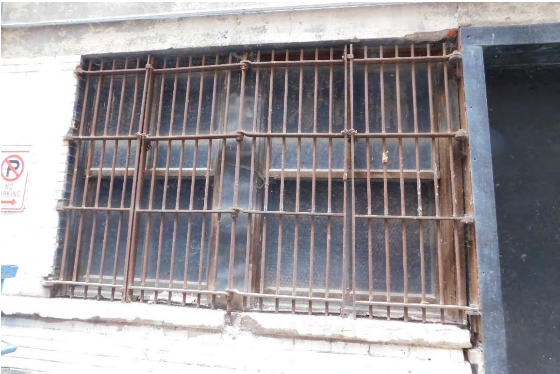
Figure #36: Exterior, Alley Façade Window, Looking East. 10/15/19
