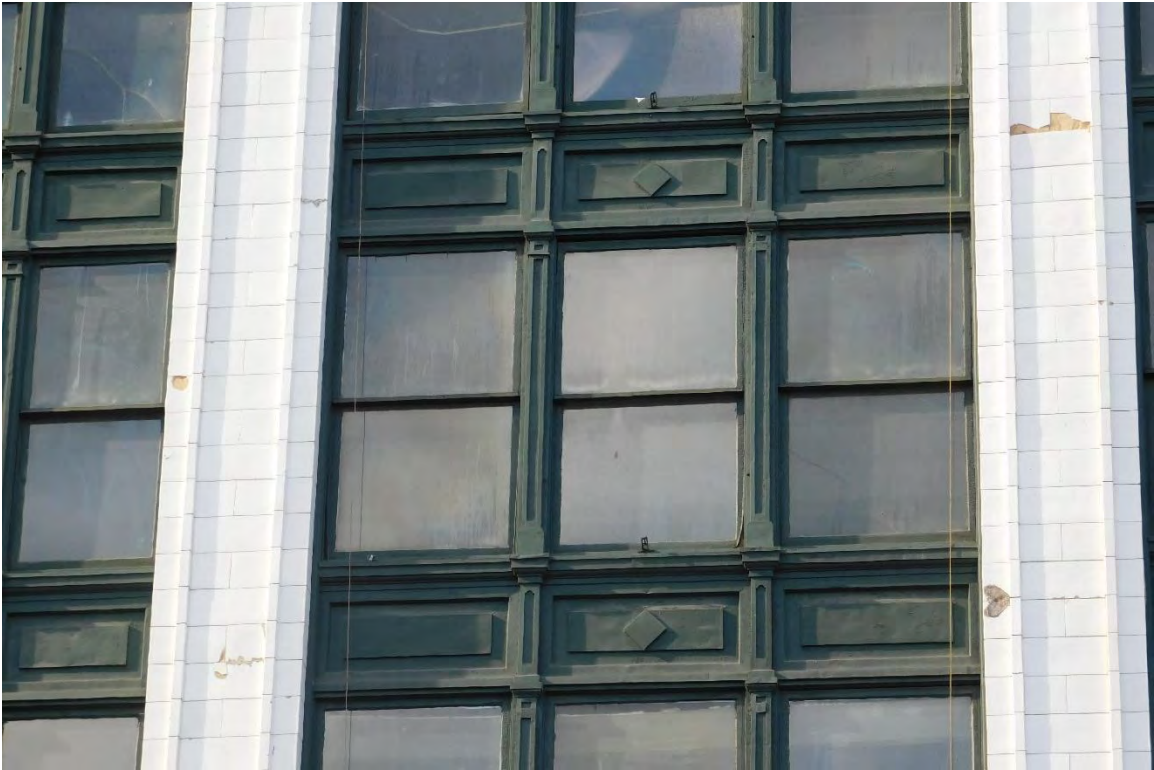
Figure #6: Exterior, Looking West. 10/15/19
