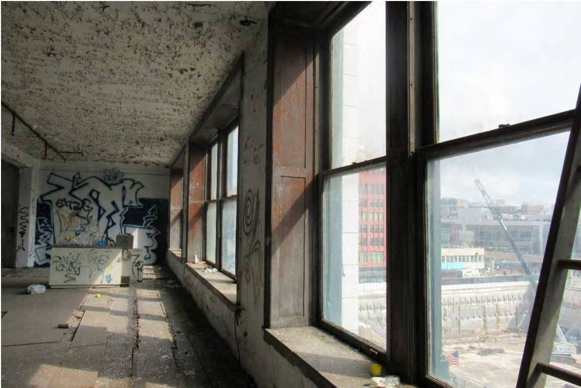
Figure #68: Interior, 4 th floor, Looking Northeast. 5/31/19
