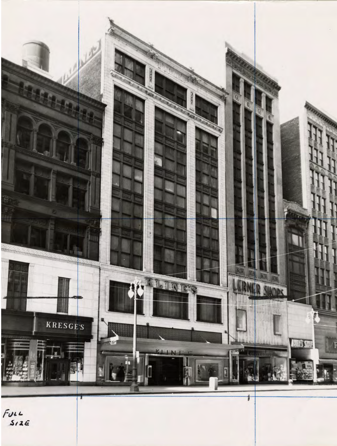
Figure #98: Exterior – Loewy Storefront - 1954
