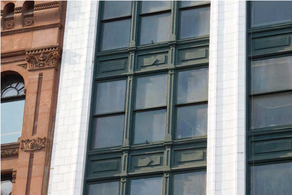
Figure #8: Exterior, Looking West. 10/15/19
