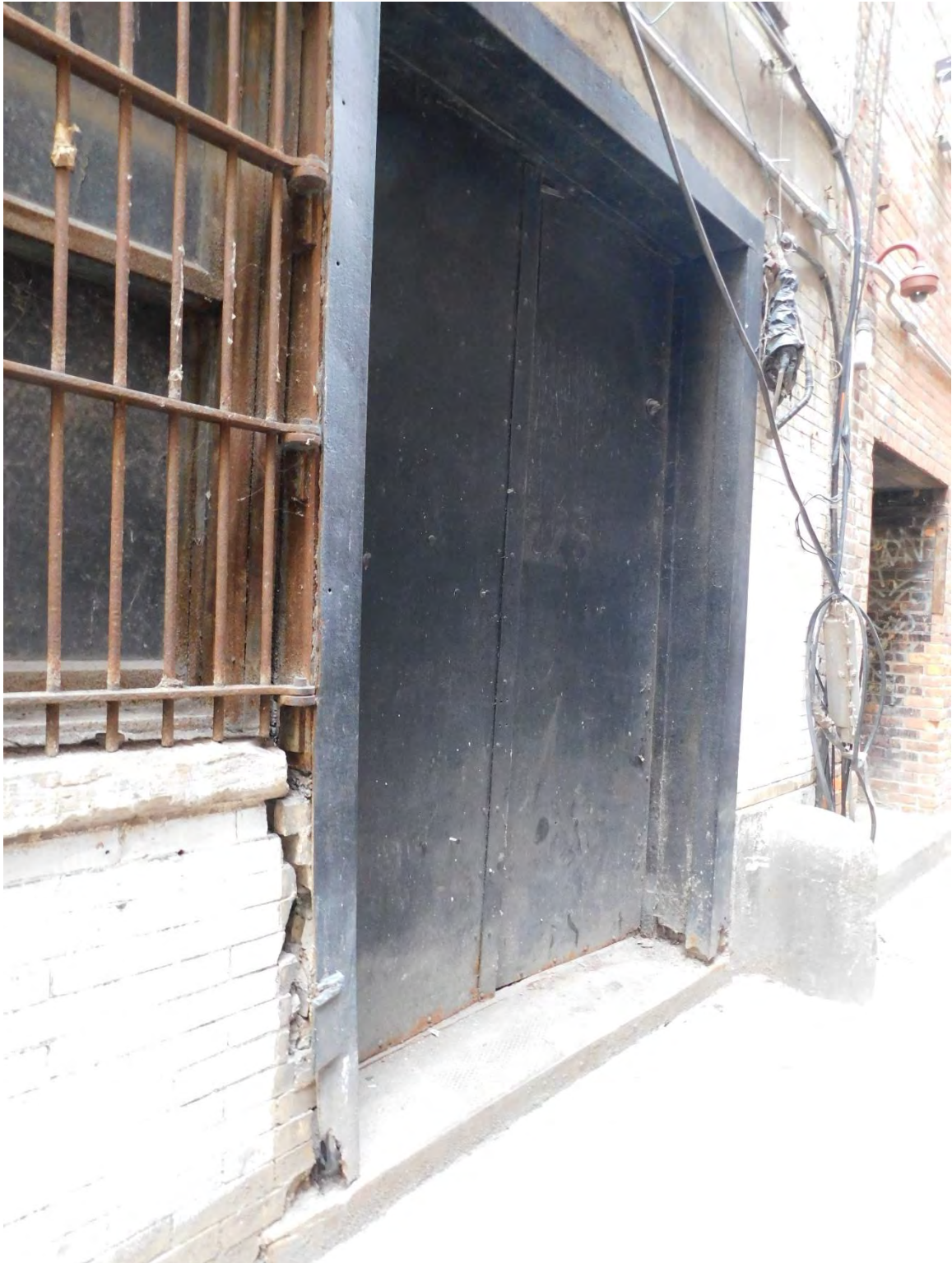
Figure #39: Exterior, Alley Façade Door. 10/15/19
