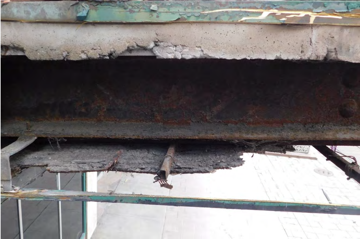
Figure #23: Exterior, Canopy Detail, Looking North. 10/15/19
