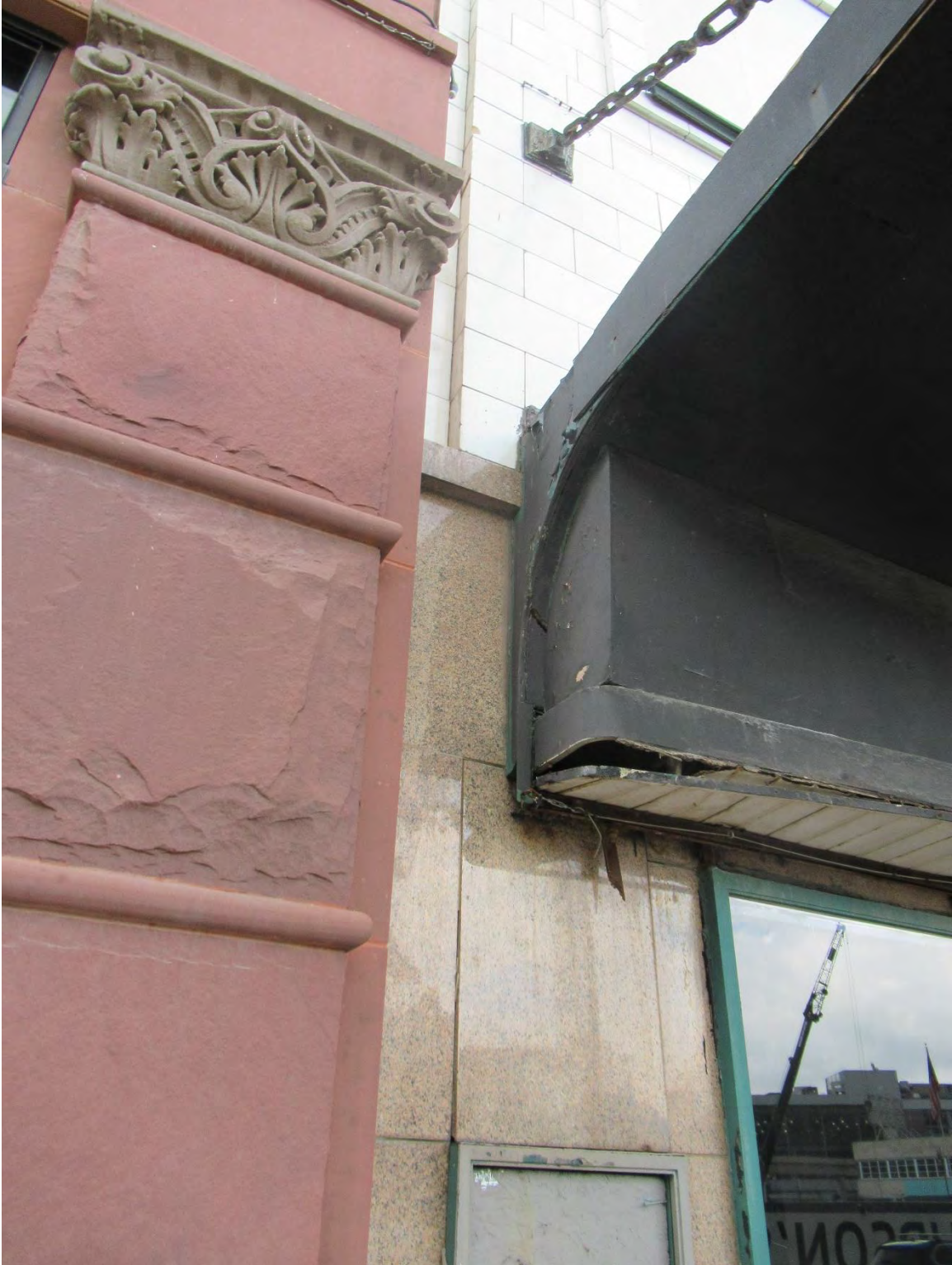
Figure #20: Exterior, Detail, Looking West. 10/15/19
