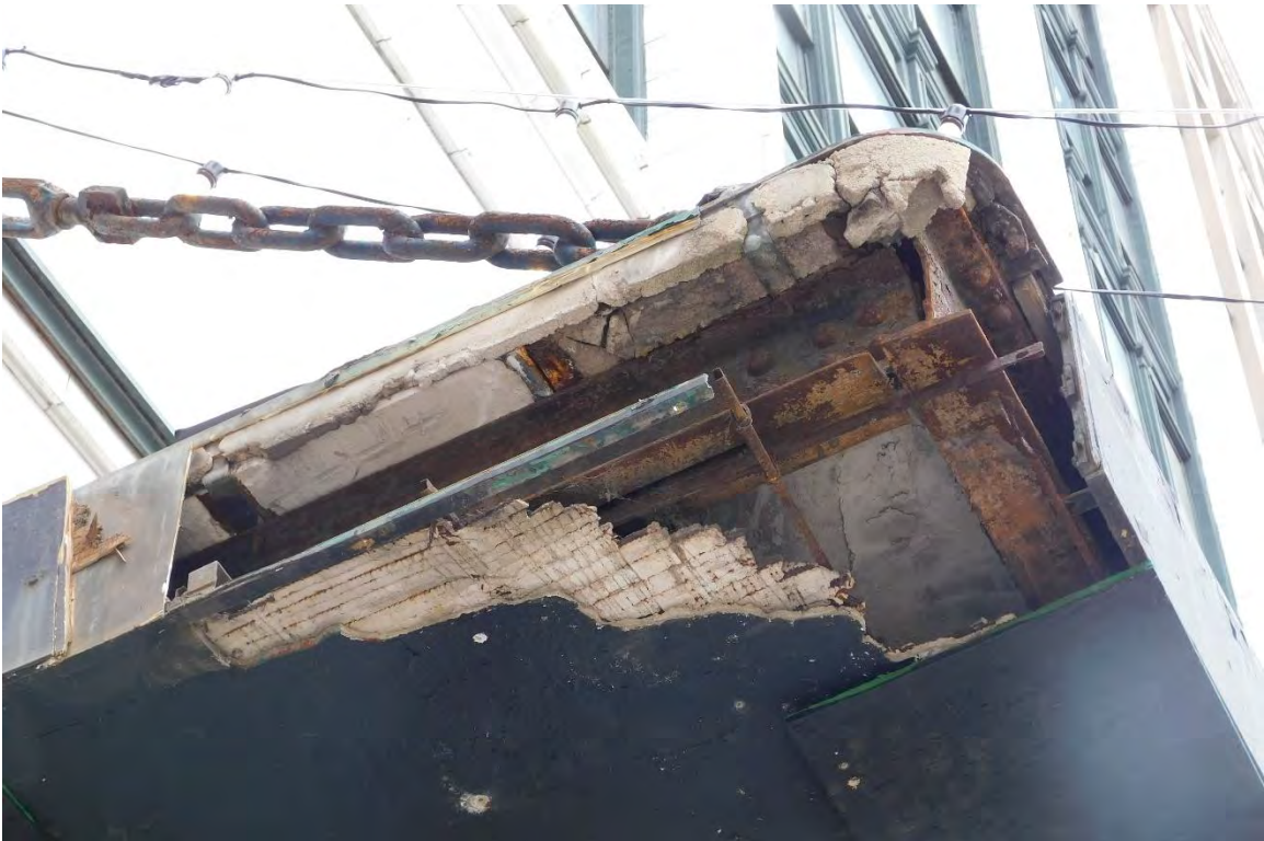
Figure #22: Exterior, Canopy, Looking Up. 10/15/19
