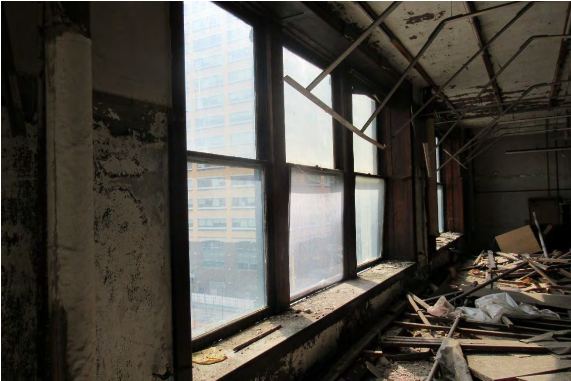
Figure #74: Interior, 5 th floor, Looking southeast. 7/17/19
