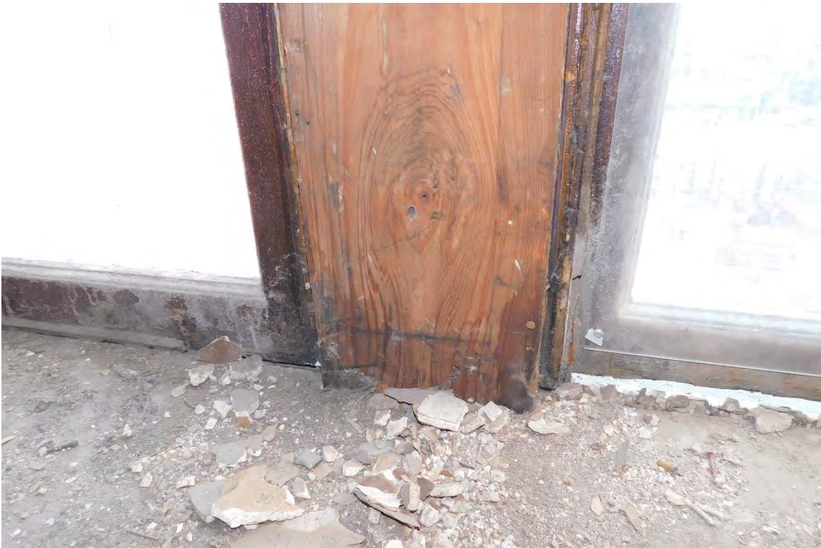
Figure #75: Interior, 5 th floor, Window Detail, Looking Down. 10/15/19
