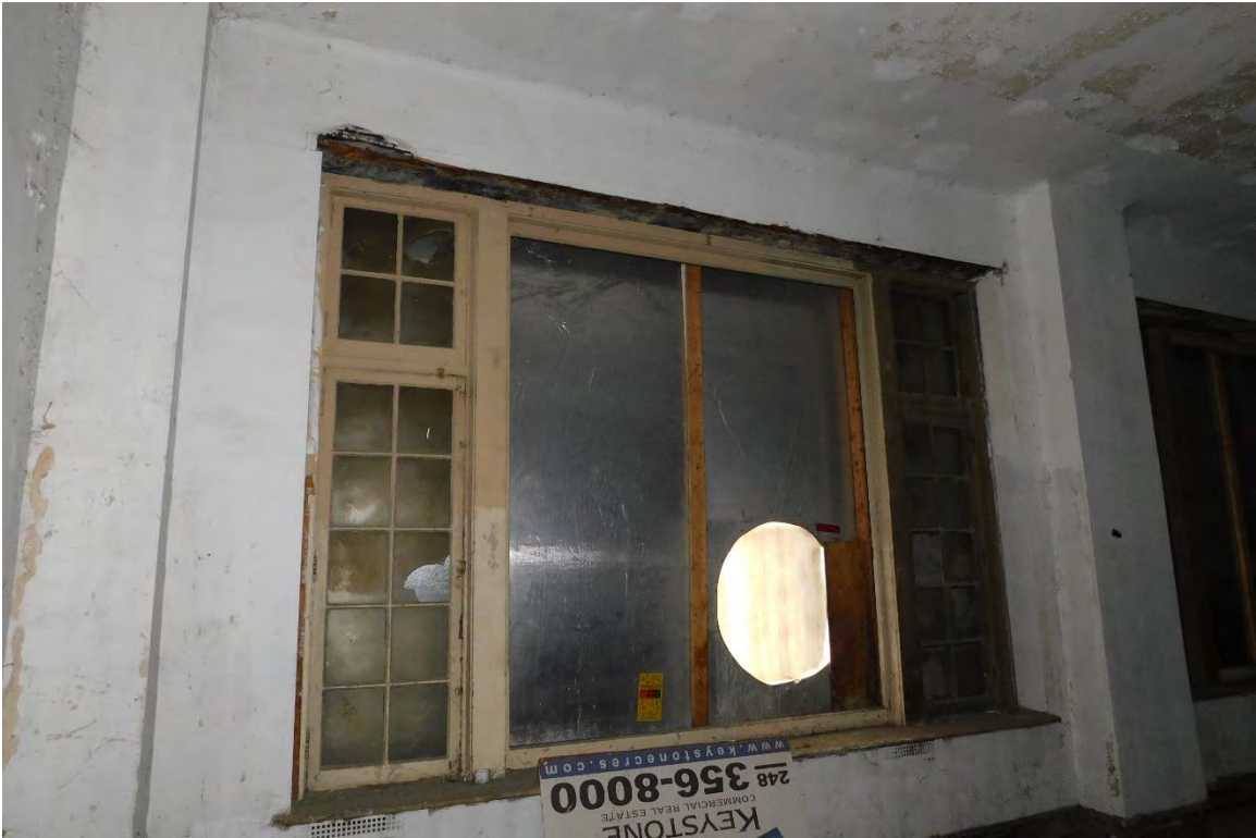
Figure #56: Interior, 2 nd floor, Looking East. 10/15/19
