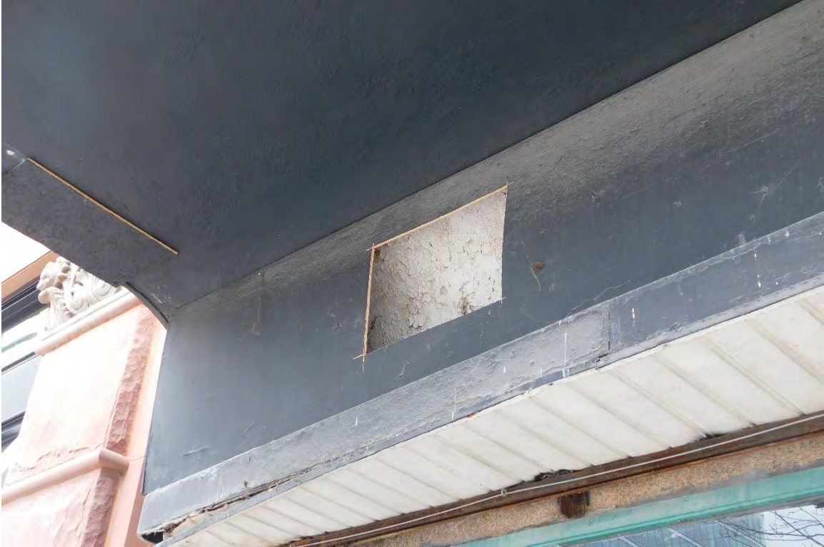
Figure #21: Exterior, Canopy, Looking up. 10/15/19
