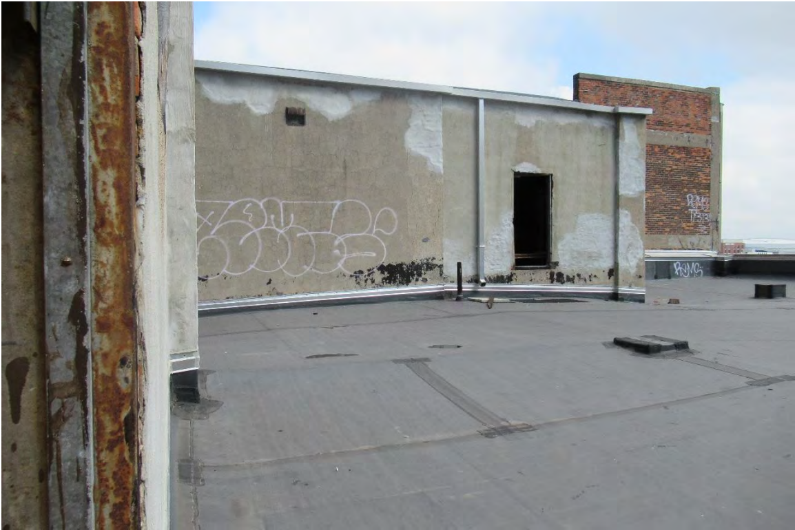
Figure #84: Exterior, Roof, Looking North. 7/17/19
