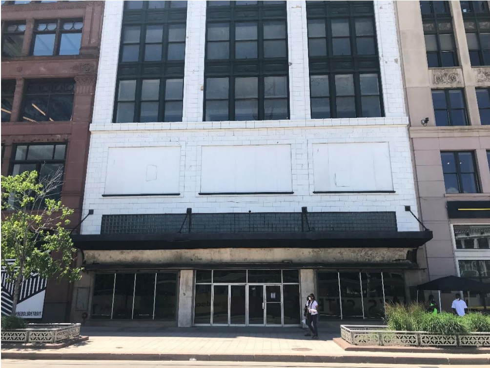
Front of 1225 Woodward, Staff Photo (East Elevation)
