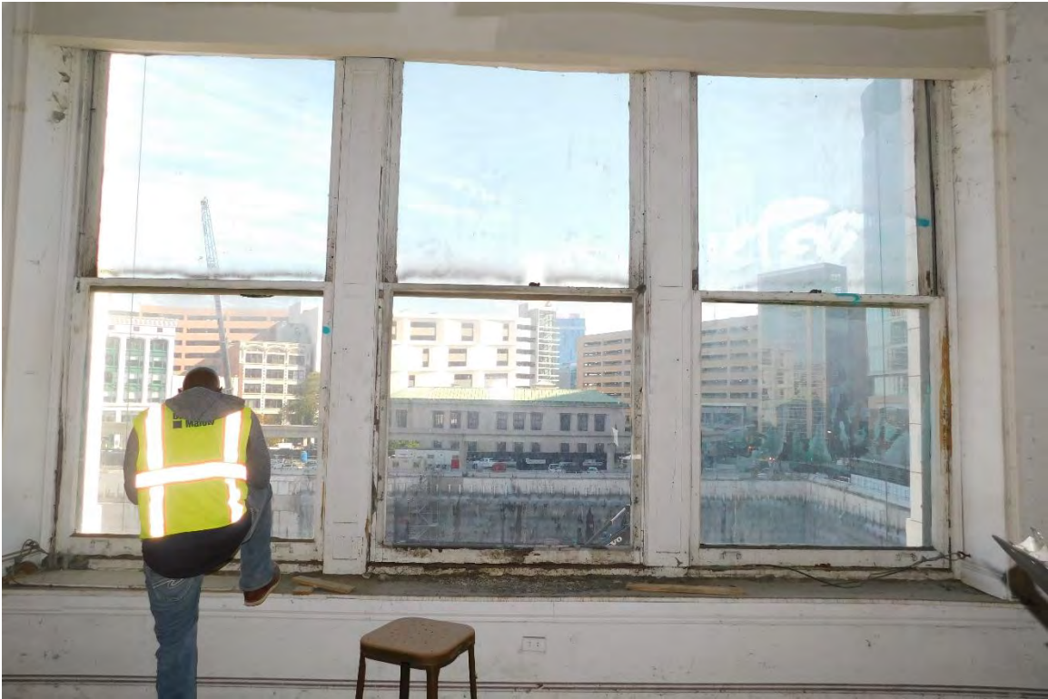
Figure #61: Interior, 3 rd Floor, Looking East. 10/15/19
