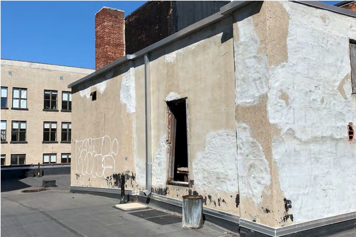
Figure #89: Exterior, Roof and Penthouse, Looking Northwest. 6/12/20
