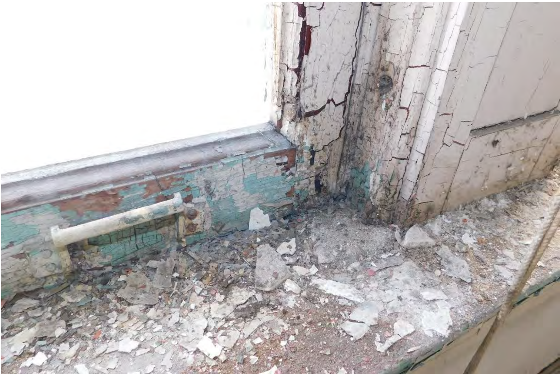
Figure #81: Interior, 8 th floor, Window Detail. 10/15/19
