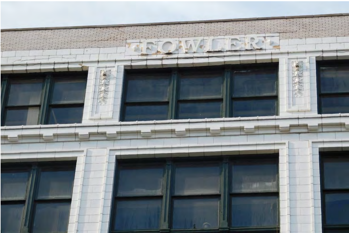
Figure #7: Exterior, Looking Up. 10/15/19
