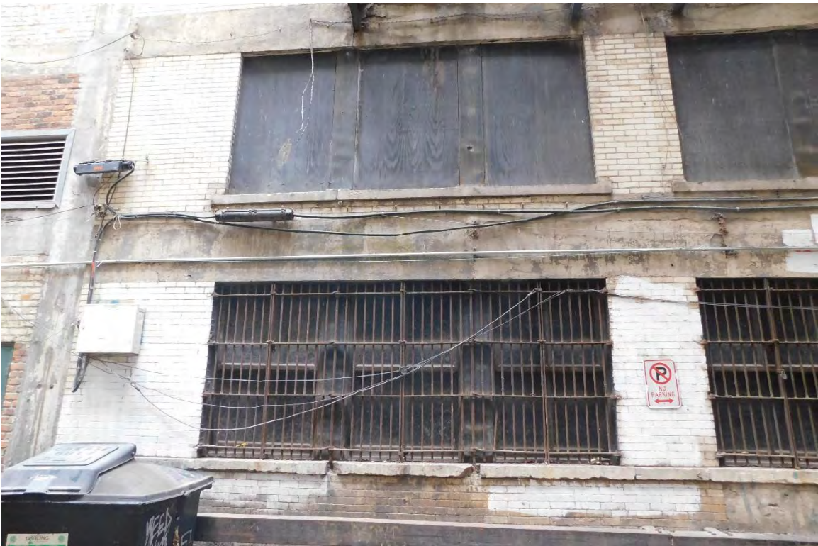
Figure #43: Exterior, Alley Façade, Looking East. 10/15/19
