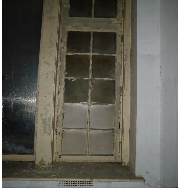
Figure #54: Interior, 2 nd floor, Looking East. 10/15/19
