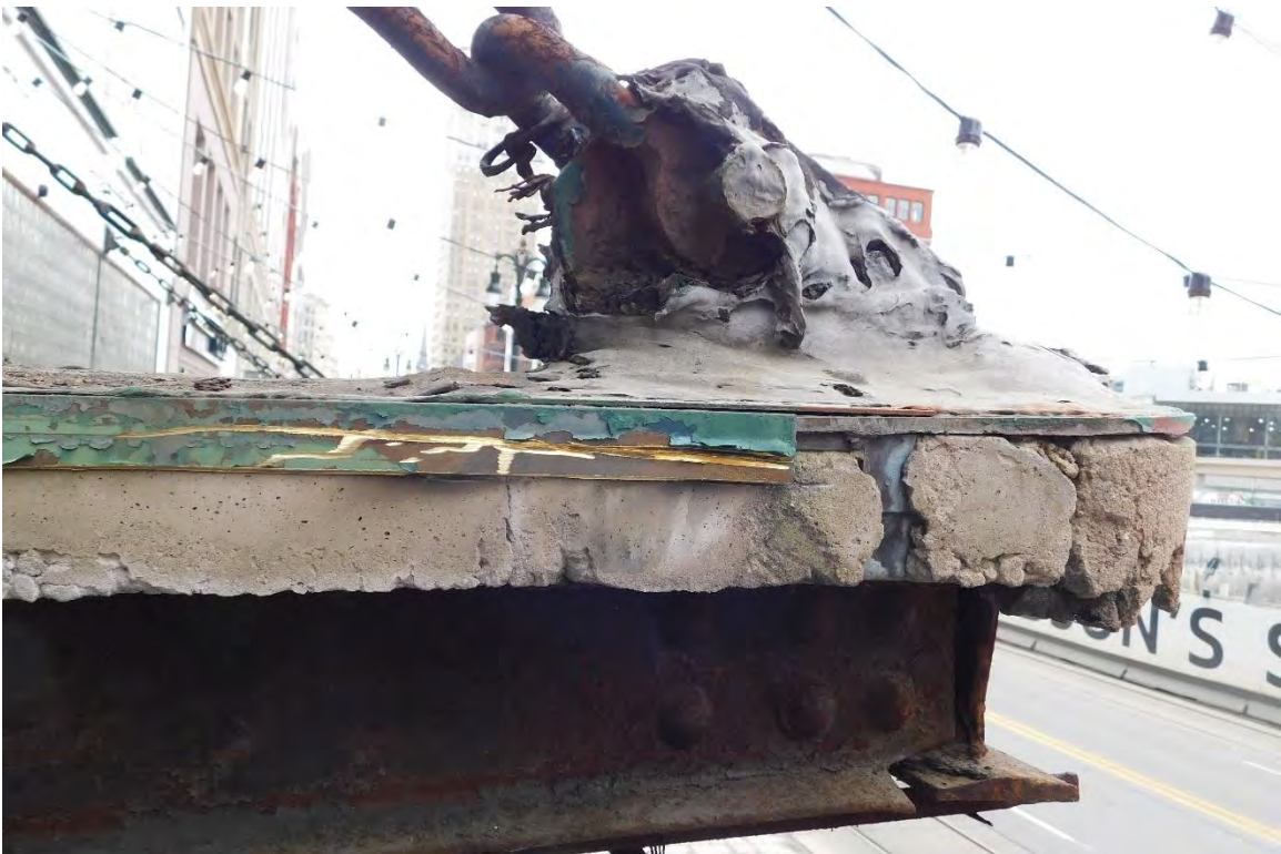
Figure #24: Exterior, Canopy Detail, Looking North. 10/15/19
