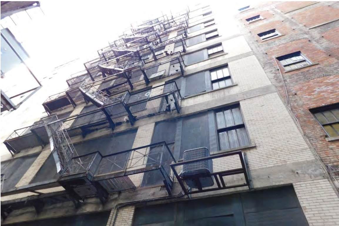
Figure #38: Exterior, Alley Façade, Looking Up. 10/15/19
