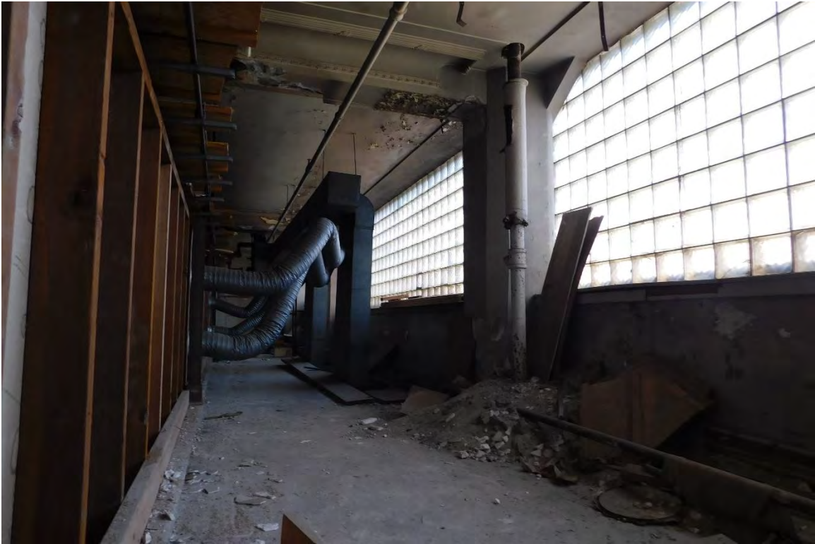
Figure #52: Interior, Mezzanine Glass Block, Looking Northeast. 10/15/19
