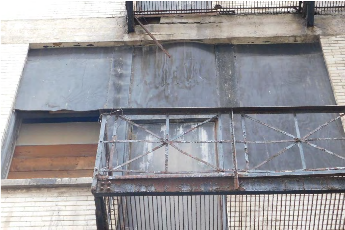
Figure #45: Exterior, Fire Escape, Looking Up. 10/15/19
