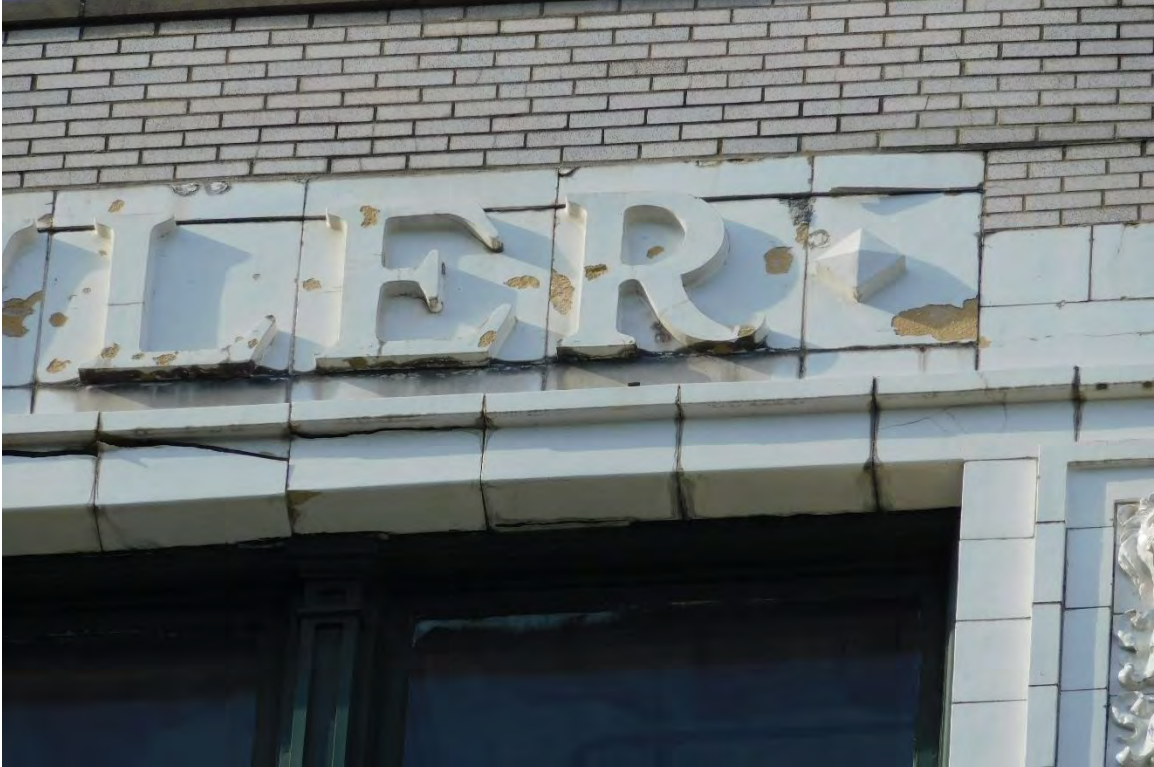
Figure #10: Exterior, Detail, Looking Up. 10/15/19
