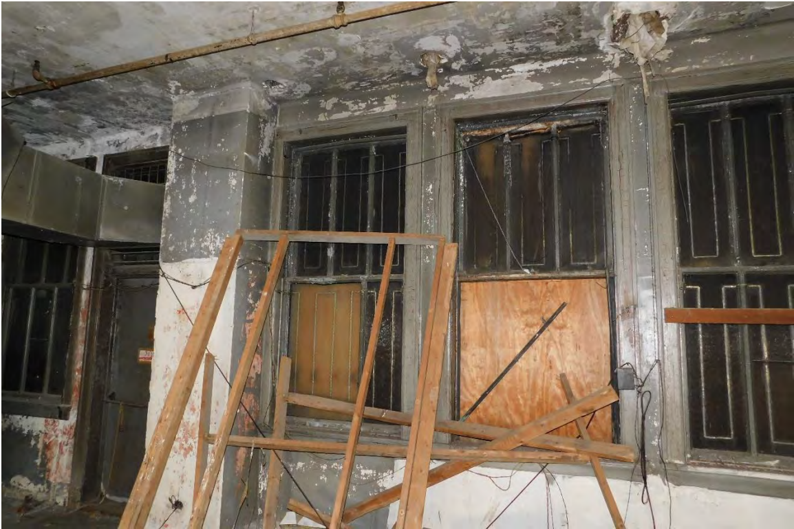
Figure #70: Interior, 4 th floor, Looking East. 10/15/19
