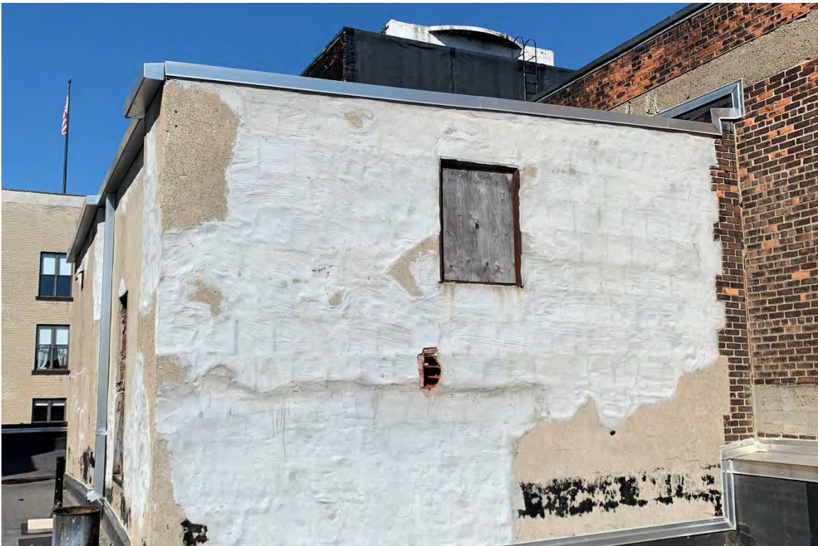
Figure #90: Exterior, Penthouse and Roof, Looking West. 6/12/20
