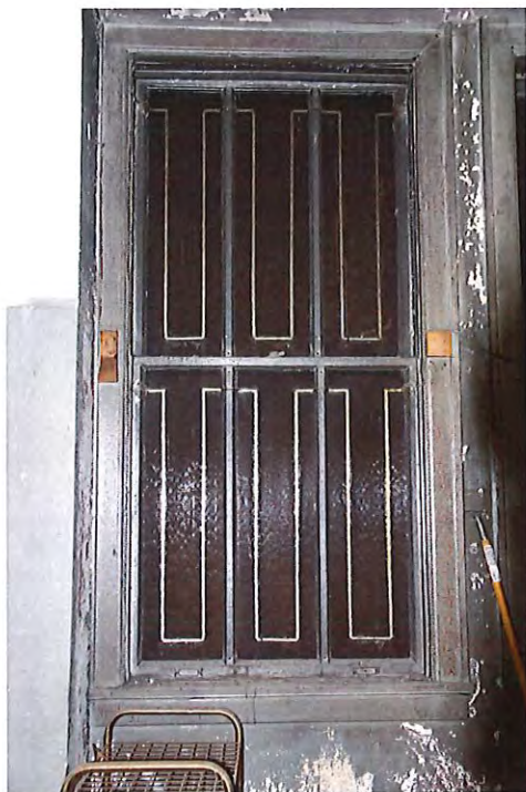
Interior of Steel Double Hung
