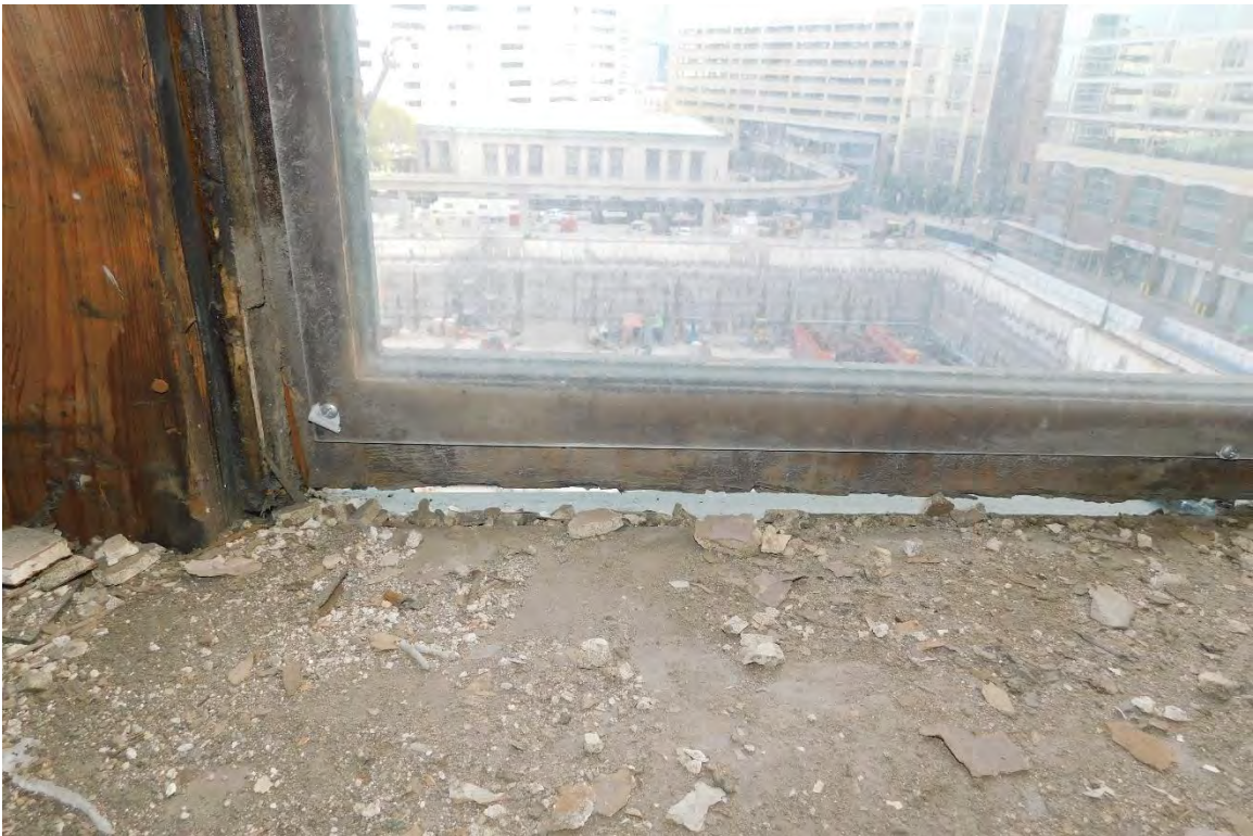
Figure #73: Interior, 5 th floor, Window Detail, Looking East. 10/15/19
