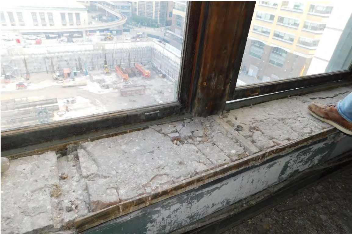
Figure #79: Interior, 7 th floor, Looking Down. 10/15/19
