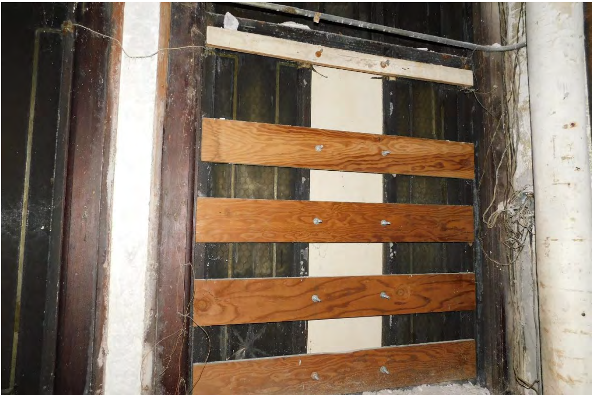
Figure #83: Interior, 8 th floor, Window Detail. 10/15/19
