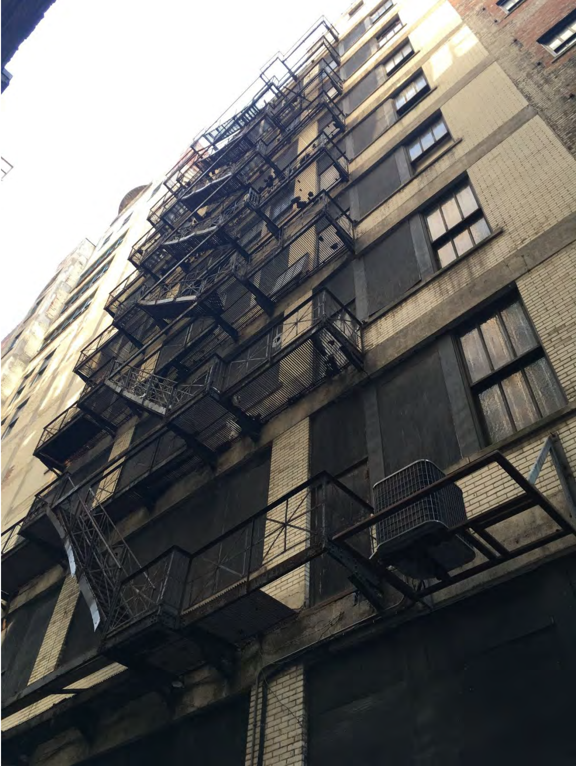
Figure #33: Exterior, Alley, Looking Up. 5/31/19
