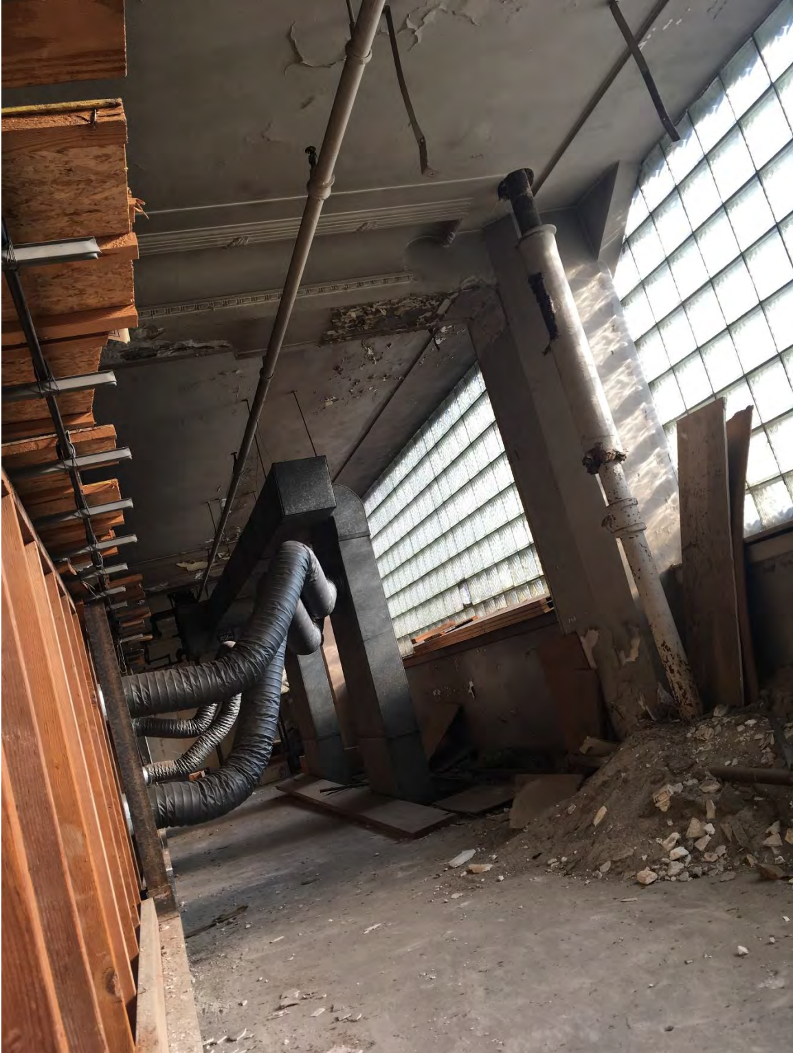
Figure #51: Interior, Mezzanine Windows, Looking Northeast. 5/31/19
