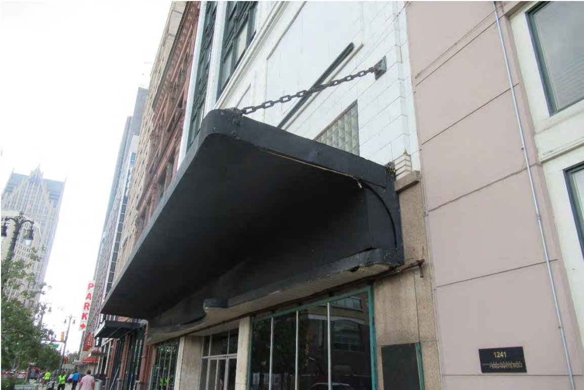
Figure #18: Exterior, Looking Up. 7/17/19
