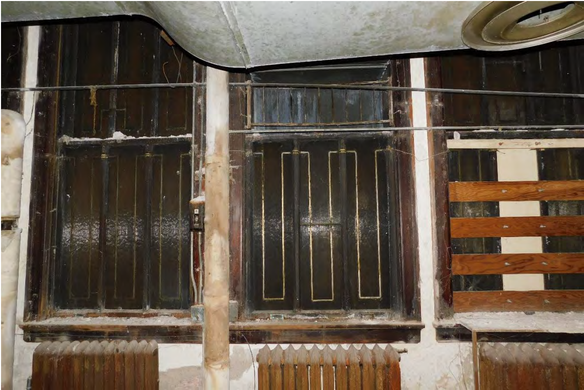
Figure #82: Interior, 8 th floor, Looking West. 10/15/19
