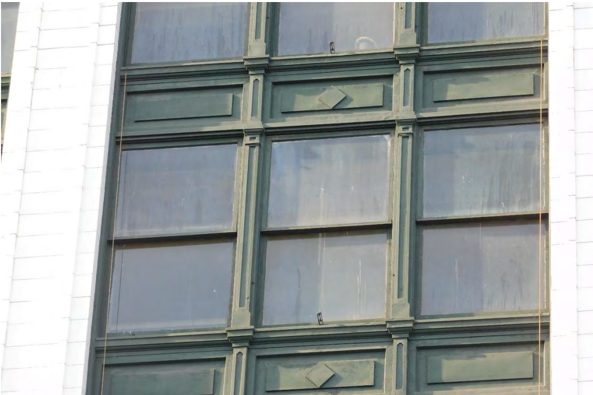
Figure #9: Exterior, Looking West.. 10/15/19
