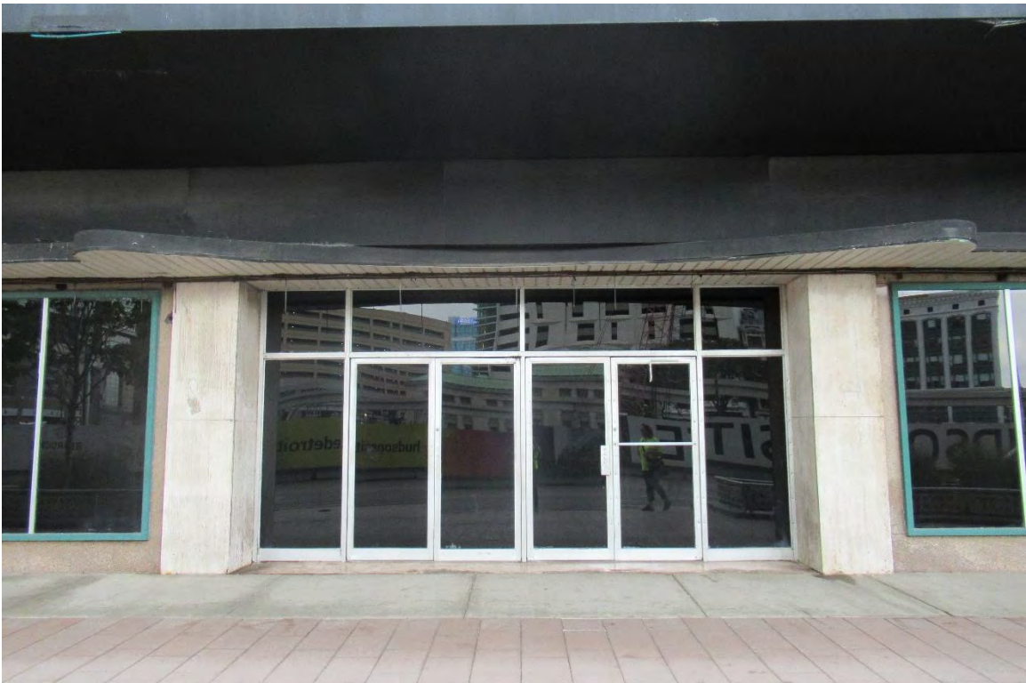
Figure #5: Exterior, Looking West. 7/17/19
