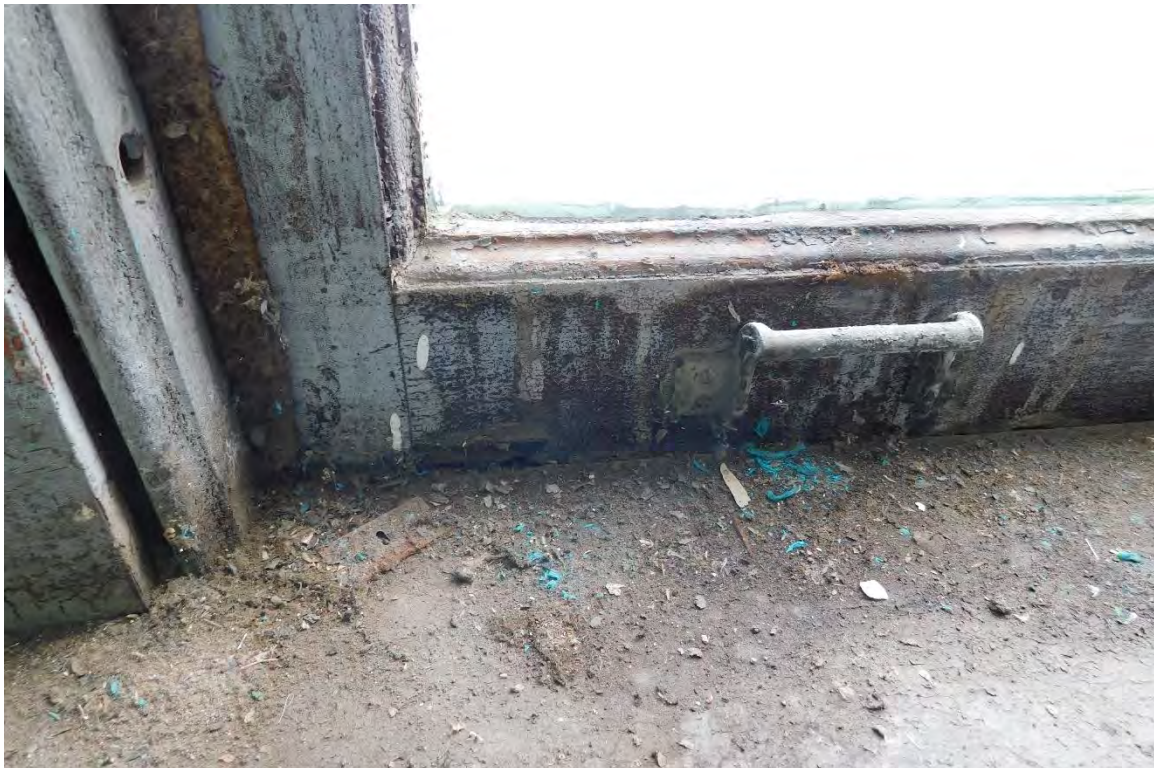
Figure #69: Interior, 4 th floor, Window Detail. 10/15/19
