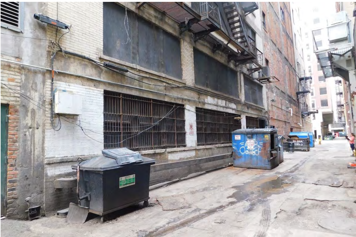
Figure #32: Exterior, Alley and West Façade, Looking Southeast. 10/15/19
