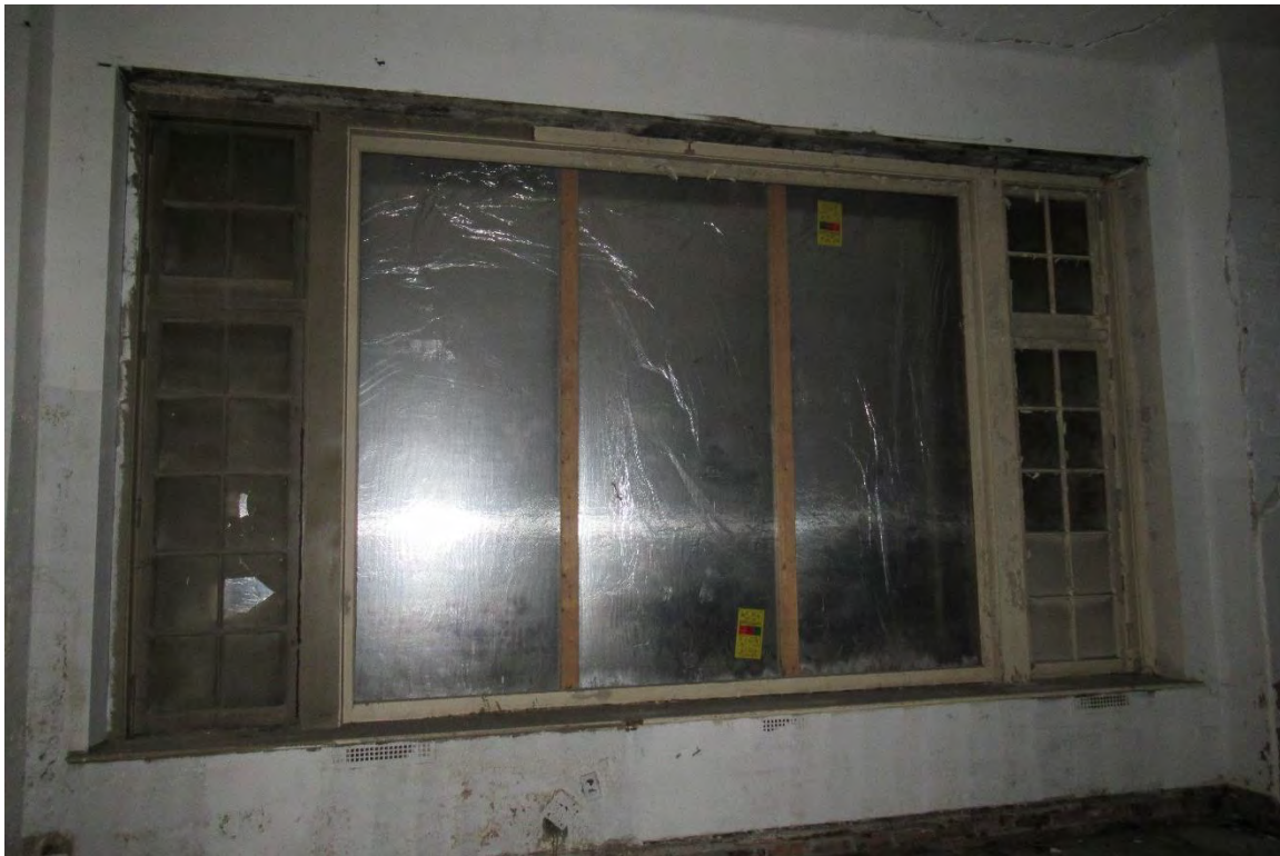
Figure #55: Interior, 2 nd floor, Looking East. 7/17/19
