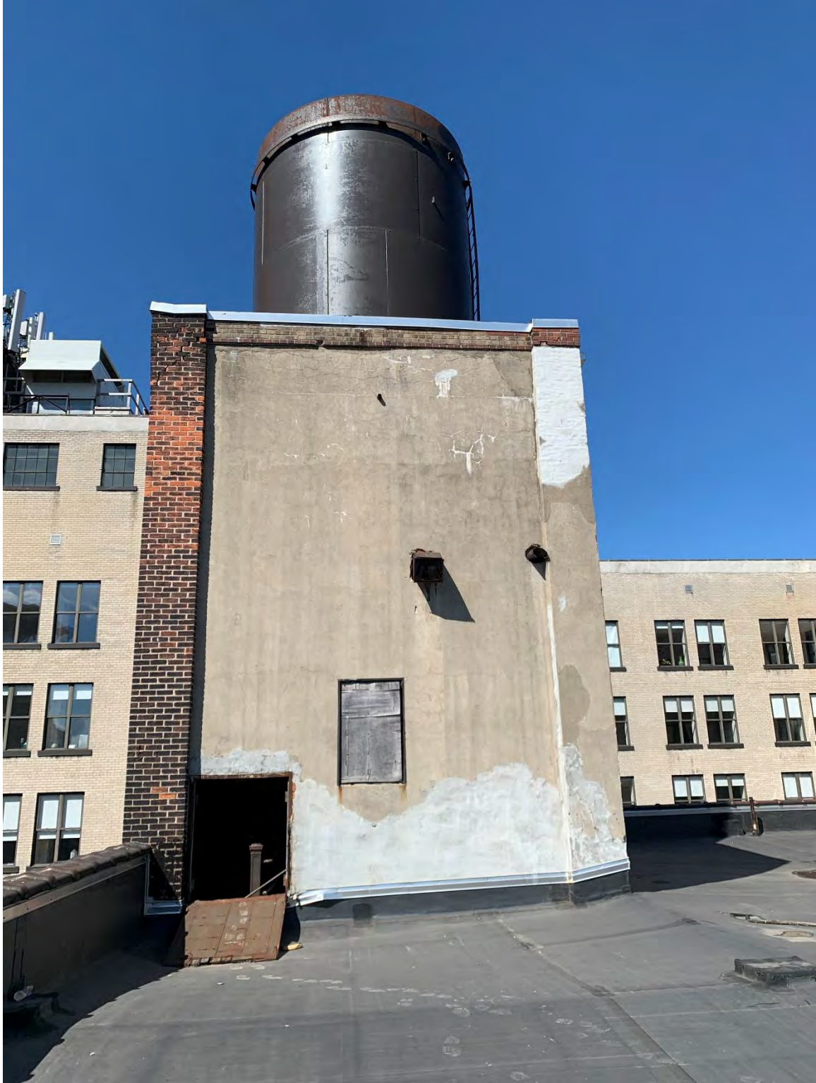
Figure #88: Exterior, Water tower, Looking up. 6/12/20
