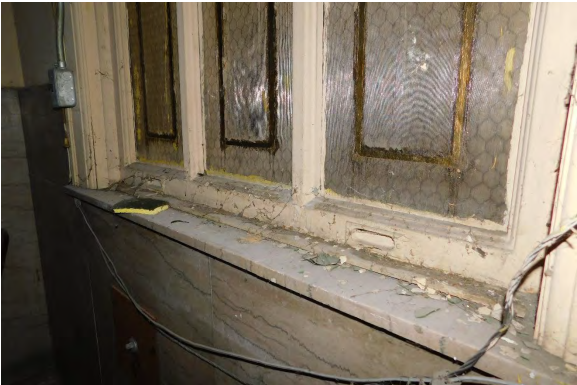
Figure #59: Interior, 2 nd floor, Window Detail. 10/15/19
