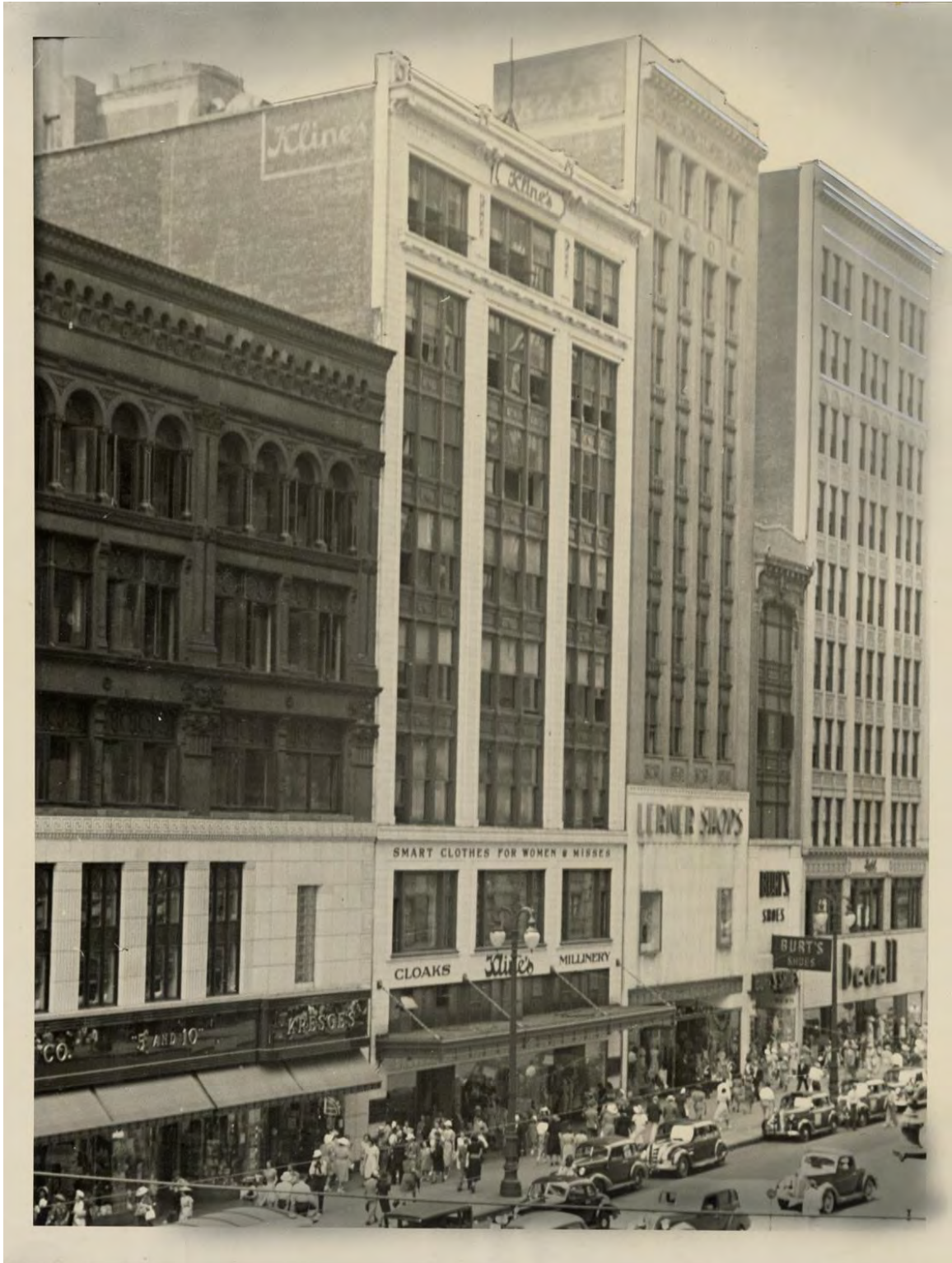
Figure #95: Exterior – Date Unknown
