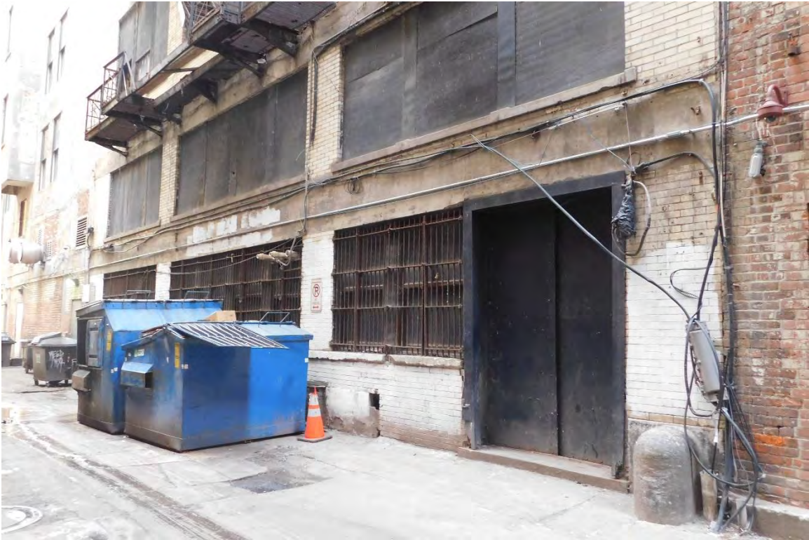
Figure #35: Exterior, Alley Façade, Looking Northeast. 10/15/19
