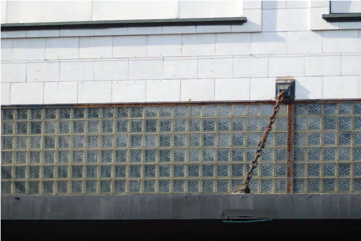
Figure #14: Exterior, Detail, Looking West. 10/15/19
