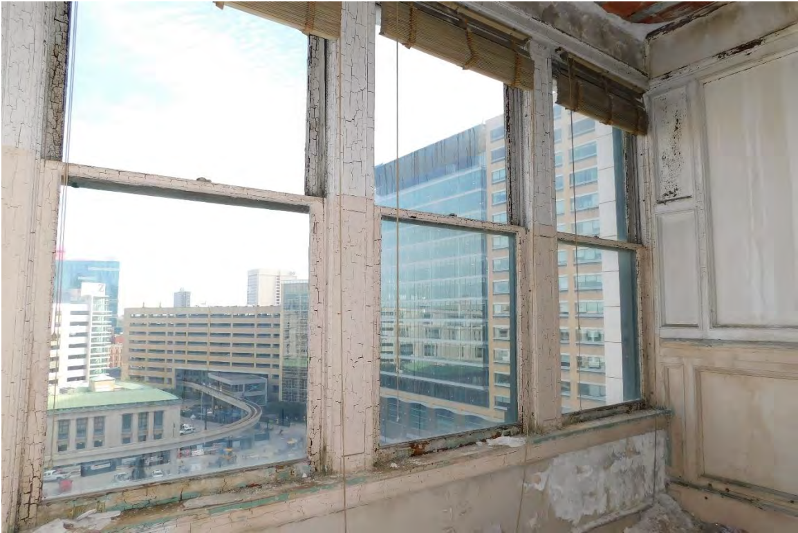
Figure #80: Interior, 8 th floor, Looking Southeast. 10/15/19
