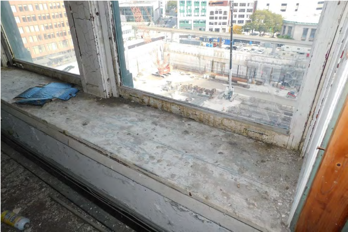
Figure #78: Interior, 7 th floor, Window Detail. 10/15/19
