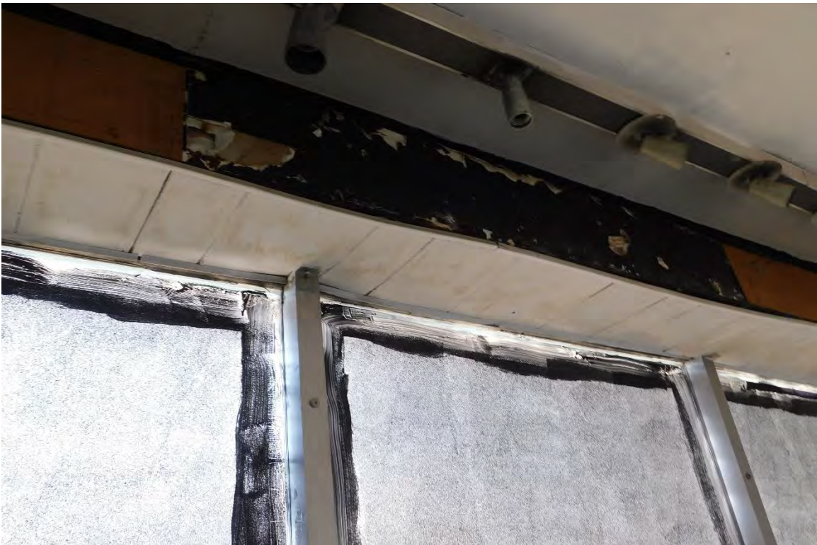
Figure #49: Interior, 1 st Floor Storefront, Looking Up. 10/15/19
