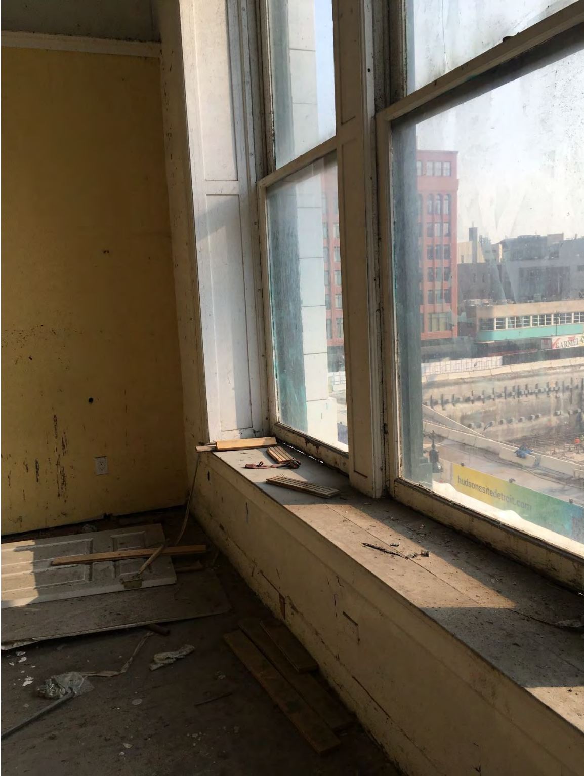
Figure #60: Interior, 3 rd floor, Window Detail, Looking Northeast. 5/31/19
