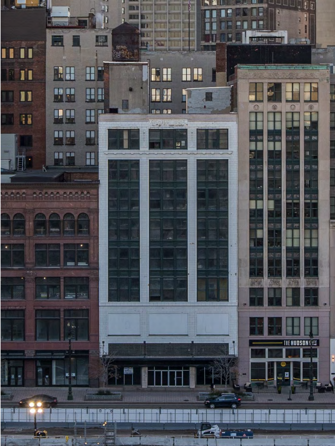
Figure #1: Exterior, Looking West. 5/31/19
