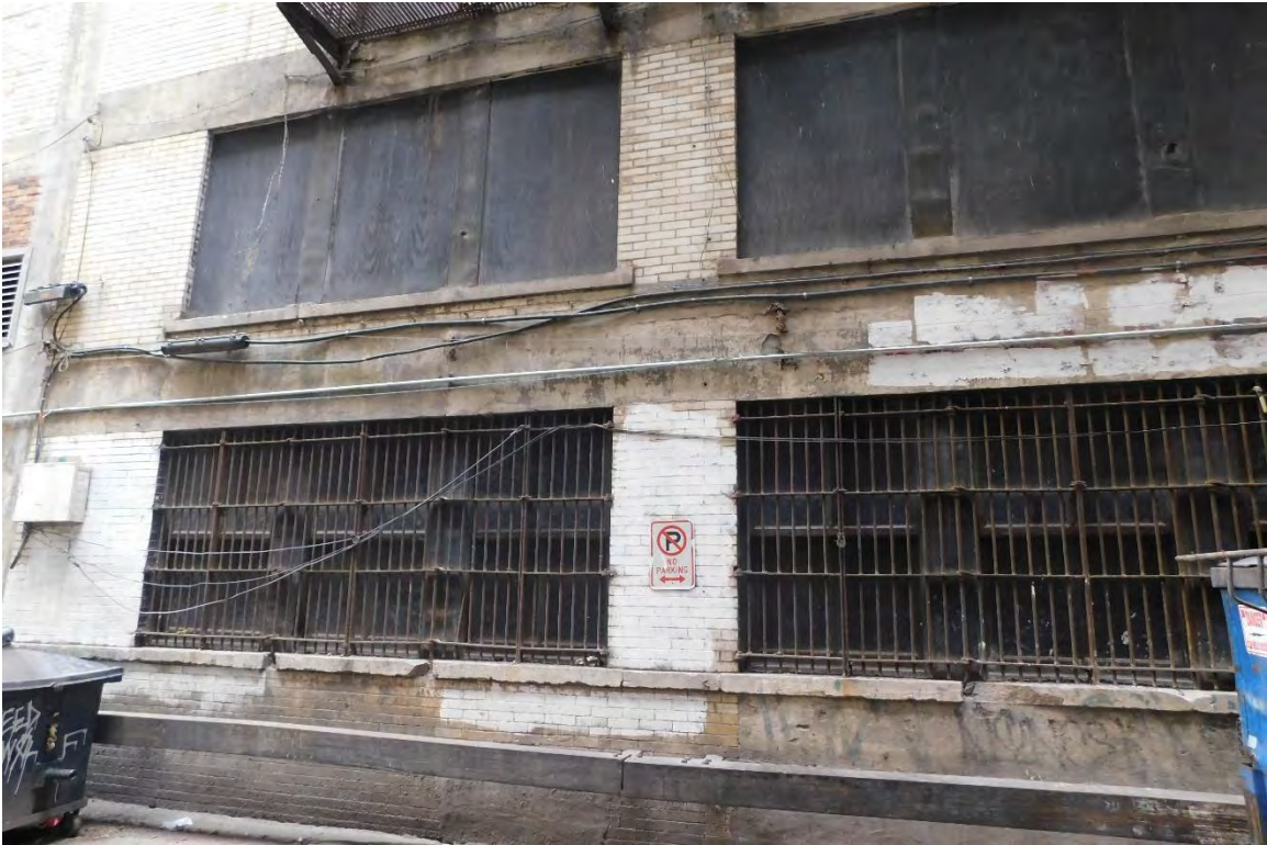
Figure #40: Exterior, Alley façade windows, Looking East. 10/15/19
