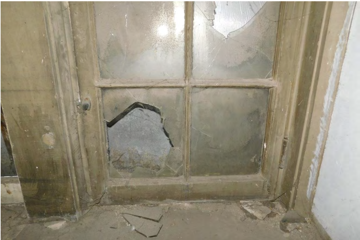
Figure #57: Interior, 2 nd floor, Window Detail. 10/15/19
