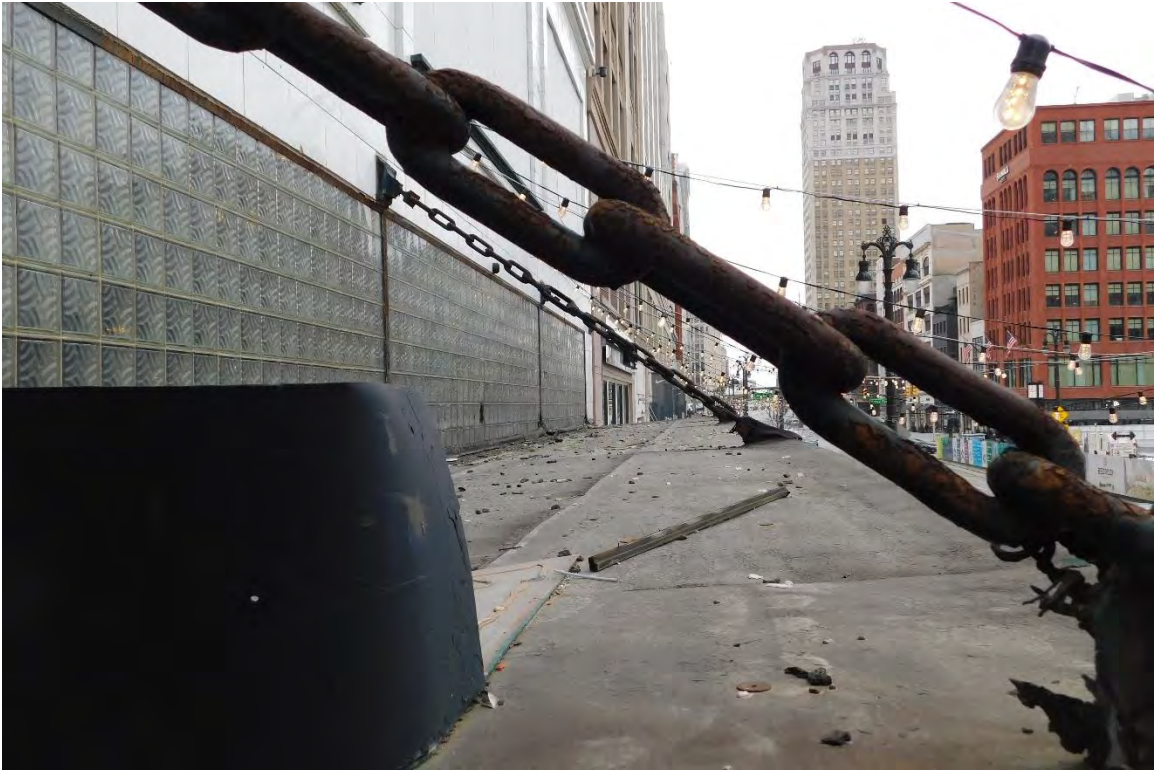
Figure #25: Exterior, Canopy, Looking North. 10/15/19
