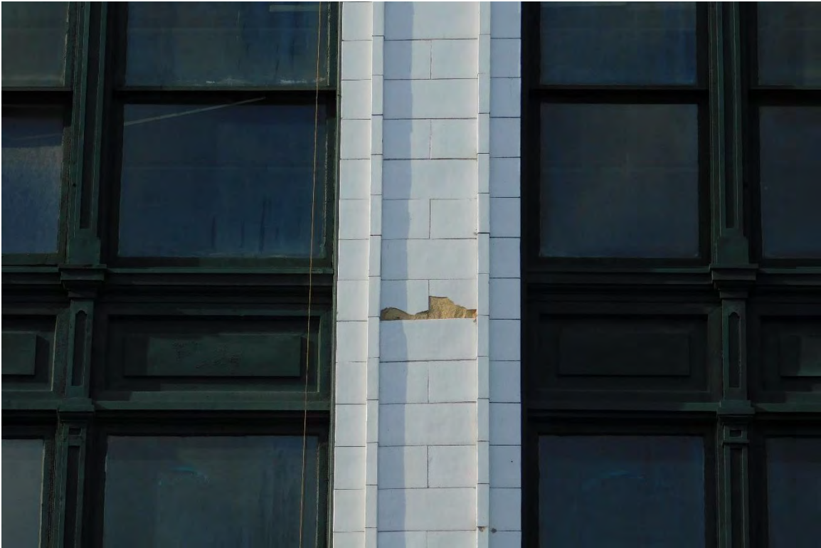
Figure #12: Exterior, Detail, Looking West. 10/15/19
