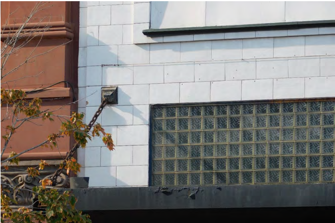
Figure #15: Exterior, Detail, Looking West. 10/15/19
