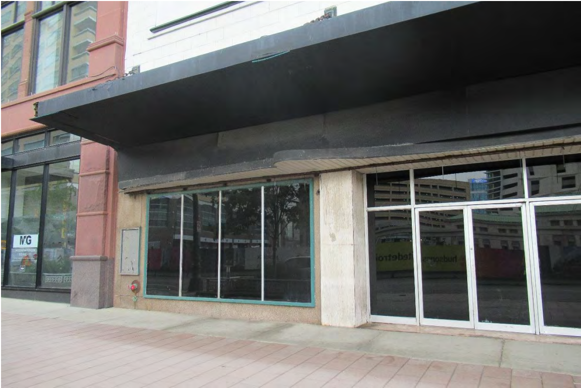
Figure #16: Exterior, Looking Southwest. 7/17/19
