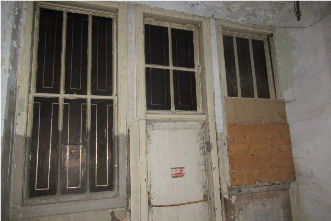
Figure #58: Interior, 2 nd floor, Looking West. 7/17/19
