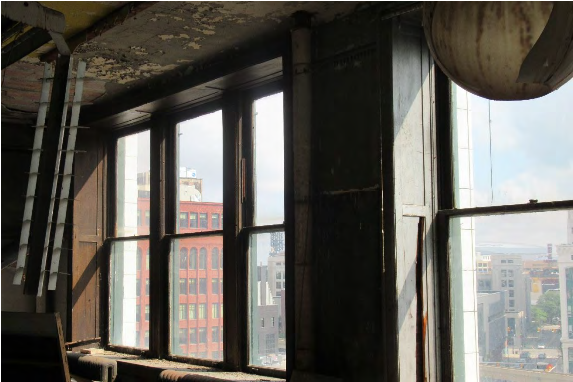
Figure #76: Interior, 6 th floor, Looking Northeast. 7/17/19
