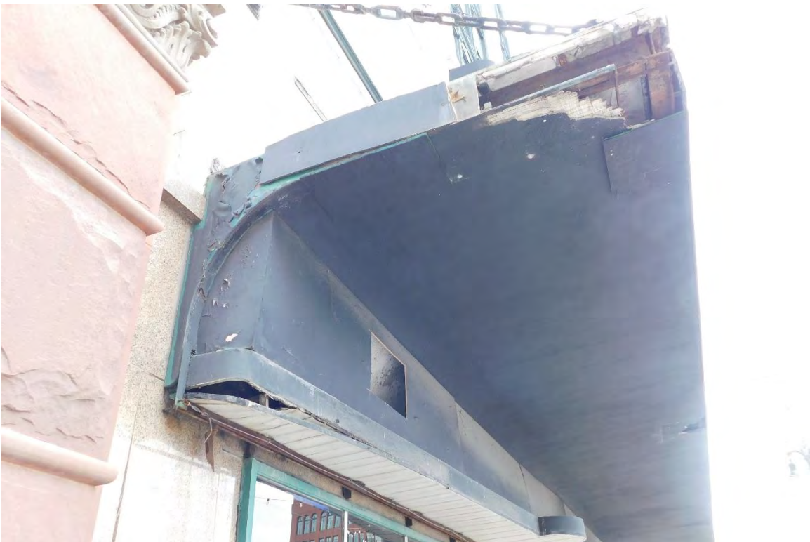
Figure #26: Exterior, Canopy, Looking Northwest. 7/17/19
