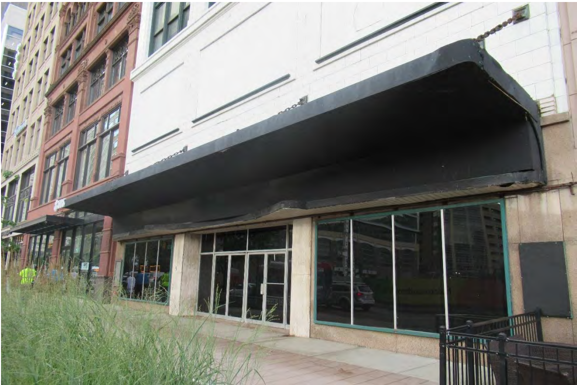
Figure #17: Exterior, Looking Southwest. 7/17/19
