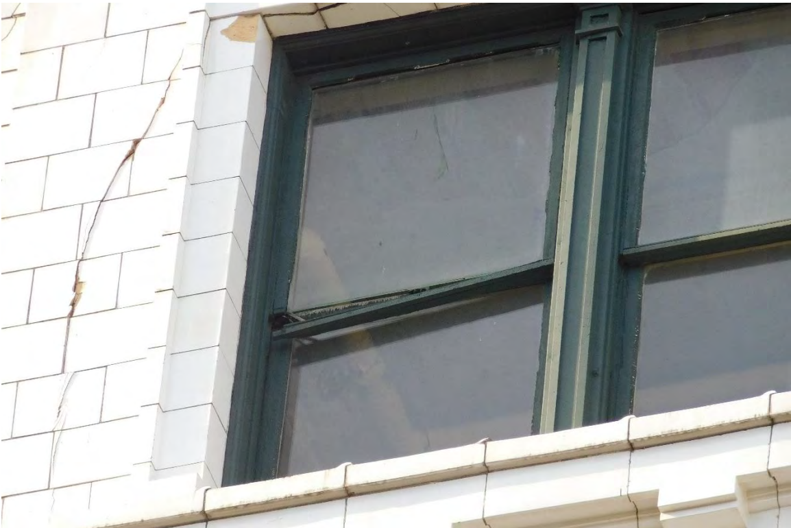
Figure #11: Exterior, Looking Up. 10/15/19
