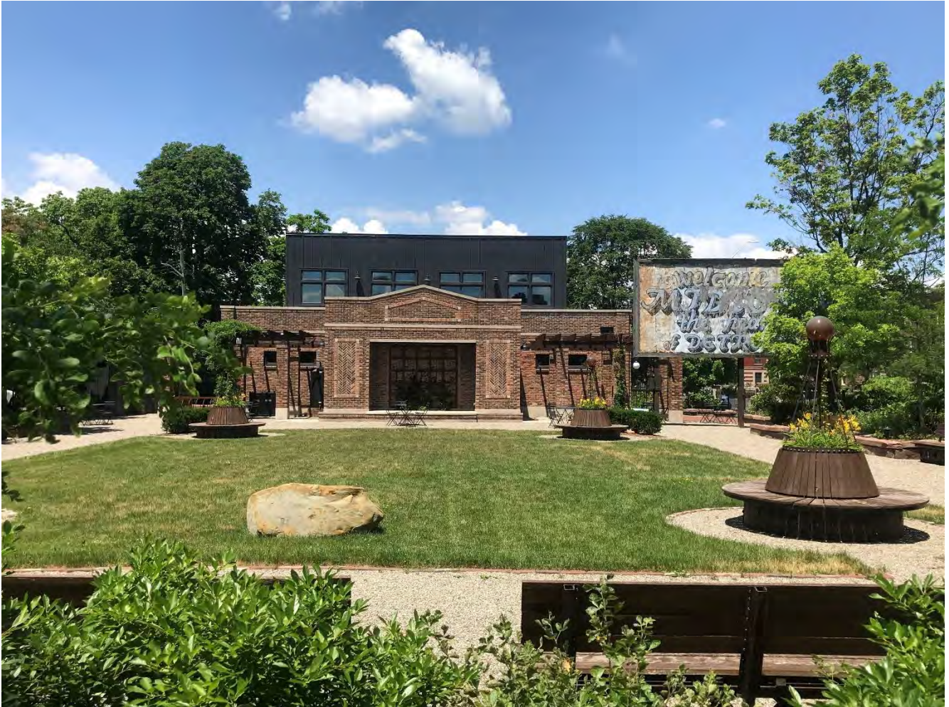
“Rear” Elevation and view of gardens, from W. Alexandrine, Staff Photo
