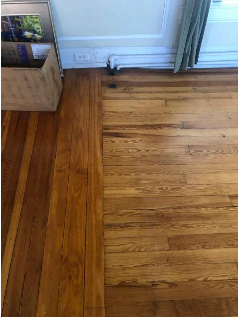
2ND FLOOR PITCH DUE TO SETTLING
