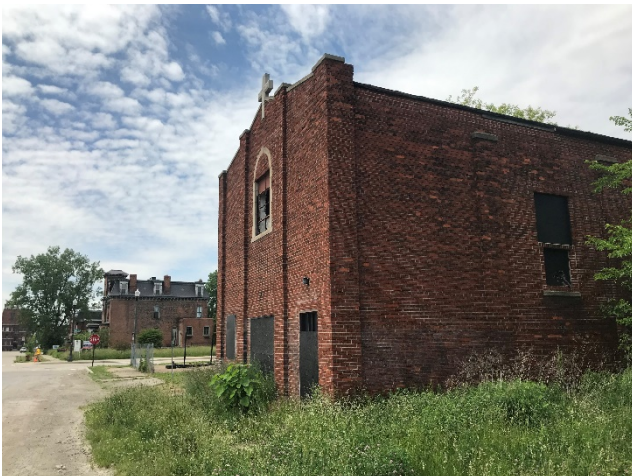
South-West View, staff photo, 6/4/2020
