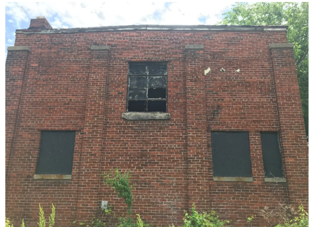
North Elevation, staff photo, 6/4/2020
