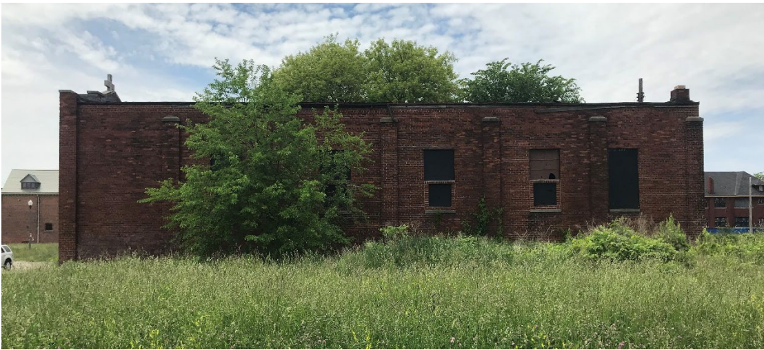
East Elevation, staff photo, 6/4/2020
