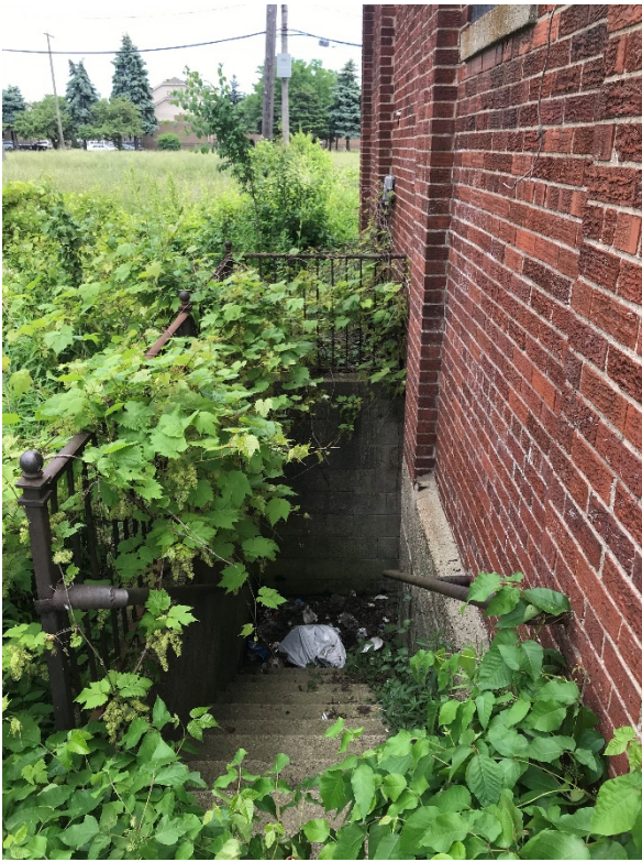
Rear staircase to basement door, staff photo, 6/4/2020
