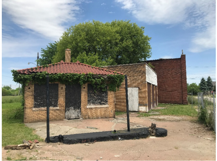
Adjacent vacant structures on Watson, staff photo, 6/4/2020
