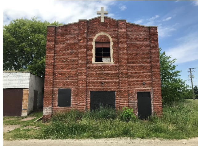
South Elevation, staff photo, 6/4/2020
