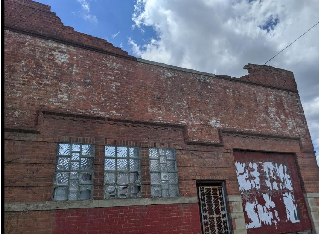
Carriage house, east elevation
