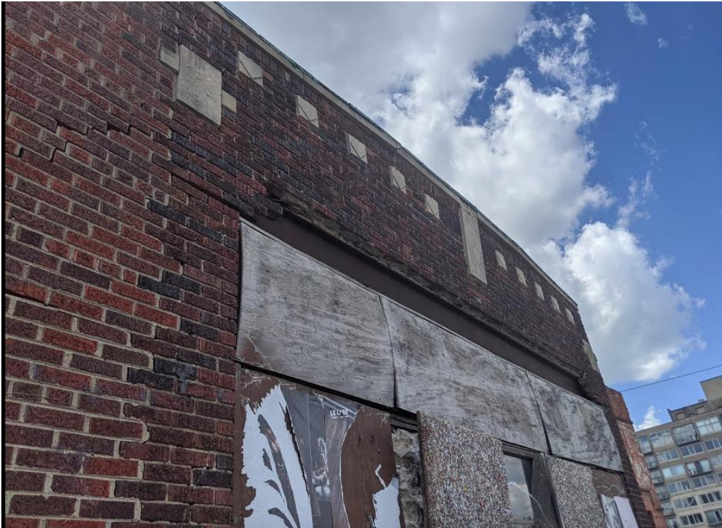
2827 John R, ca. 1952 storefront addition proposed for demolition
