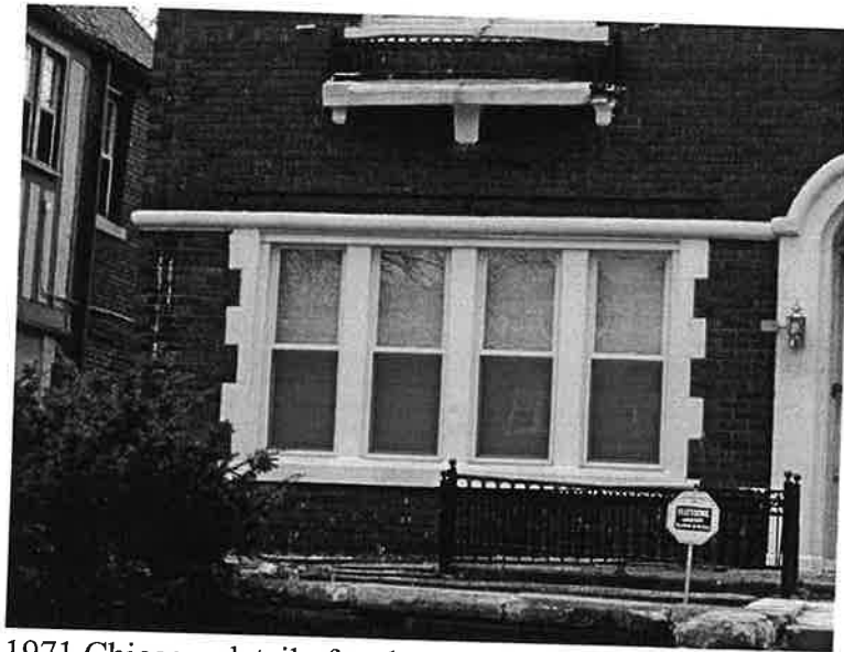
1971 Chicago, detail of replacement windows
