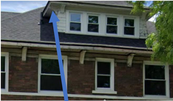
All dormer soffits will be replaced as needed with 1408 beaded ceiling as referenced in the photo below. **Paint color will match C4 from color pallet C.**
