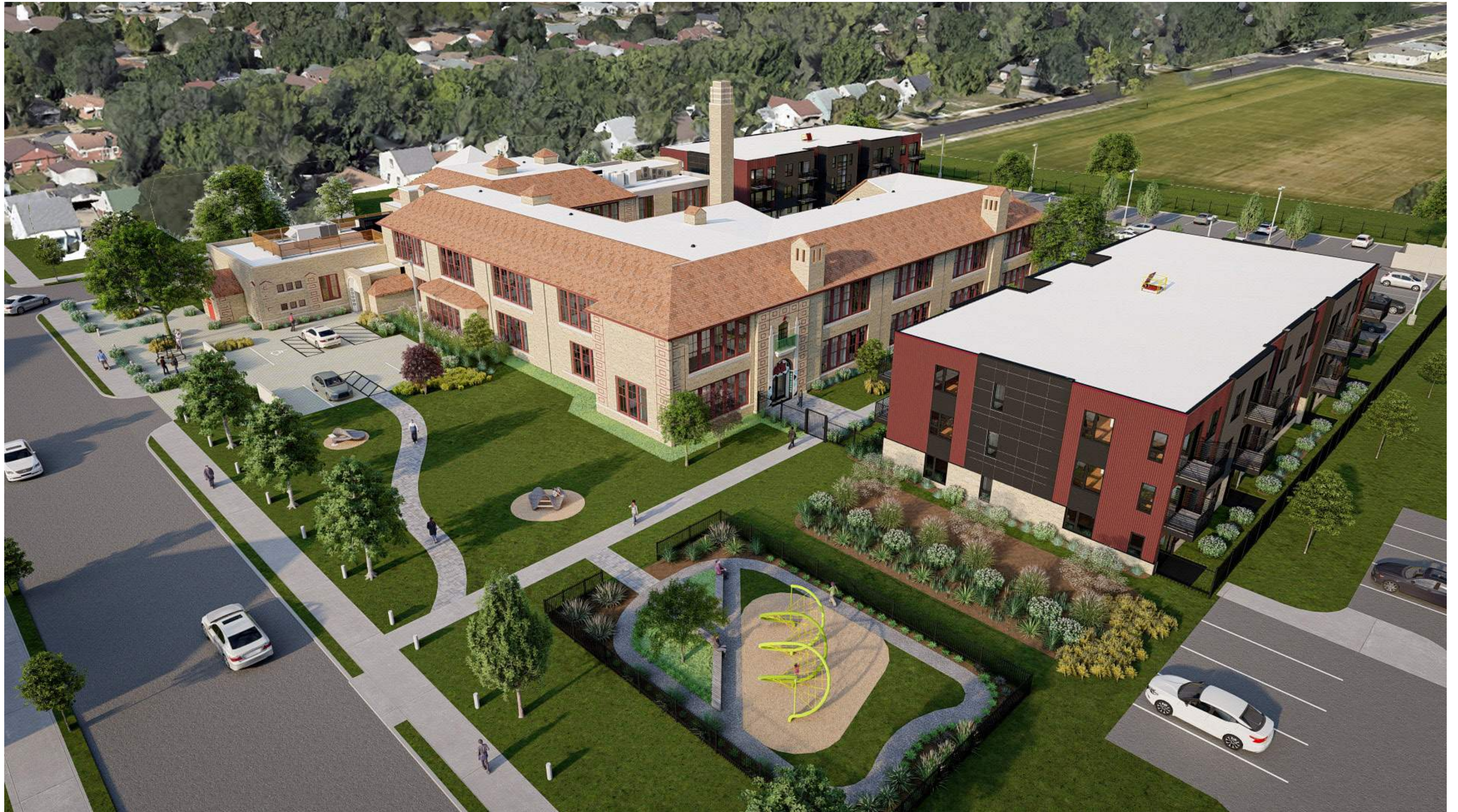
Aerial view looking Northwest
