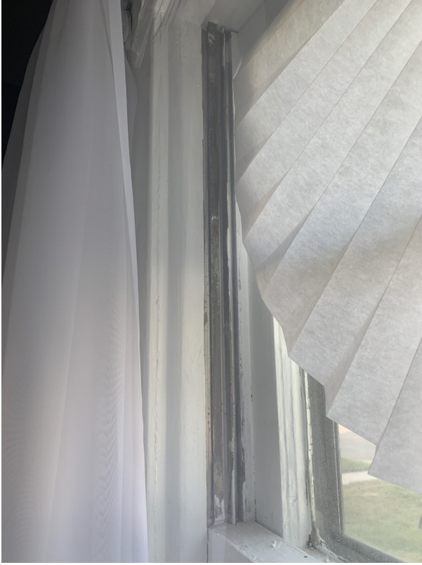
Reel spring window balancer
