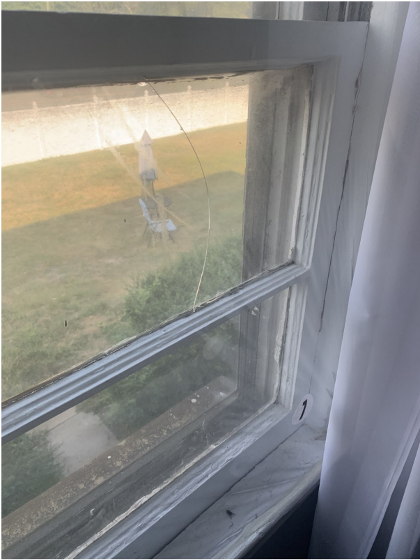
Interior view. Reel spring sash balance.
