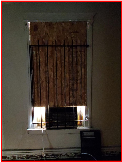
Existing Bedroom window
