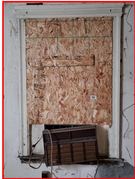
Existing Family Room window
