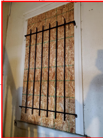
Existing Stair window
