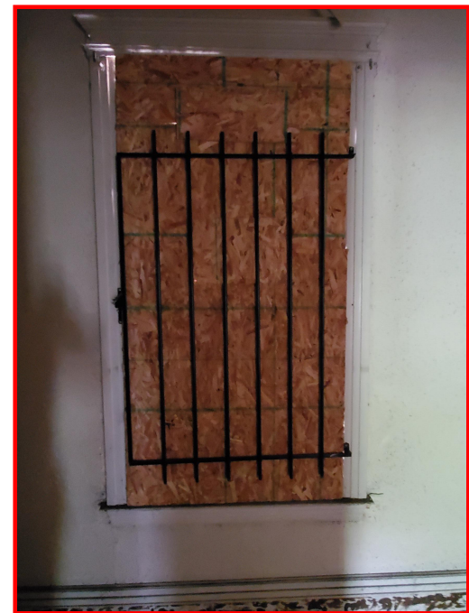
Existing Bedroom window
