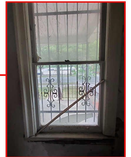
Existing Dining Room window
