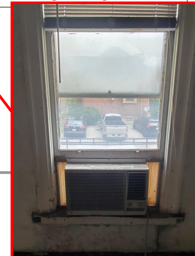
Existing Dining Room window
