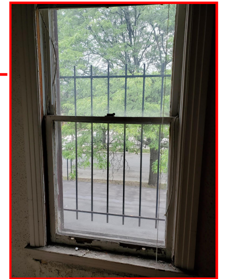
Existing Bathroom window
