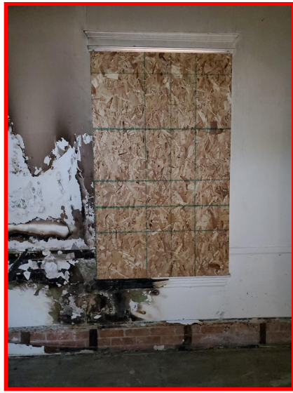
Existing Kitchen window
