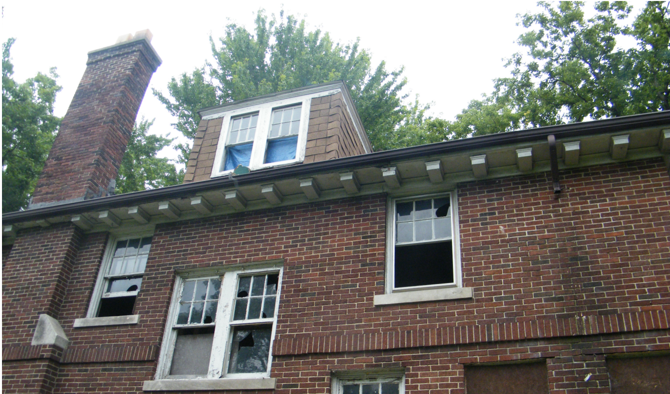
Exhibit Three: Dormer with Asphalt Shingle, 2013
