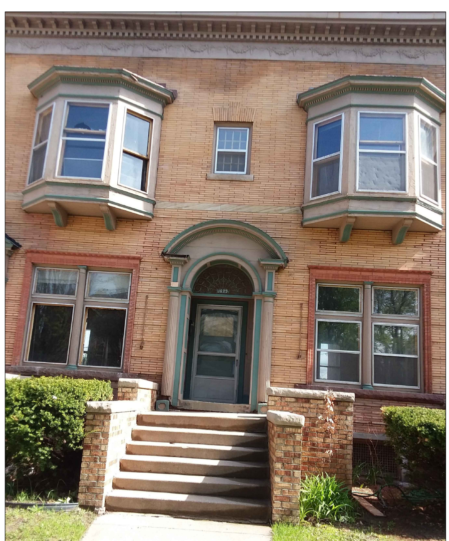
Building Before Renovations Front Entry Porch (Typical)
