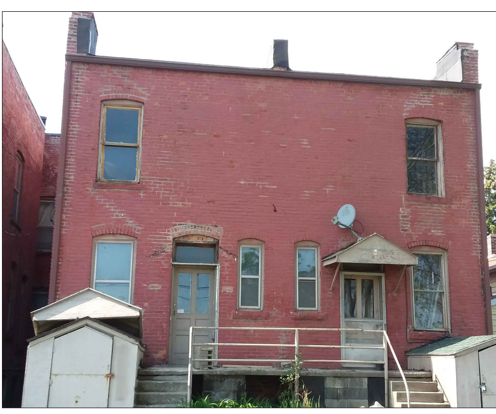
Building Before Renovations South Wall - Units 1 and 2
