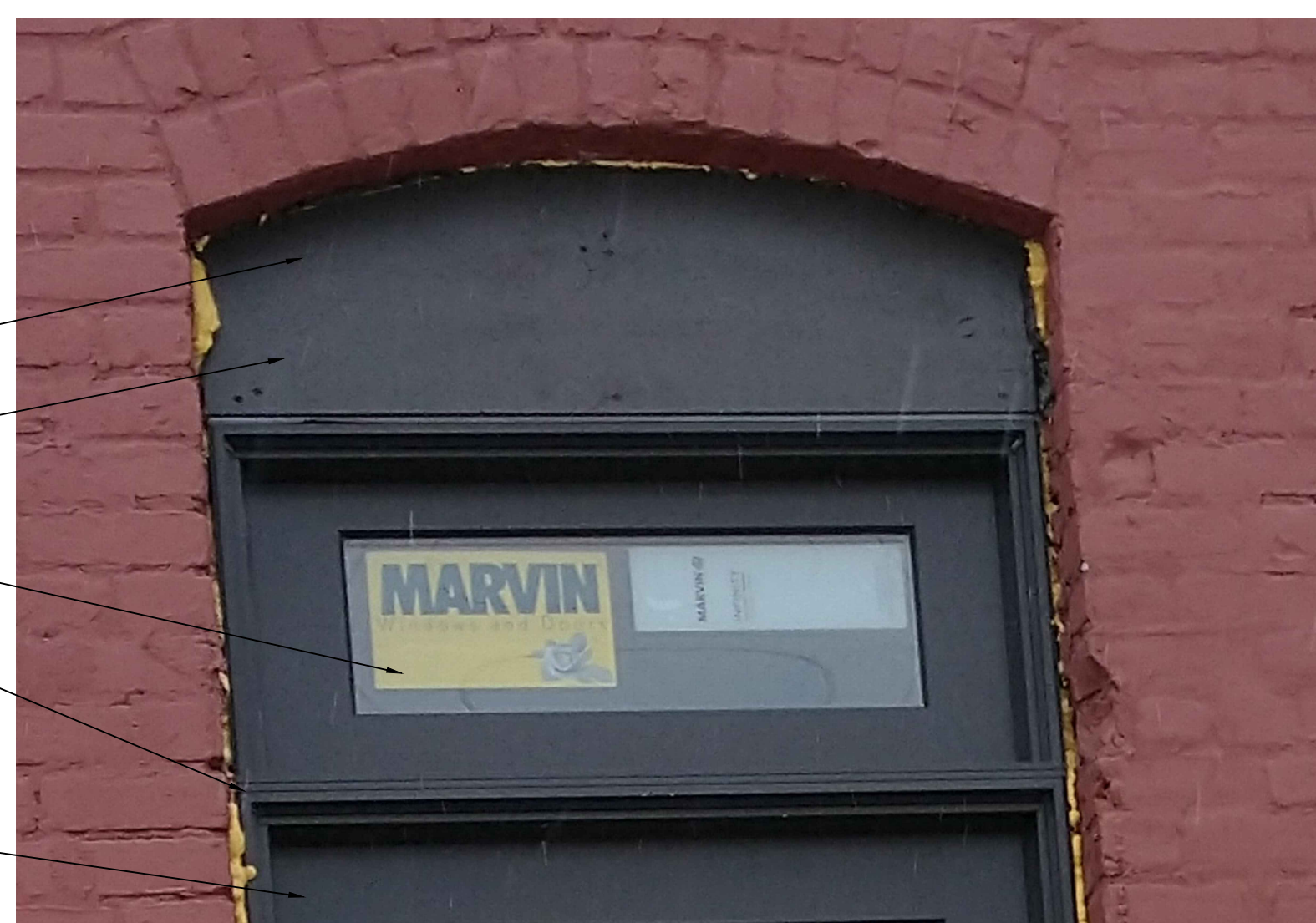
Enlarged View of New Door Transom Opening
