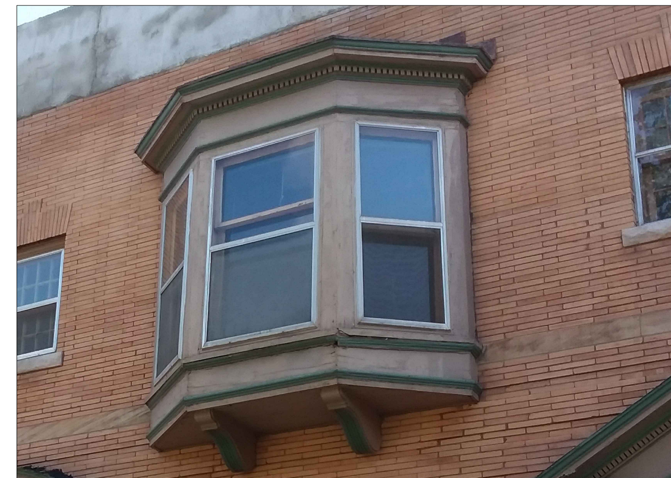
Bay Window Before Replacement
