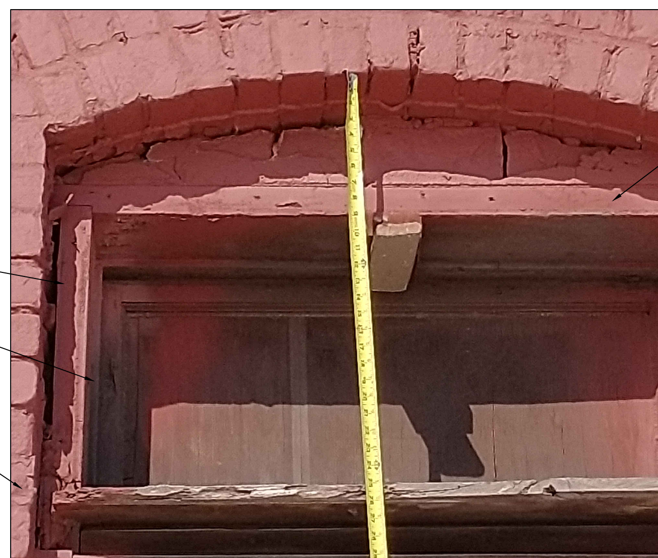
Enlarged View of Existing Door Transom Opening
