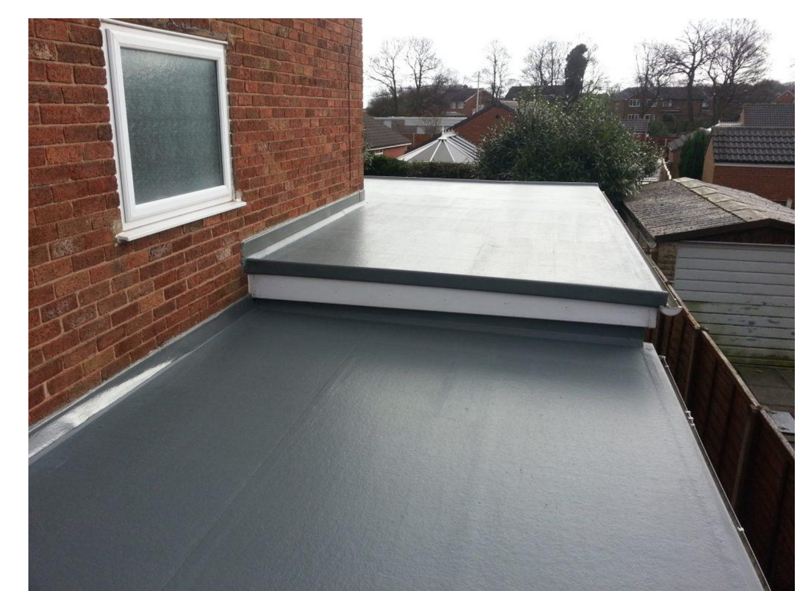
TYPICAL EPDM ROOF SIMILAR TO THAT PROPOSED FOR THIS PROJECT
