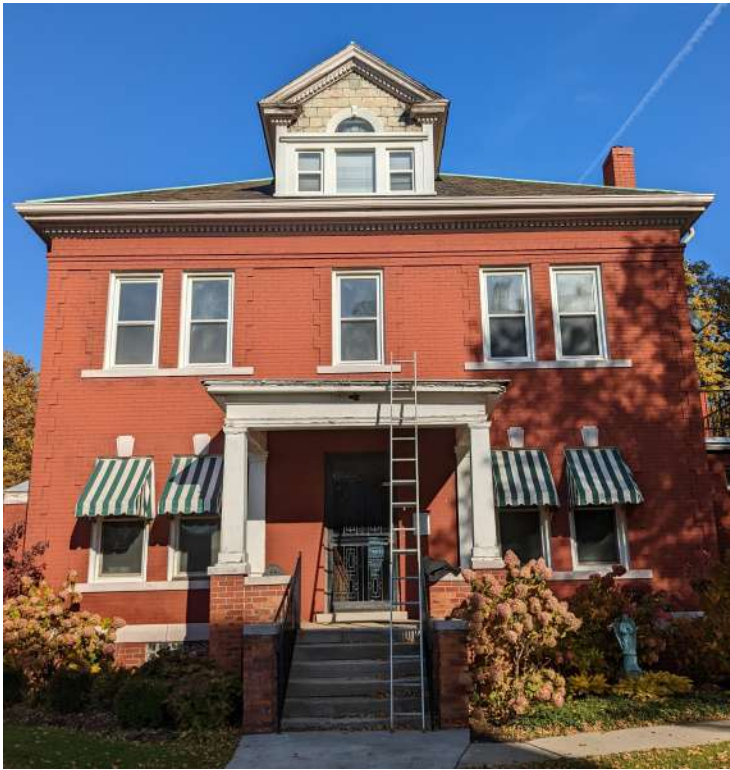
OVERALL EXISTING CONDITION
