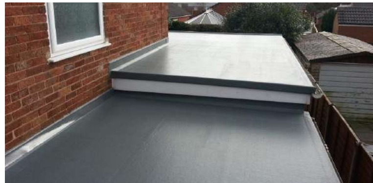
TYPICAL EPDM ROOF SIMILAR TO THAT PROPOSED FOR THIS PROJECT
