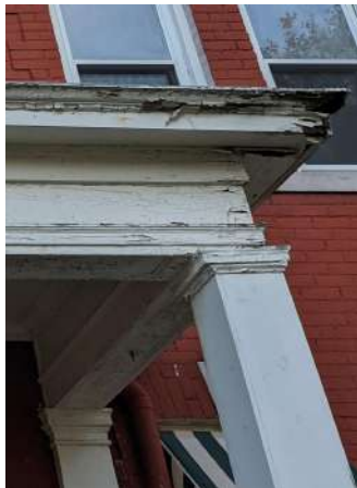
TEMPORARY COLUMNS COLUMN/PILASTER OFFSET, EXPOSED COLUMN CAPITALS
