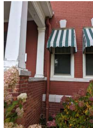
EXISTING PILASTER EXISTING DOWNSPOUT
