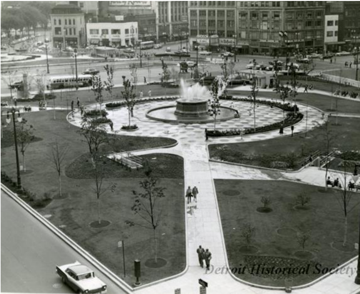
Looking southeast after reconstruction, 1959
