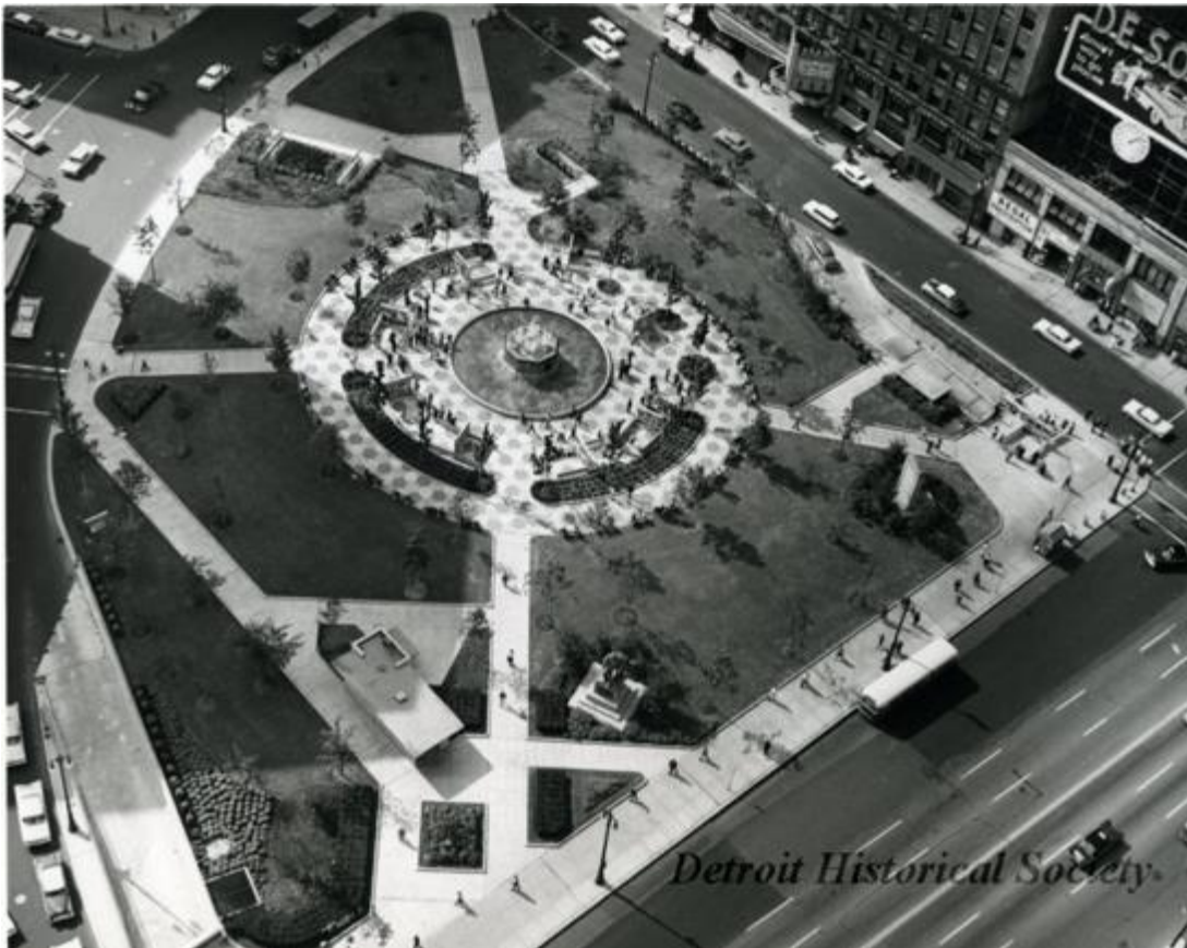
West half of the park after reconstruction, 1959
