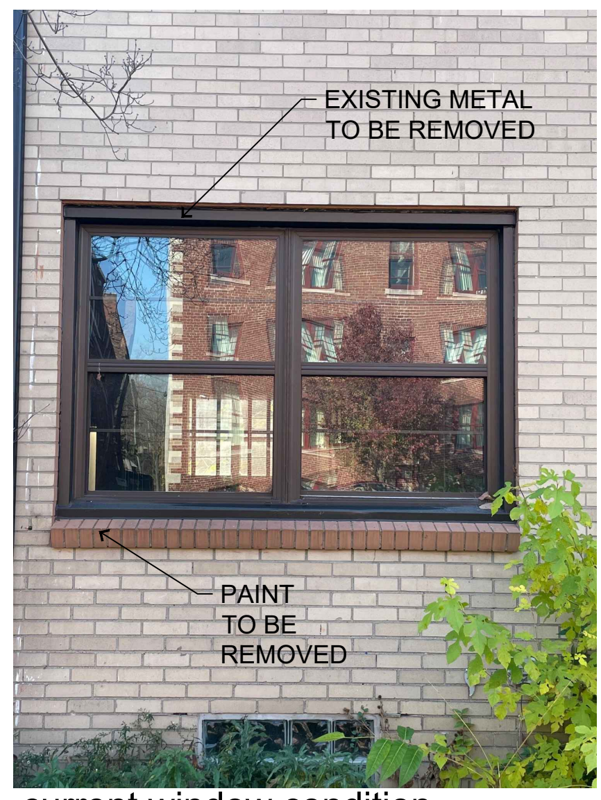
current window condition (typical for 160 windows)
