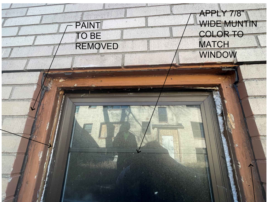
window with metal removed (top head view)
