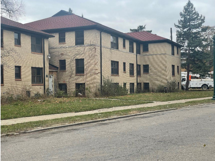
Photo 3: View looking southwest from Whitmore
