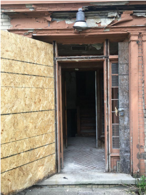
Door 2 – Existing prior to securing.
