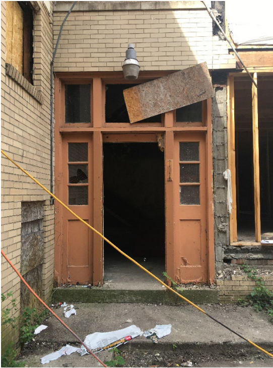
Door 4 – Existing prior to securing.
