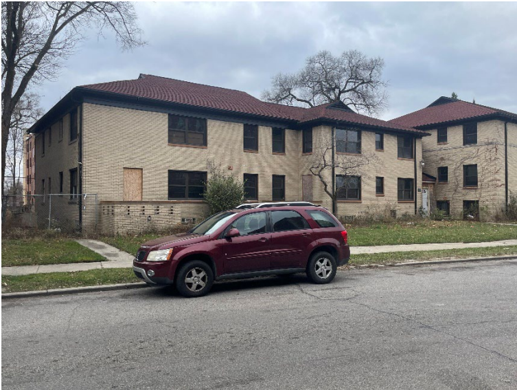
Photo 4: View looking southwest from Whitmore
