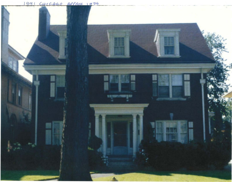
North/Front Elevation (BEFORE) 1974
