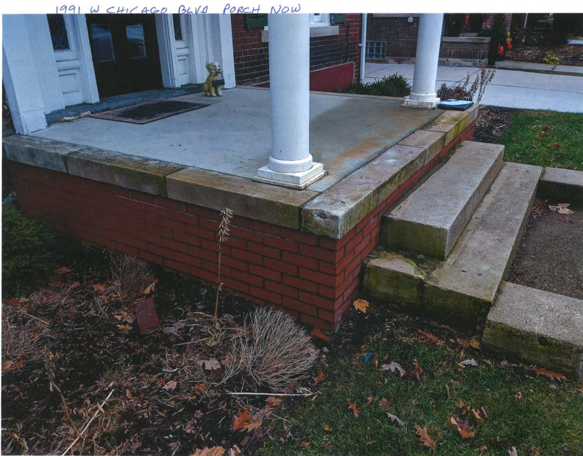
Front Porch Detail (AFTER) 2020
