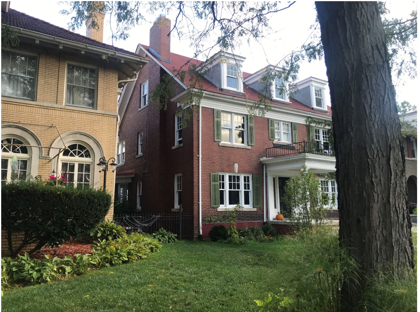
Northeast/ Front-Left Elevation
