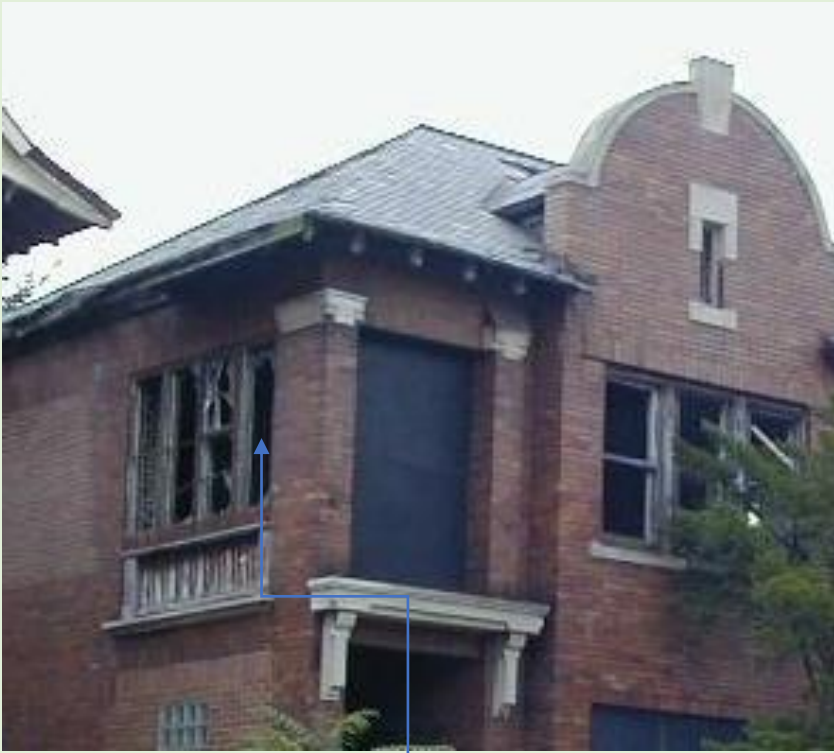
Condition in 2000. Note that this location included 4, 1/1, double-hung, mullied windows within this opening.
