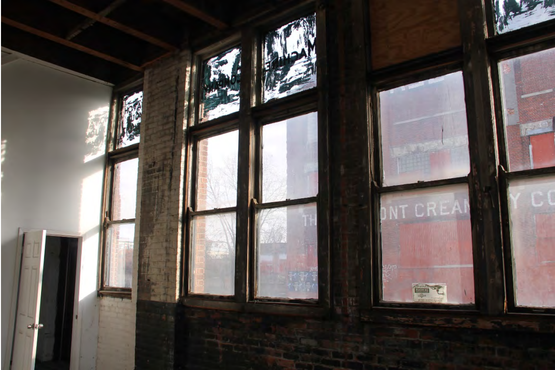
Interior View of Wood Double Hungs
