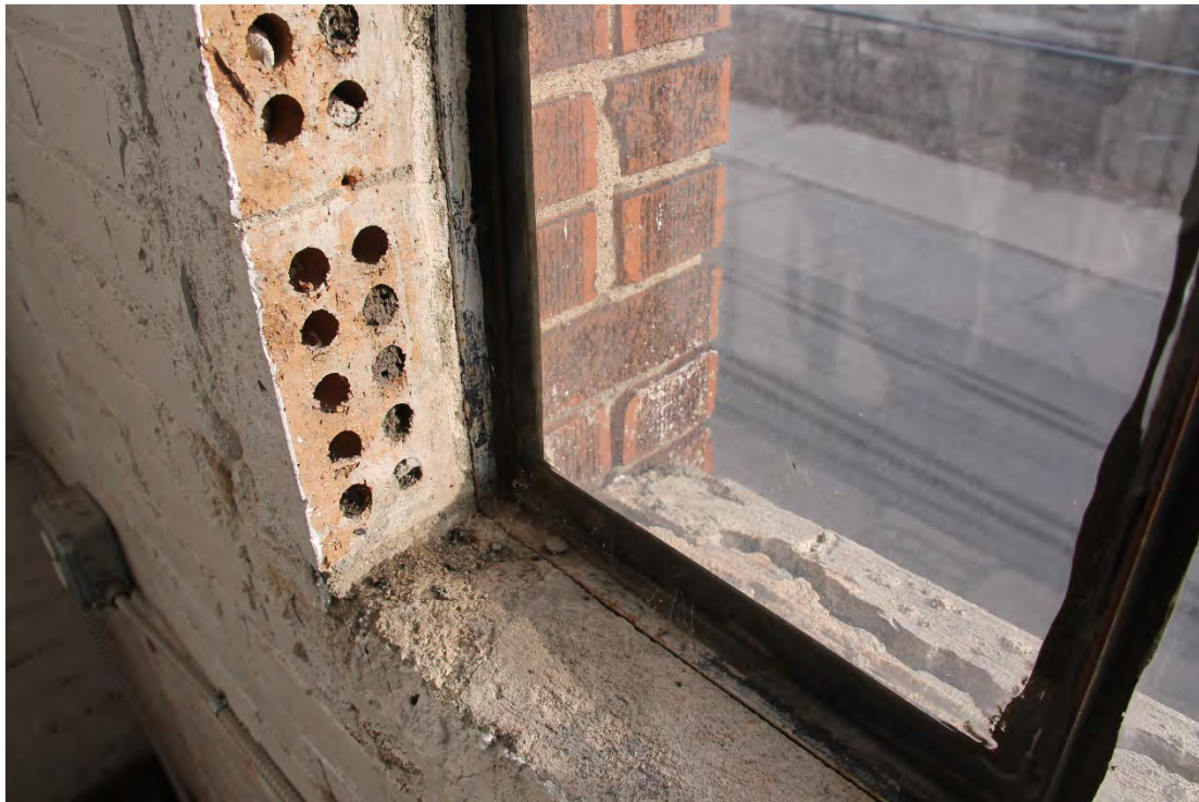
Interior View of Replica Steel Window, Shows Altered Masonry Opening Changing Window Size
