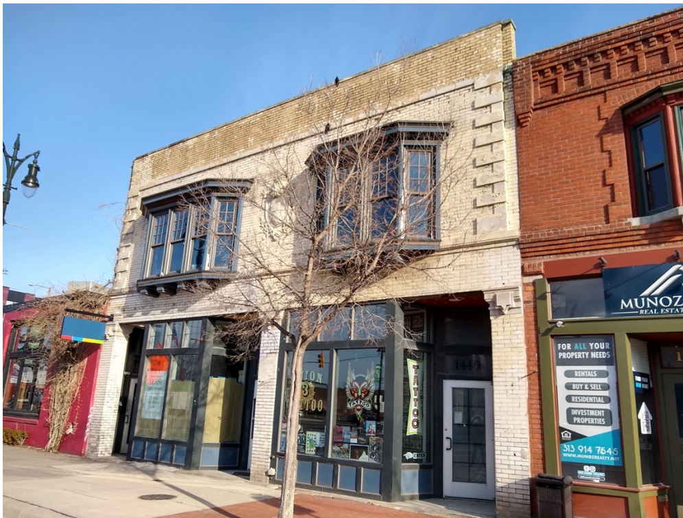
Michigan Ave Facade
