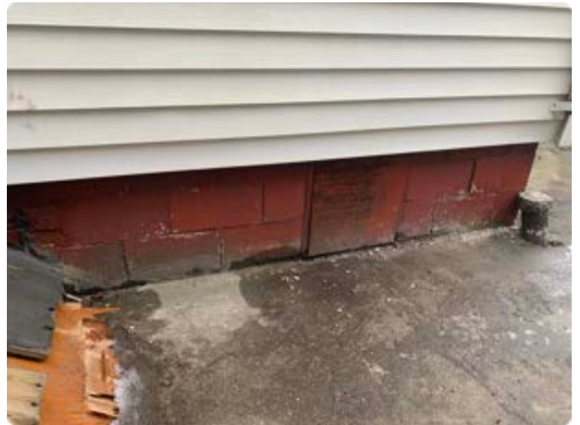
Current Rear addition foundation
