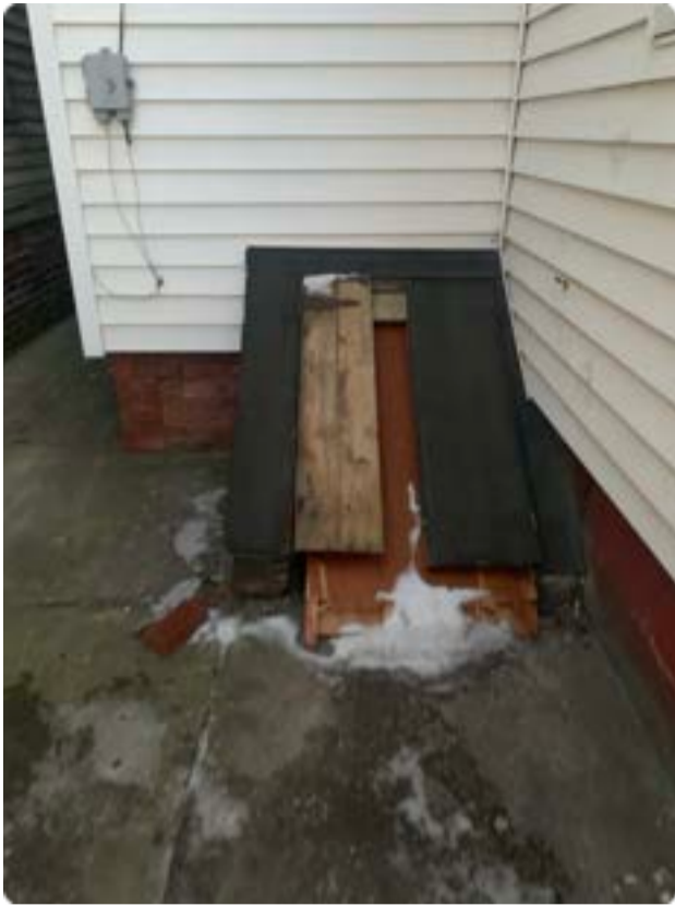
Exterior basement access
