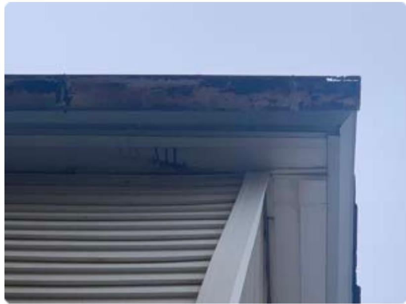
Rotted gutter
