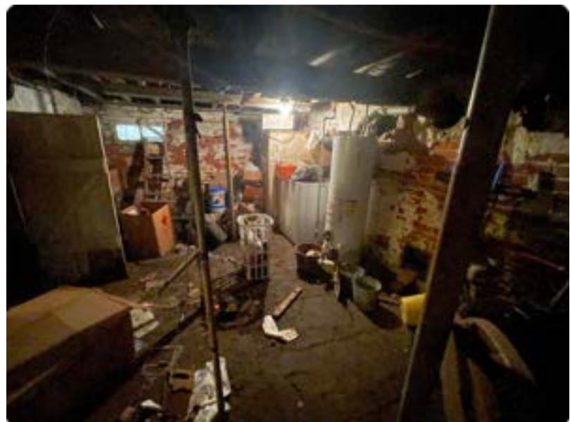
Basement floor from bulkhead door
