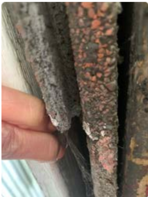
Layers of covering under vinyl siding rear left corner
