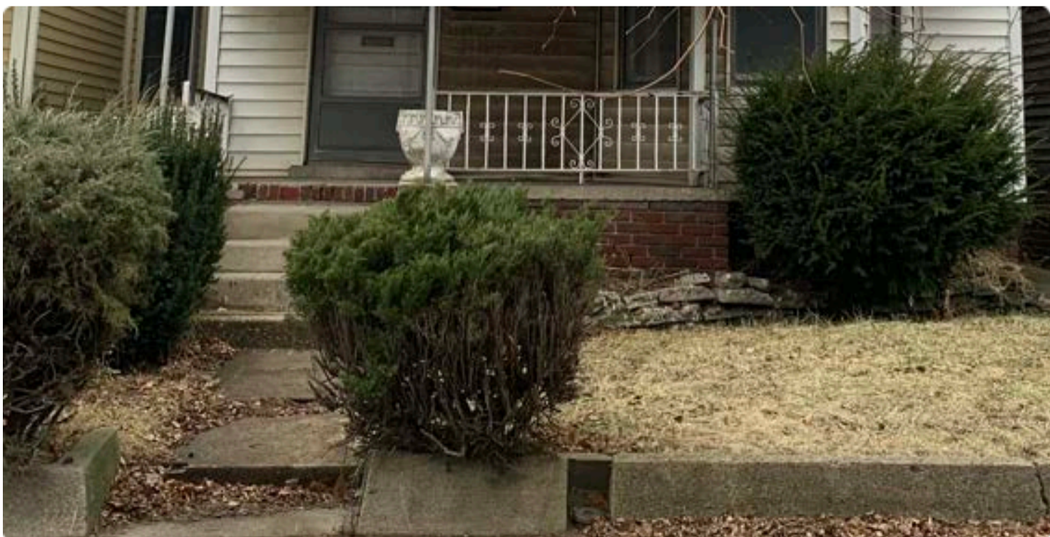
Front of Home Overgrown Landscaping
