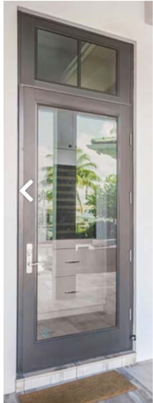
Upstairs bedroom balcony exterior door
