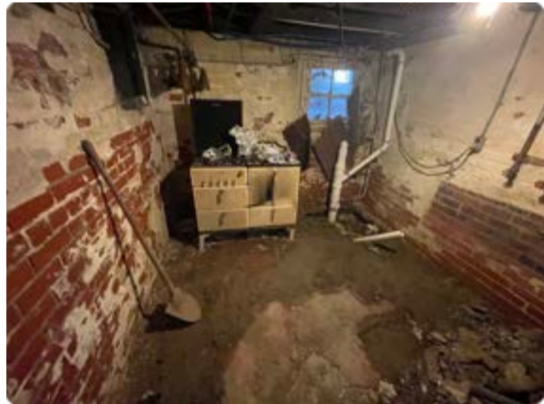
Basement floor from bulkhead door
