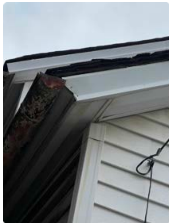
Three visible layers of roof
