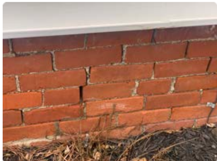
Left side brick foundation
