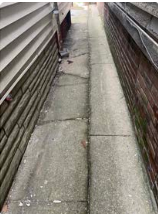
Right side stone overlay foundation
