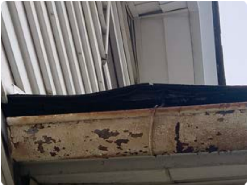
Rotted Gutter
