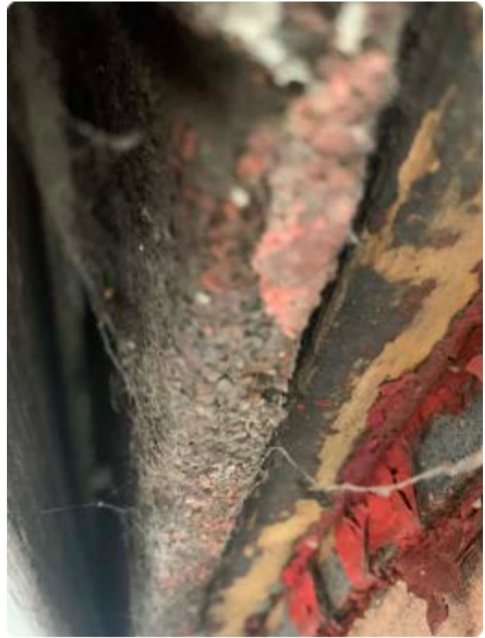
Layers of covering under vinyl siding
