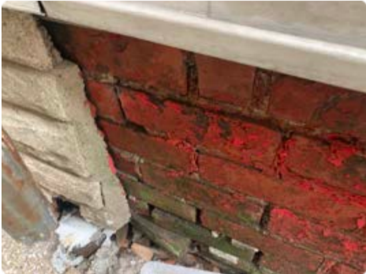
Right side brick foundation
