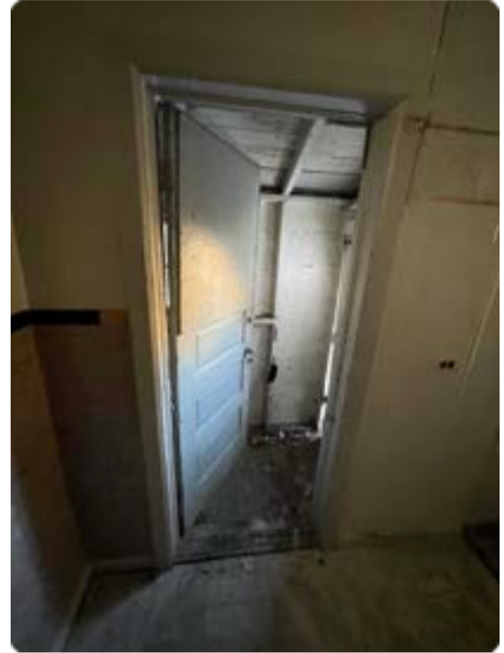
Back porch interior door
