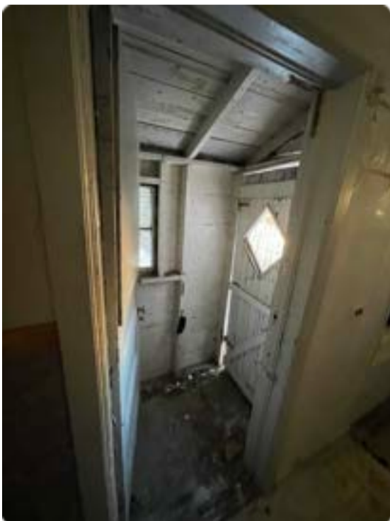
Back porch exterior door
