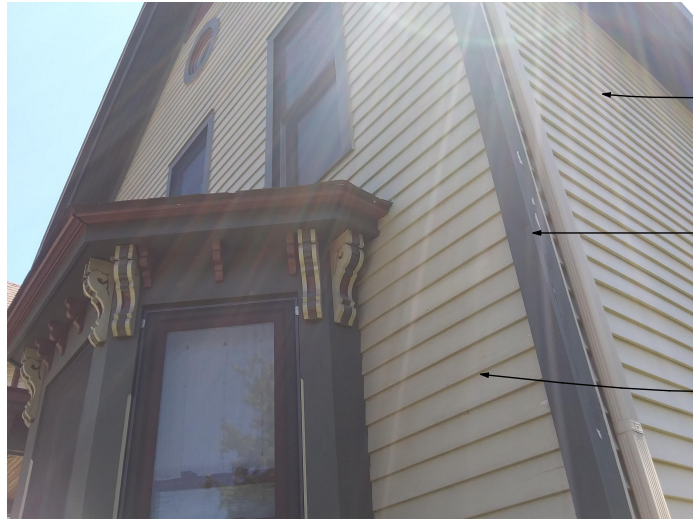
Northwest house corner showing wood siding and italianate detailing on north elevation, wood corner trim with peeling paint and west vinyl-sided elevation. All wood trim to remain in place and be repainted. All vinyl siding to be removed and replaced with cedar bevel siding to match north elevation.
