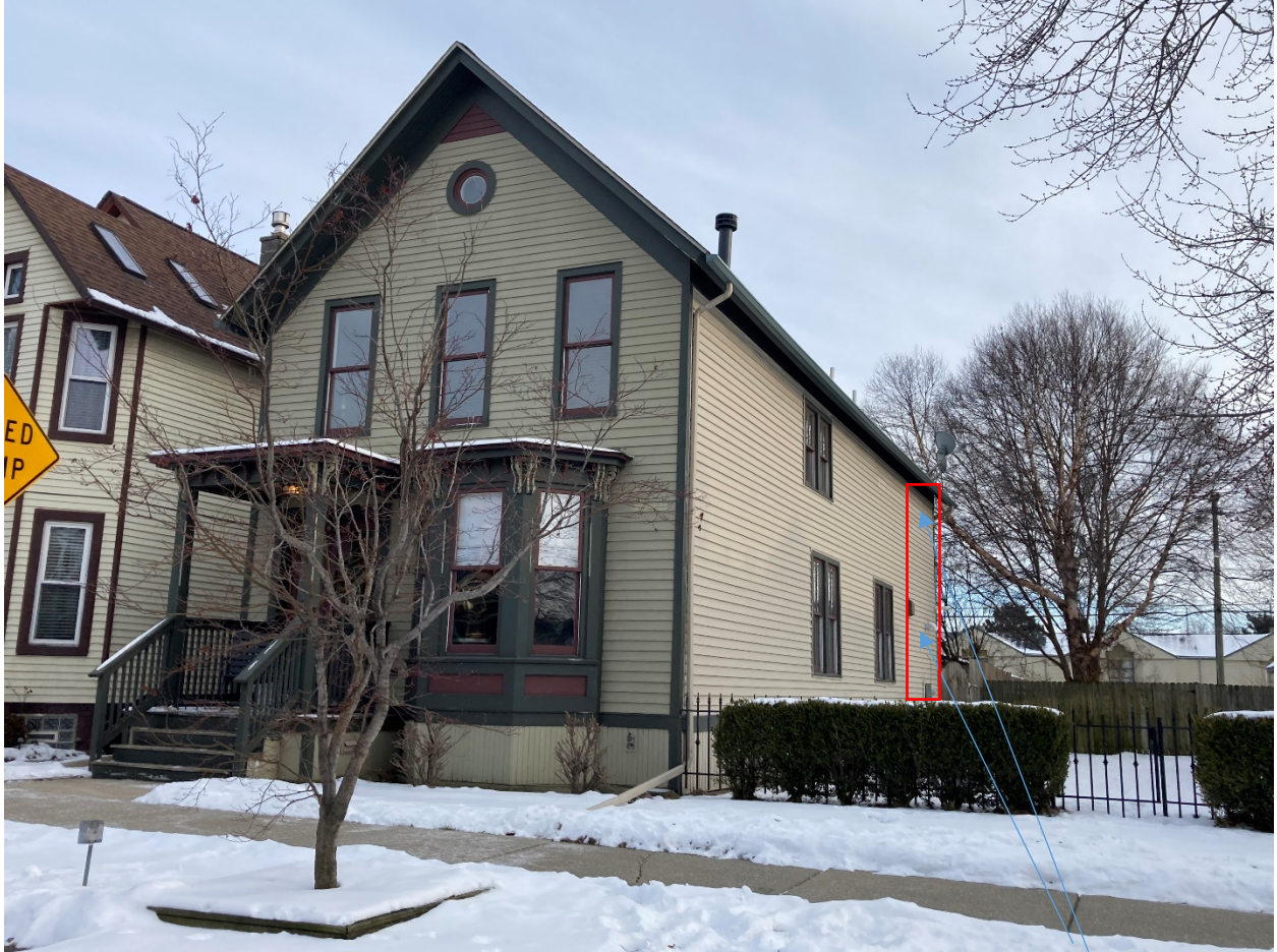
1535 Leverette, current appearance, New vinyl-clad windows to be installed at these locations. Area outlined in red shows location of 1985 addition
