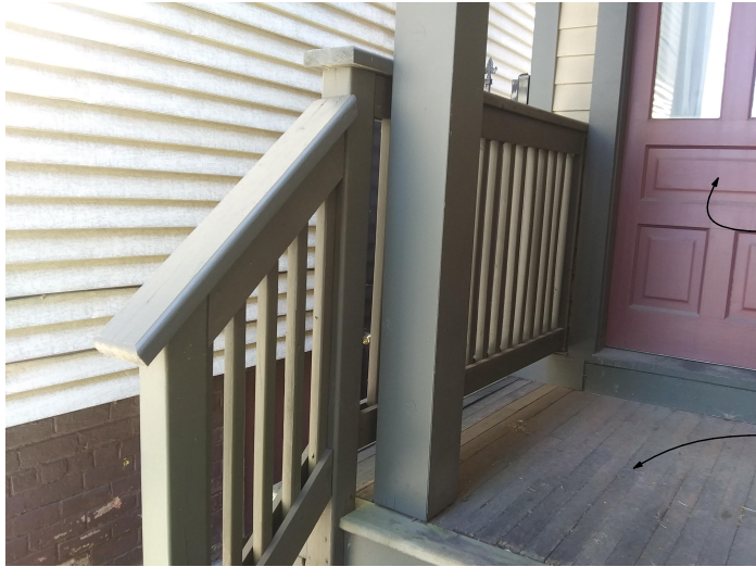
North (Front)-Facing, East Side Porch: Existing wood floor requires minor repairs, sanding and clear waterproof coating.
