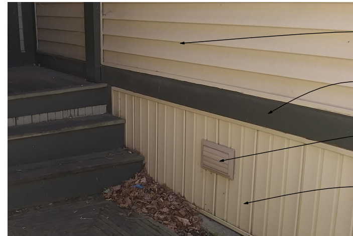
East Elevation: Remove all horizontal and vertical vinyl siding. Replace horizontal siding with new beveled cedar siding to match existing north elevation siding exposure. Replace vertical vinyl siding with new cedar vee siding to match crawlspace cladding at north elevation. Any existing wood siding discovered upon removal of vinyl siding will be repaired if possible. Replace vinyl crawlspace vents with new metal vents painted to match crawlspace vertical siding. See materials.
