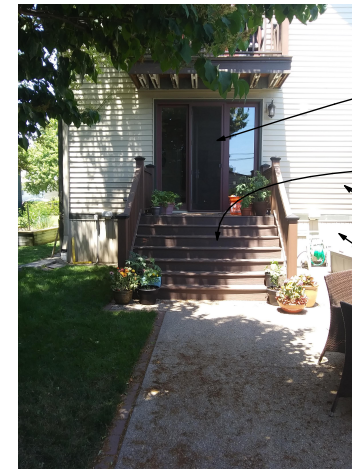
South Elevation: Rear porch to be removed. The relatively new rear porch and railing systems are clad with plastic composite lumber. All horizontal and vertical (crawl space) vinyl siding to be removed and replaced with cedar bevel and vee siding respectively to match existing materials at the north (front) elevation.
