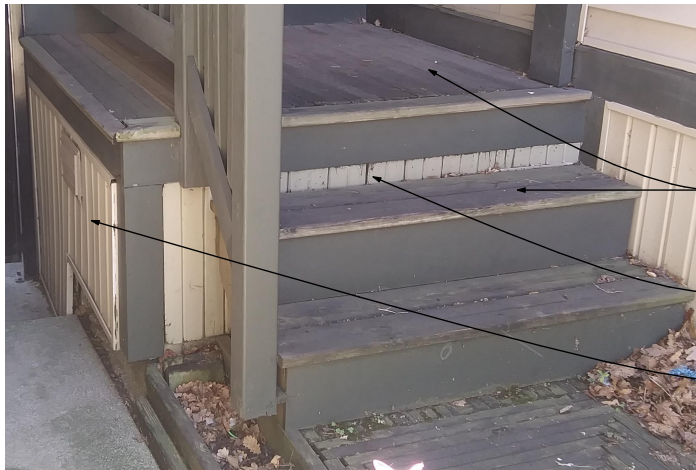
North (Front)-Facing, East Side Porch: Existing north vee siding to be repaired. East vinyl cladding to be replaced with new cedar vee siding. Step risers to be repainted, step treads to receive new clear waterproof finish.
