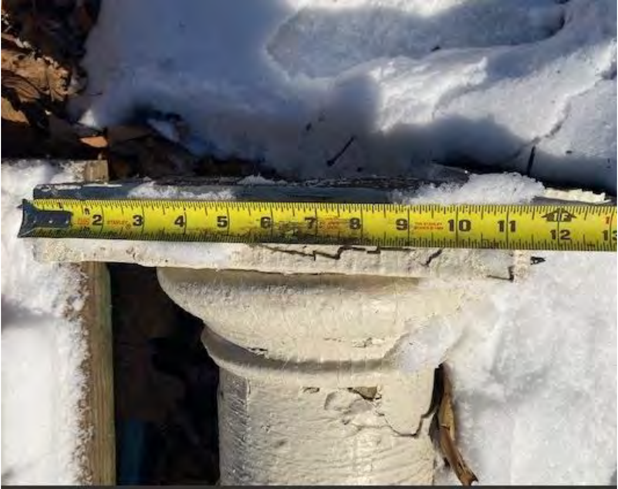
Width of the abacus (the flat slab forming the uppermost member of the capital of the column).
