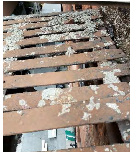
Figure 5: Warped Metal Slats
