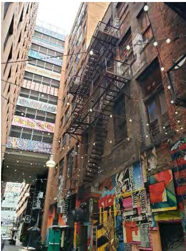
Figure 1: 1315 Broadway Fire Escape
