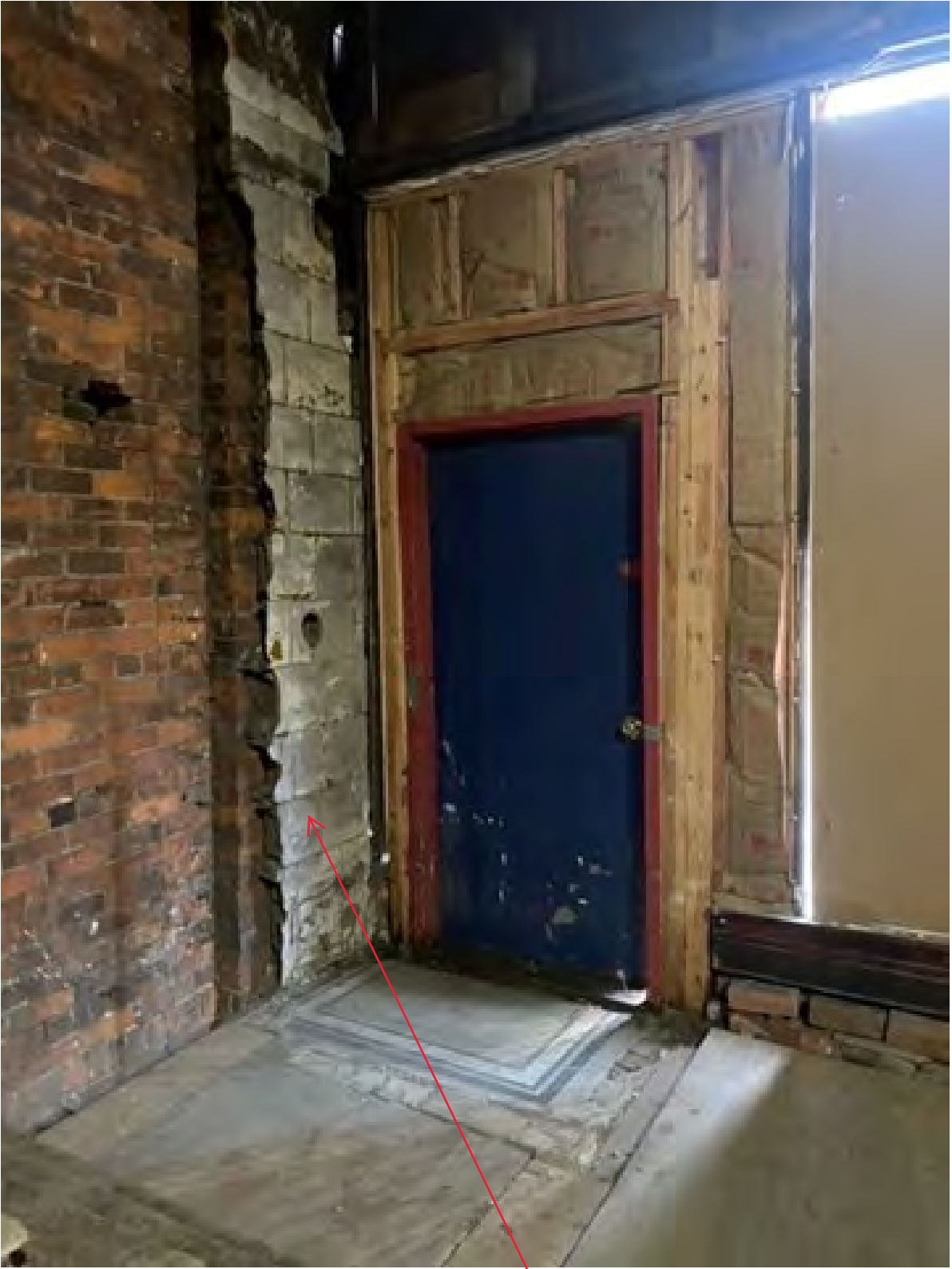
REPAIR/RESTORE SIDE WALL.
