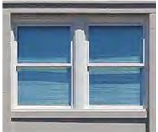
Exterior view, Thermal Windows Series 700 (Palace Apts, Tulsa OK)
