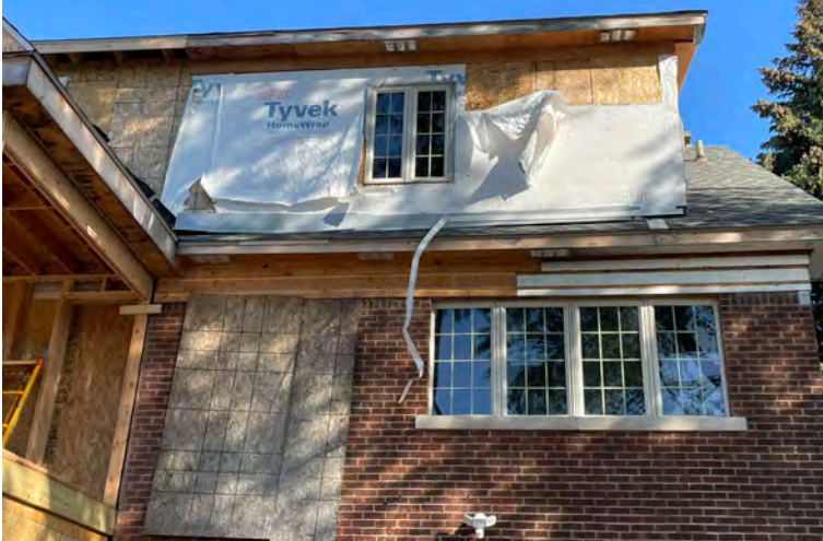
Rear Office Slider Install
