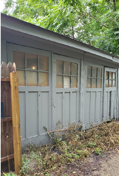
Figure 1: Garage at 864 Longfellow
