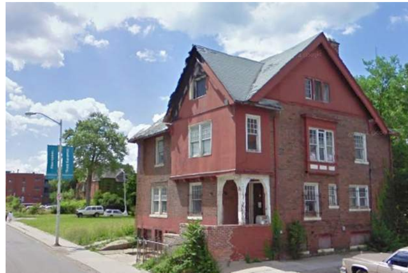
4635 JOHN R ST. - MCCOLLESTER HOUSE VACANT
