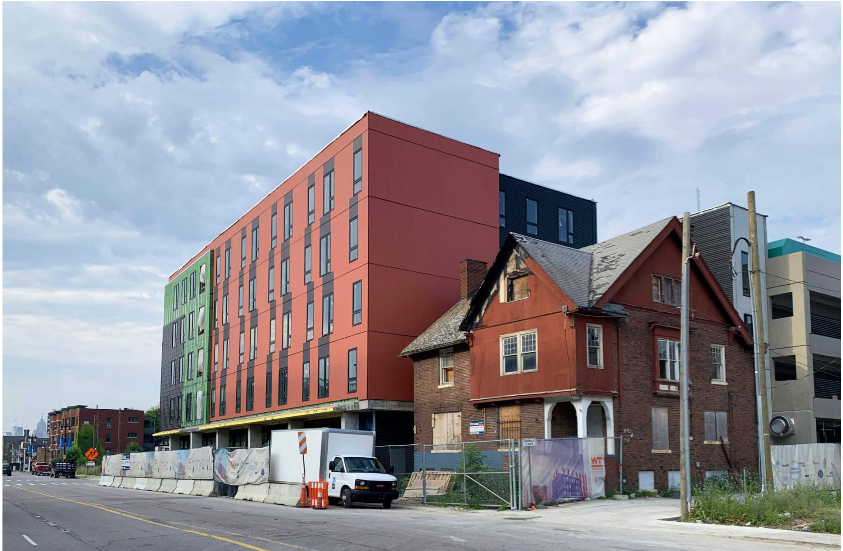
VIEW LOOKING SOUTHWEST ALONG JOHN R
