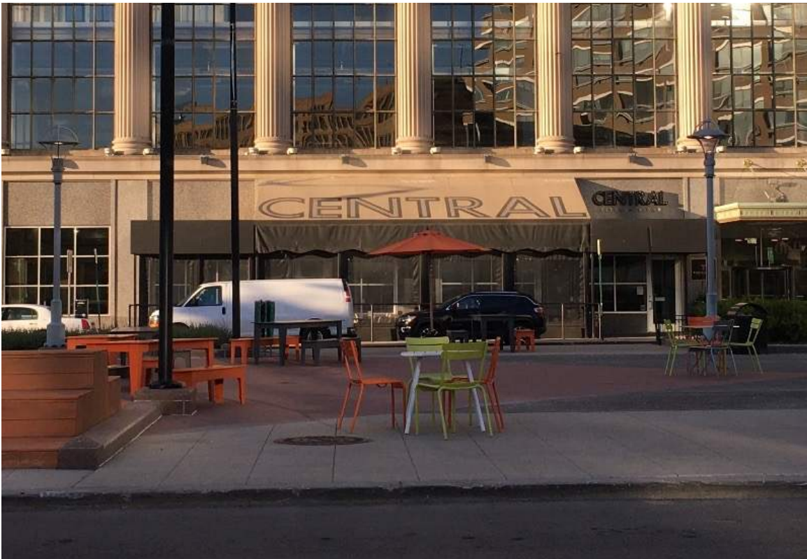
Figure #2: Central Kitchen Awning and Enclosure BEFORE REMOVAL. May 2021
