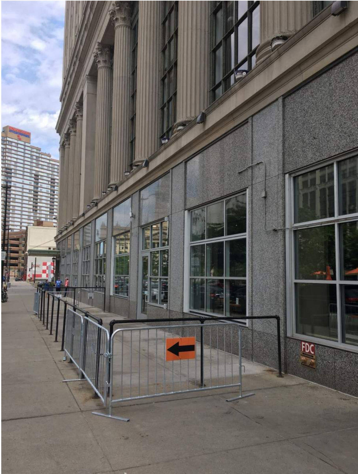
Figure #4: Central Kitchen AFTER REMOVAL. June 2021
