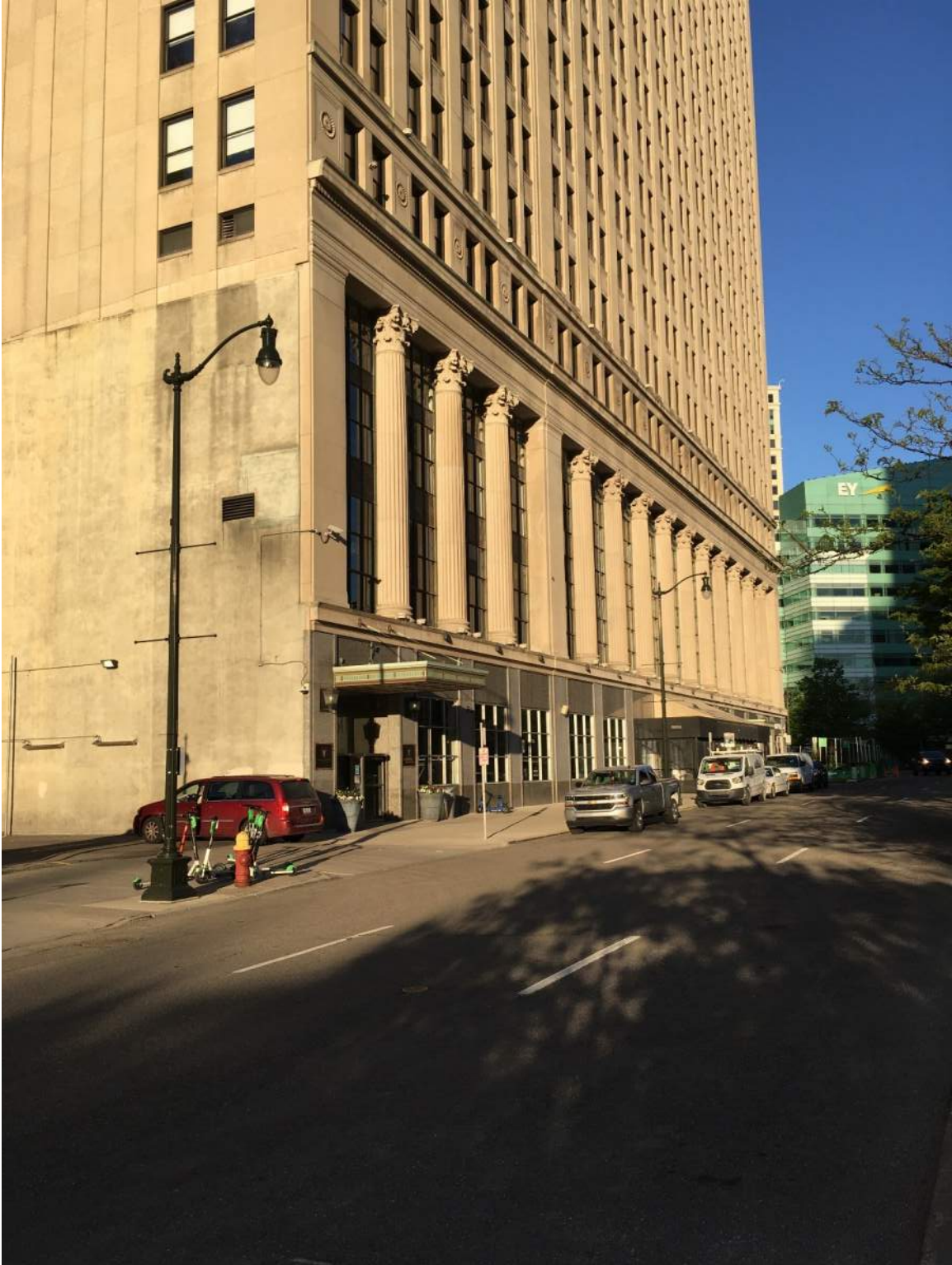
Figure #3: Central Kitchen Awning and Enclosure BEFORE REMOVAL. May 2021
