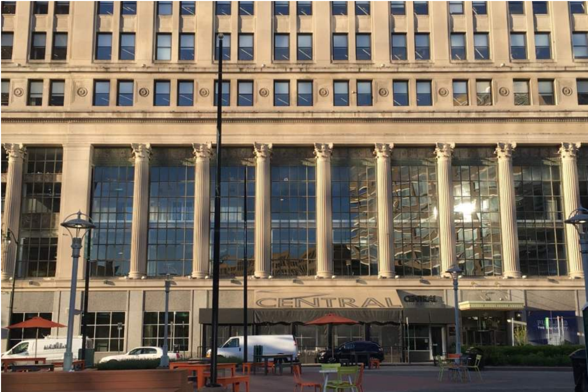
Figure #1: Central Kitchen Awning and Enclosure BEFORE REMOVAL. May 2021
