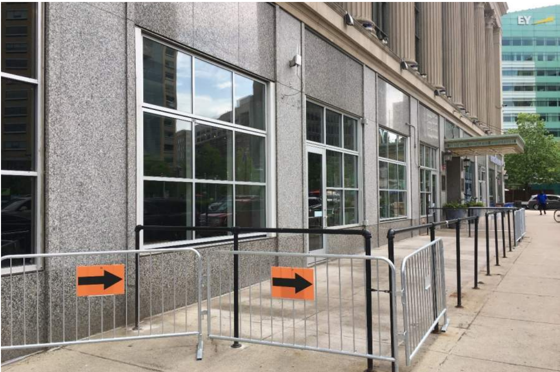
Figure #6: Central Kitchen AFTER REMOVAL. June 2021
