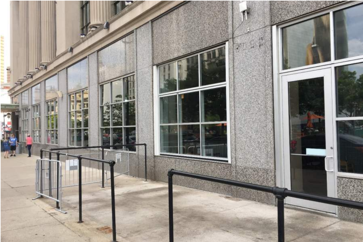
Figure #5: Central Kitchen AFTER REMOVAL. June 2021
