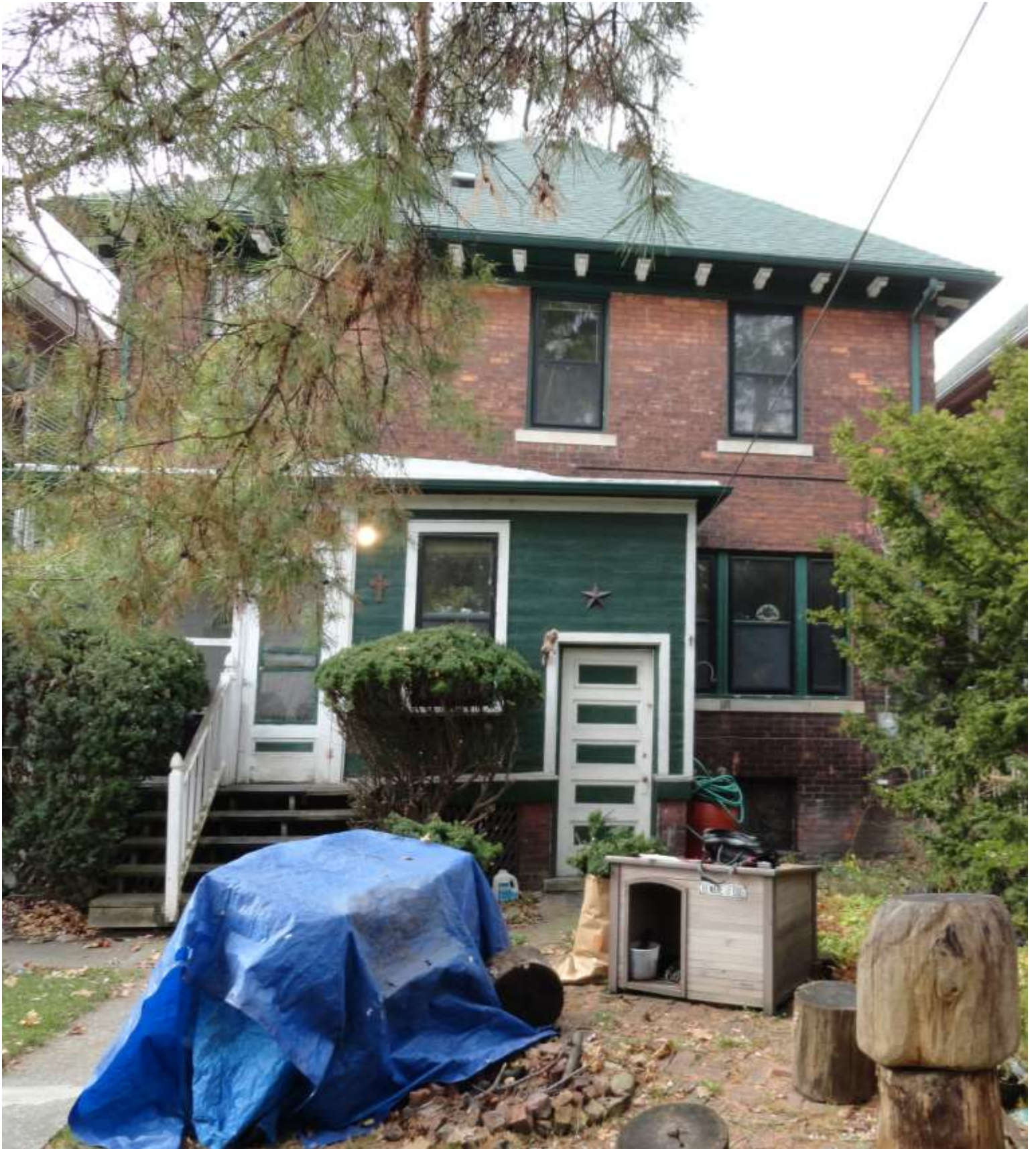
Rear structure to be removed
