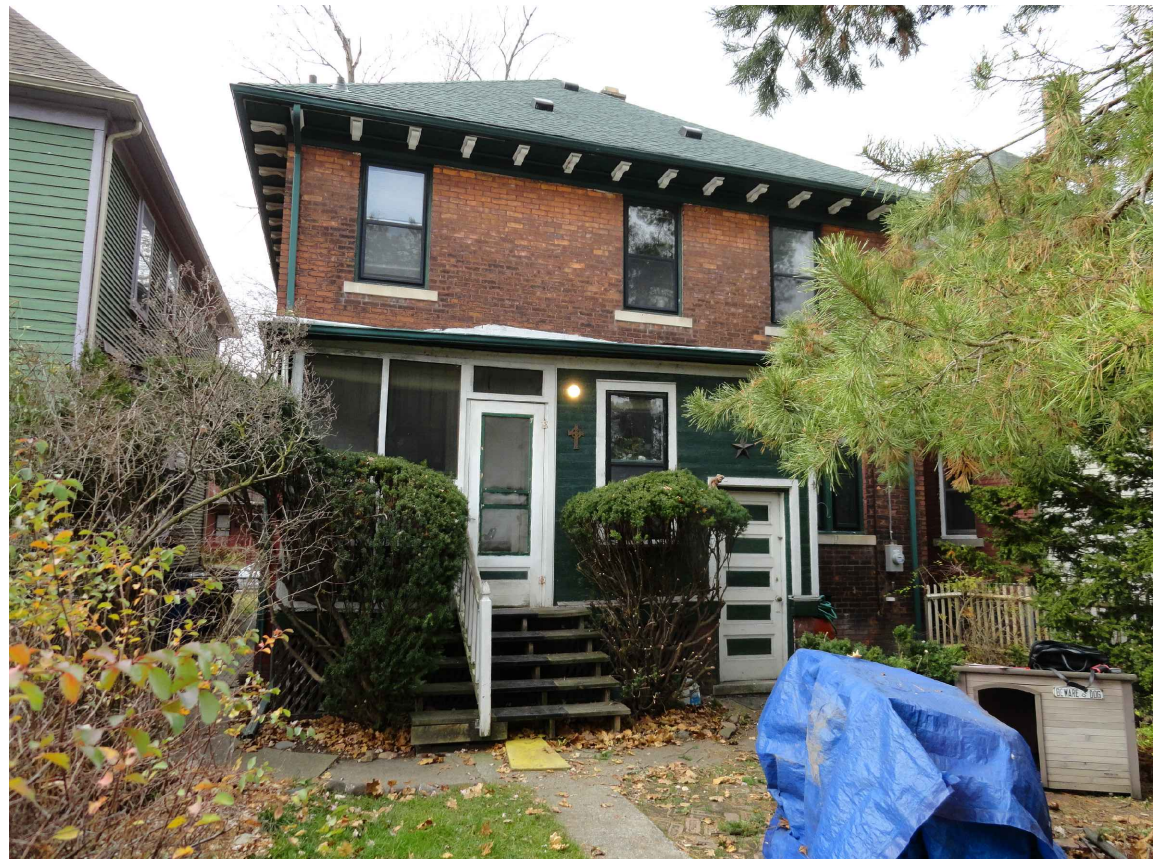
SCREEN PORCH AND BASEMENT ENTRY
