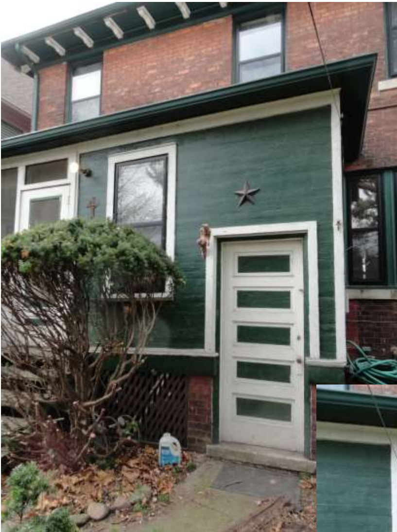
Rear Structure. Door and enclosed stairway to basement to remain
