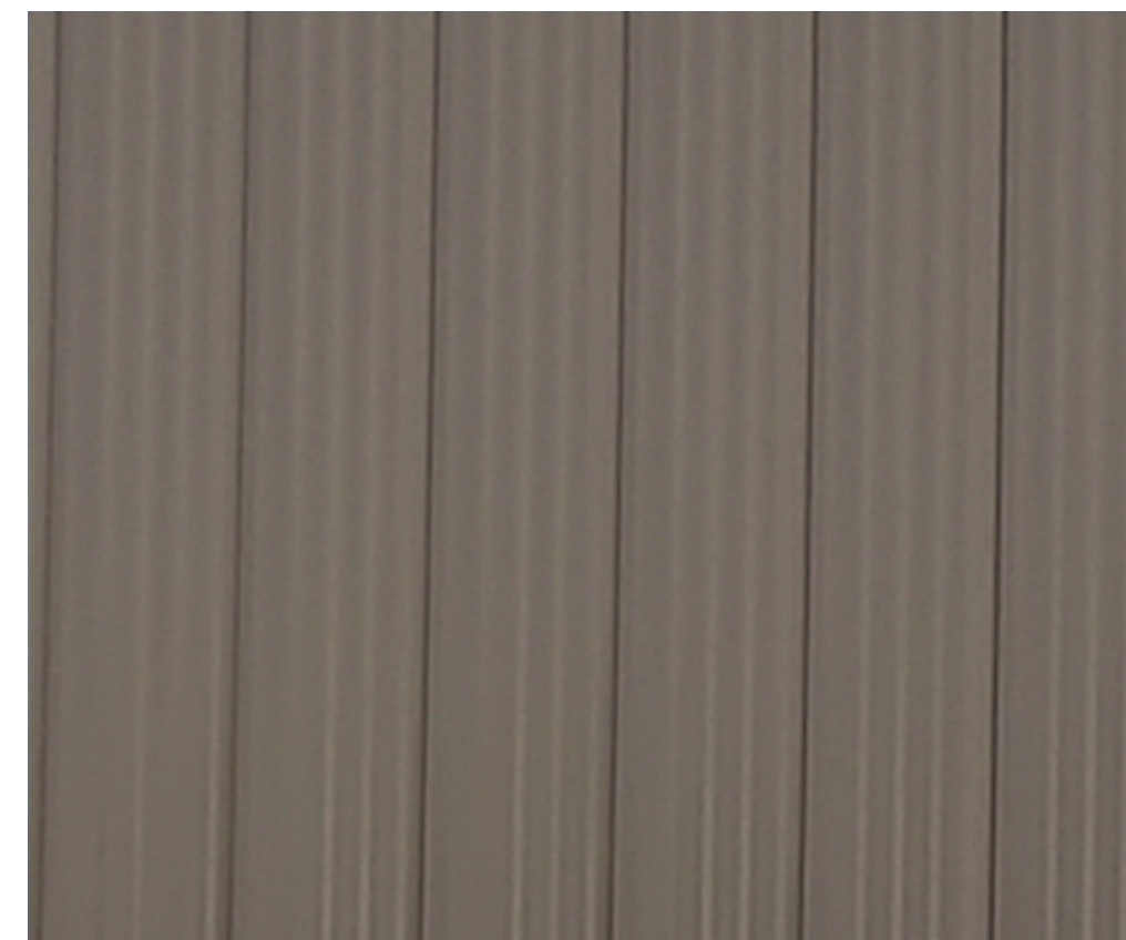
PAC CLAD STANDING SEAM SIDING R-36 PANEL, 24 GA STEEL COLOR: BURNISHED STEEL
