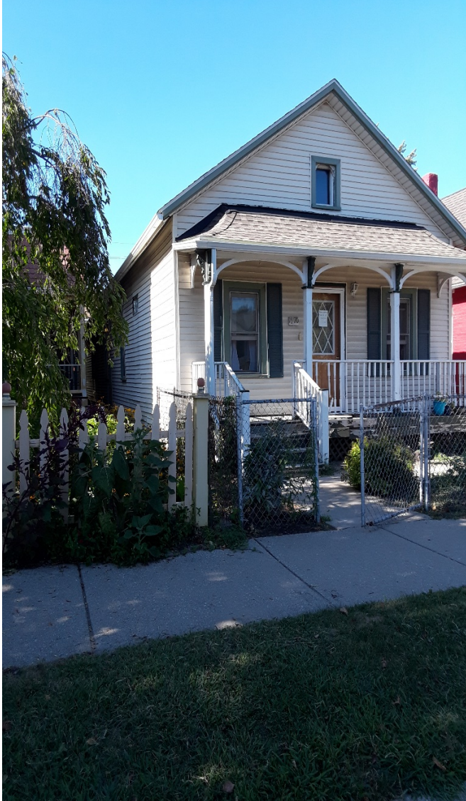
West corner of the front of the house. Metal gate and will be replanced by painted white wood gate and fence.
