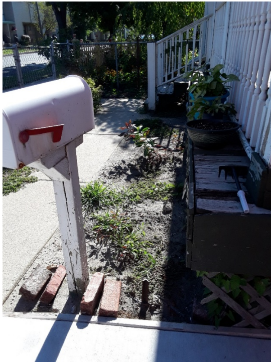
Porch floor is wider than overhang and rail.
