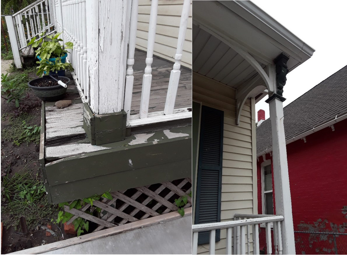
Corner of porch post and rail will go to corner of porch. Corbels will remain.
