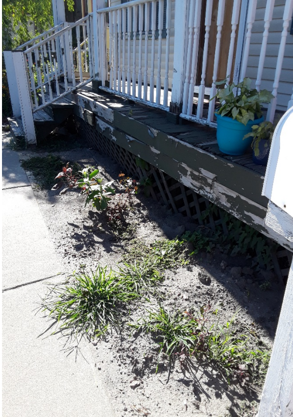
Front porch rail, skirt, and floor siding.
