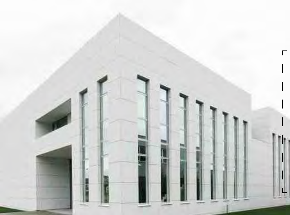
Office & production building | Spießberger Bau concrete skin in polar white with ferro
