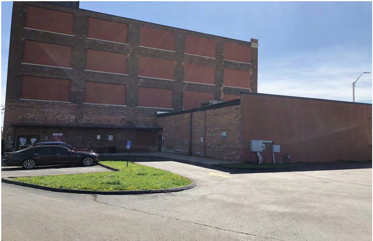
5716 MI AVE, West Elevation
