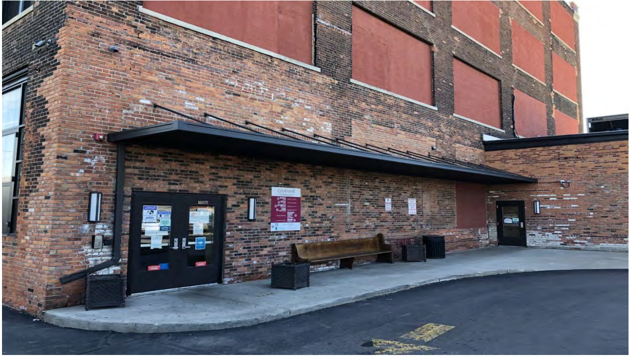
5716 MI AVE, West Elevation Entrance
