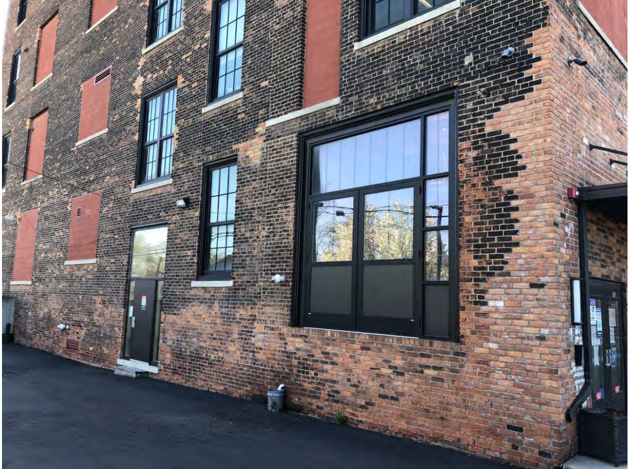
5716 MI AVE, North Elevation Close Up
