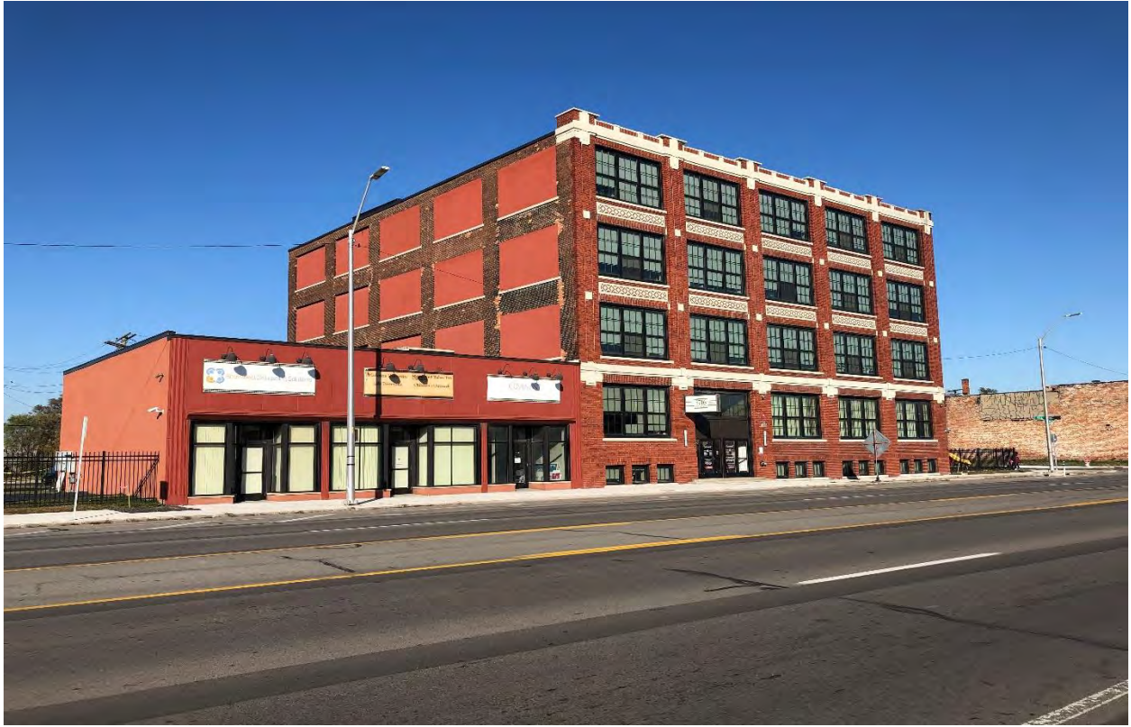
5716 MI AVE, South Elevation
