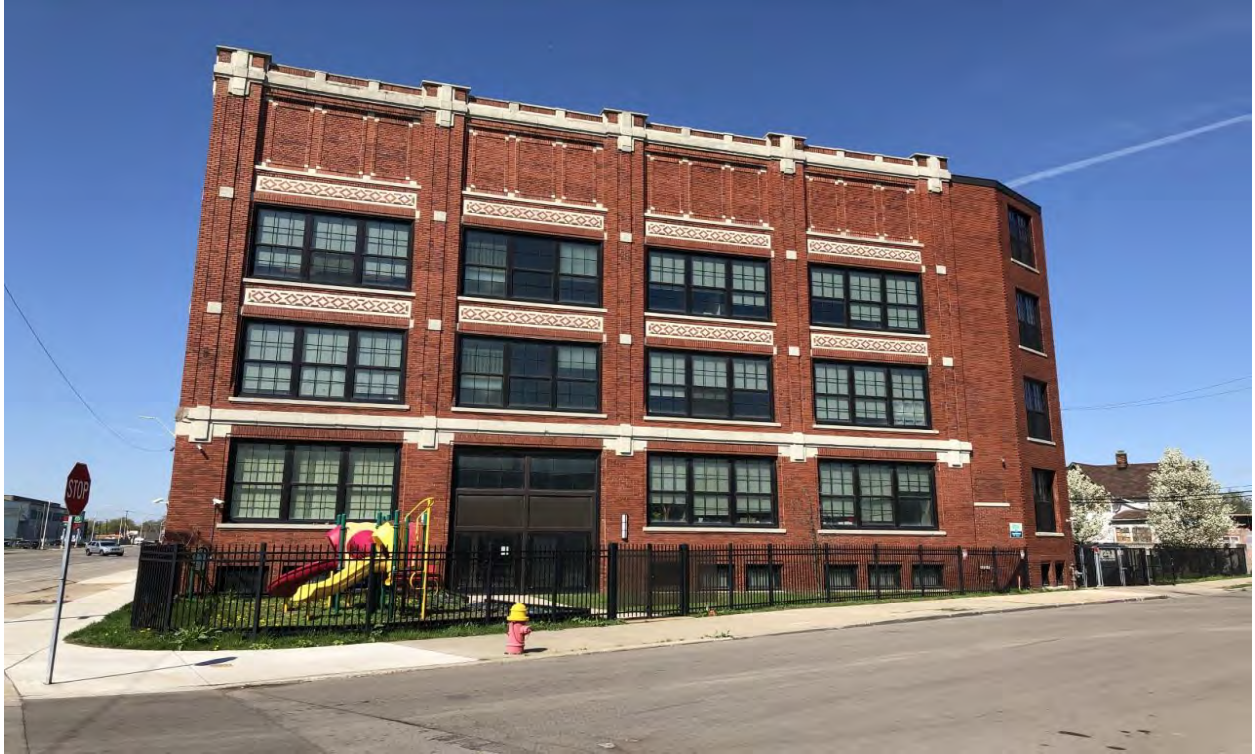
5716 MI AVE, East Elevation
