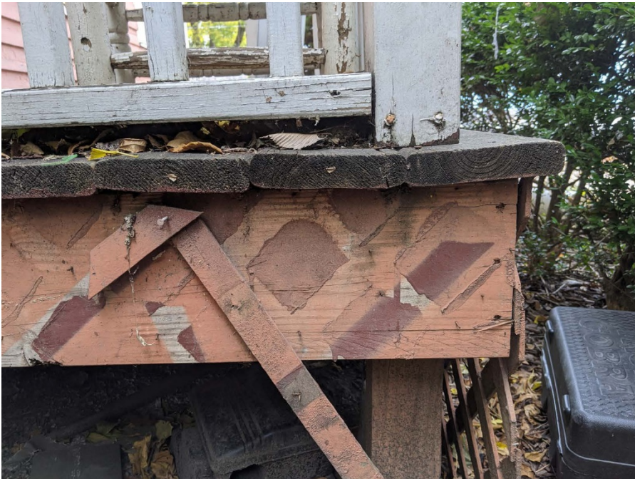
Porch Deck Detail
