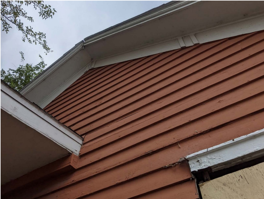
Porch Canopy Detail
