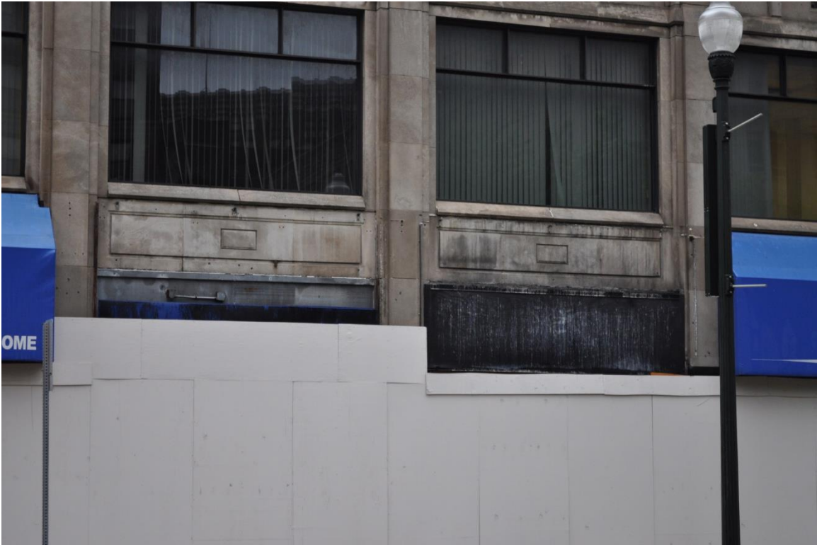
Figure #27: Exterior View of Storefronts. 7/3/2012
