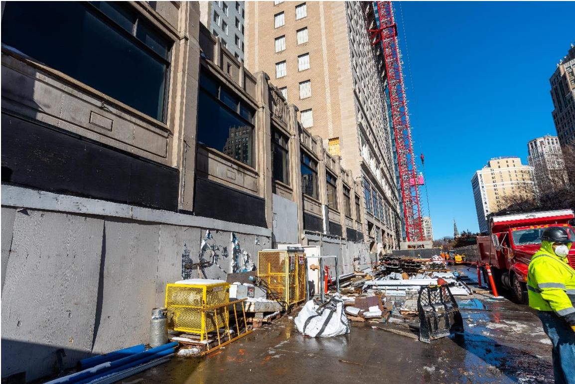
Figure #12: Exterior, Looking North. 12/2/20
