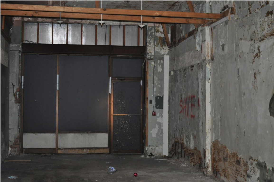
Figure #19: Interior View of Storefront. 5/8/2012
