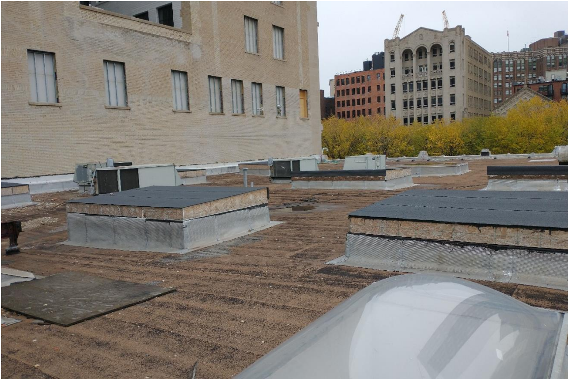
Figure #29: Exterior, Roof, Looking Northeast. 12/2/20
