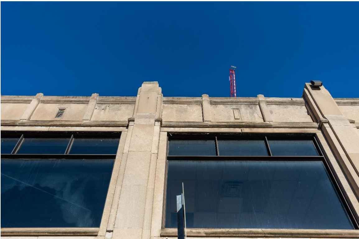
Figure #13: Exterior, Looking Up. 12/2/20
