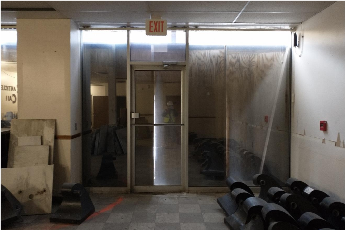
Figure #21: Interior View of Storefront. 10/30/2020
