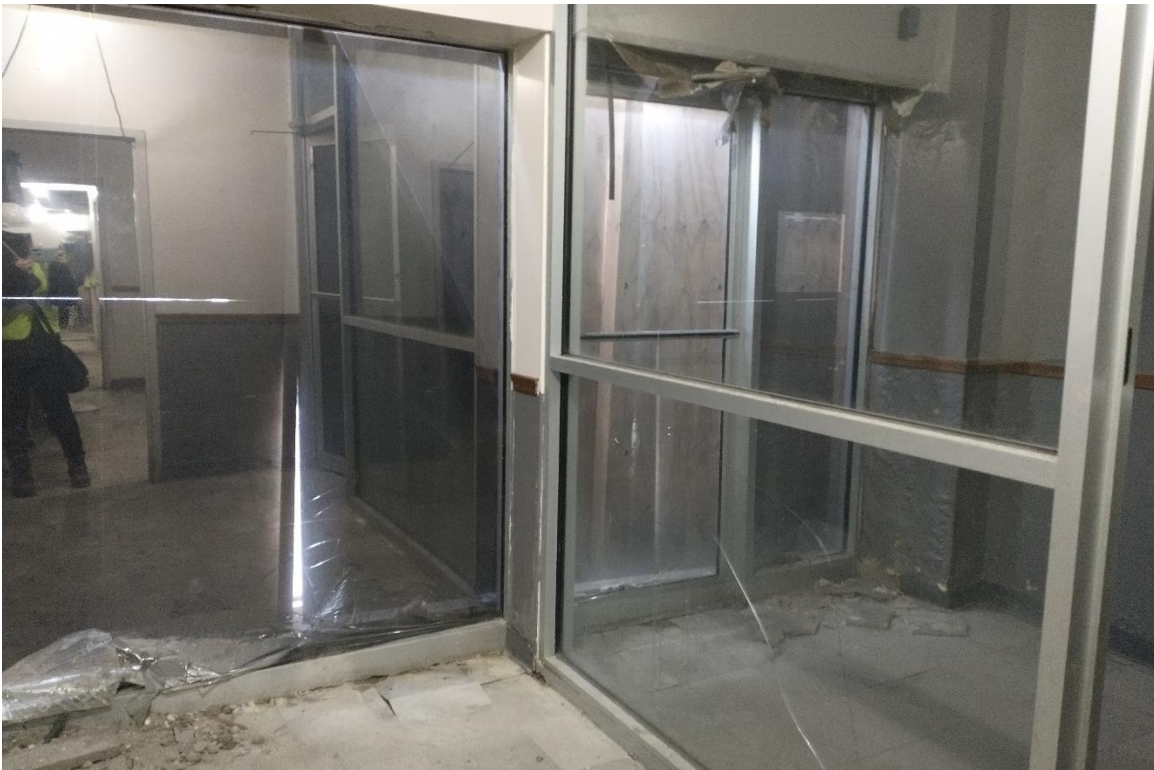
Figure #24: Interior View of Storefront and Entrance Door. 10/30/2020
