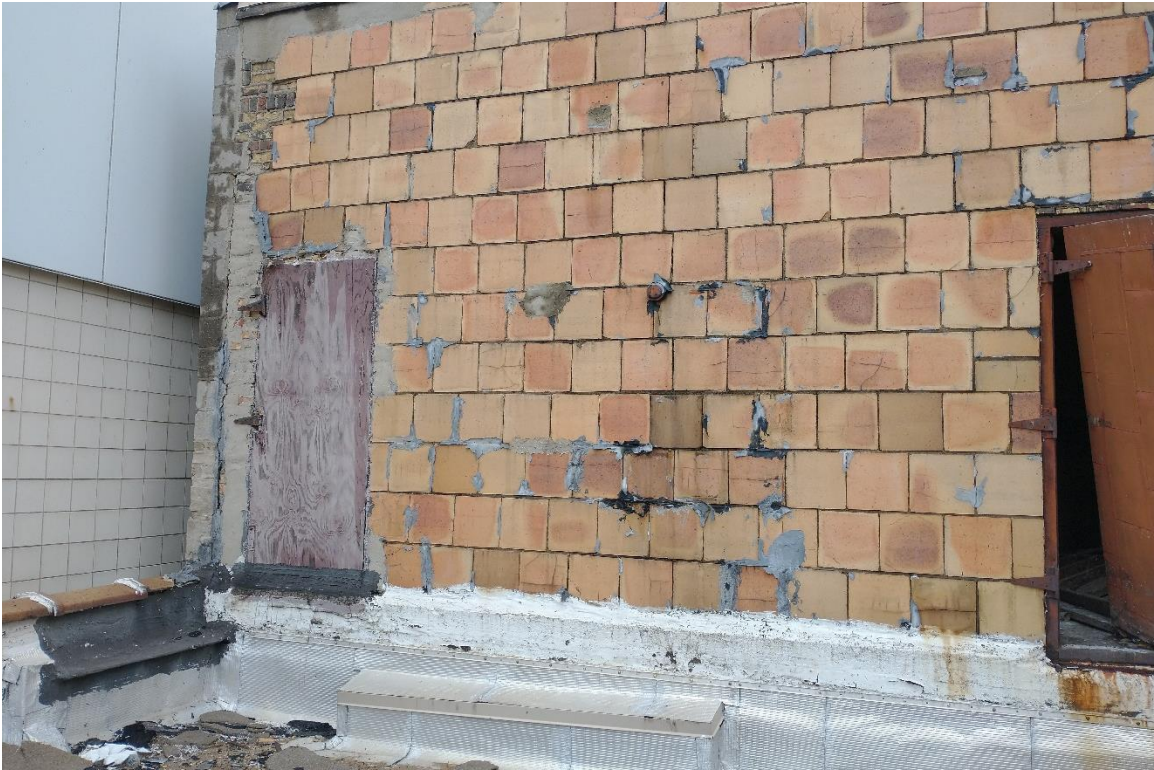
Figure #33: Exterior, Penthouse, Looking North. 12/2/20
