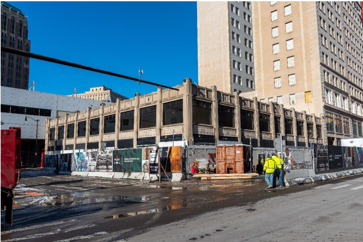
Figure #7: Exterior, Looking Northwest. 12/2/20
