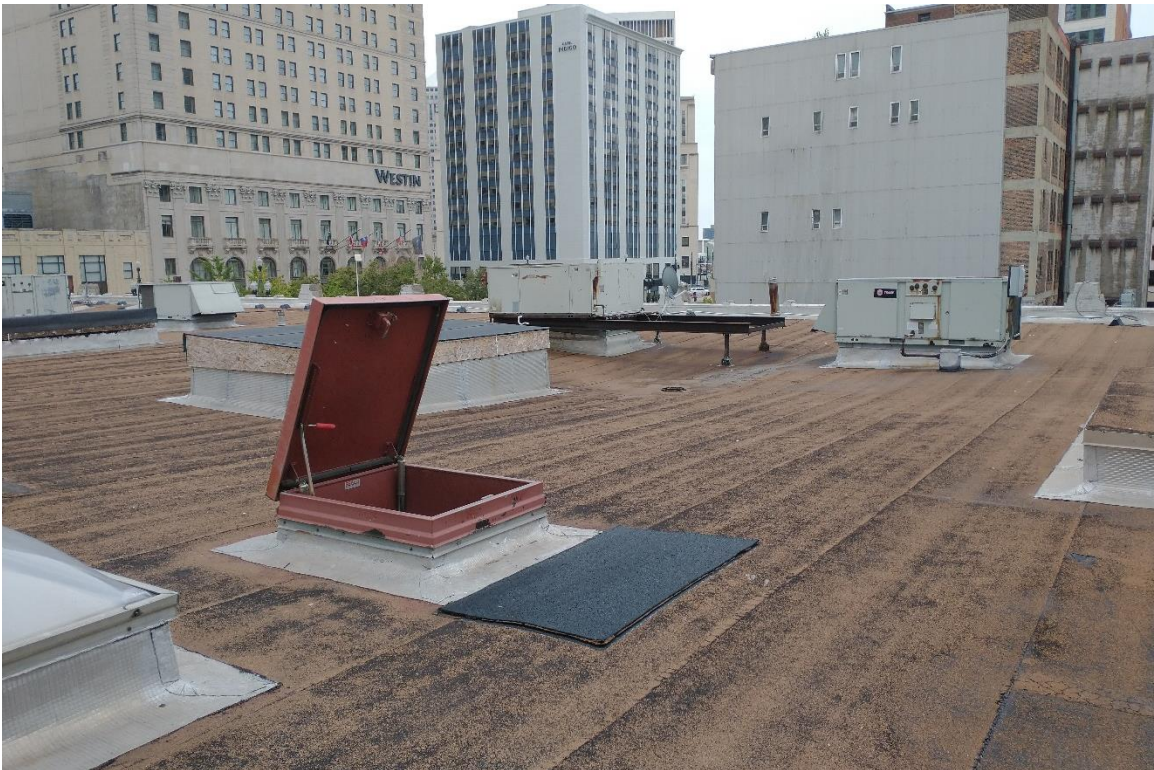
Figure #32: Exterior, Roof, Looking South. 12/2/20
