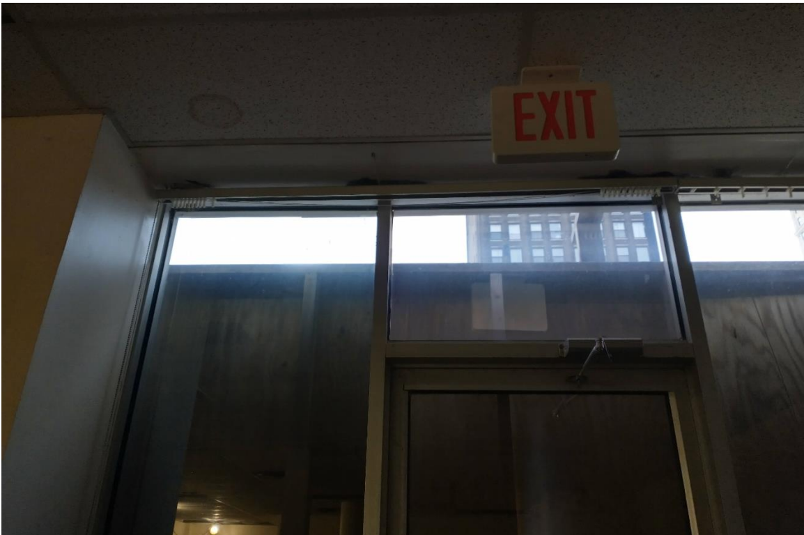
Figure #22: Interior View of Storefront. 10/30/2020
