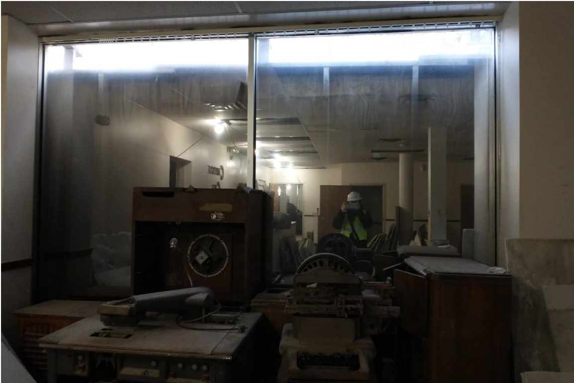
Figure #23: Interior View of Storefront. 10/30/2020
