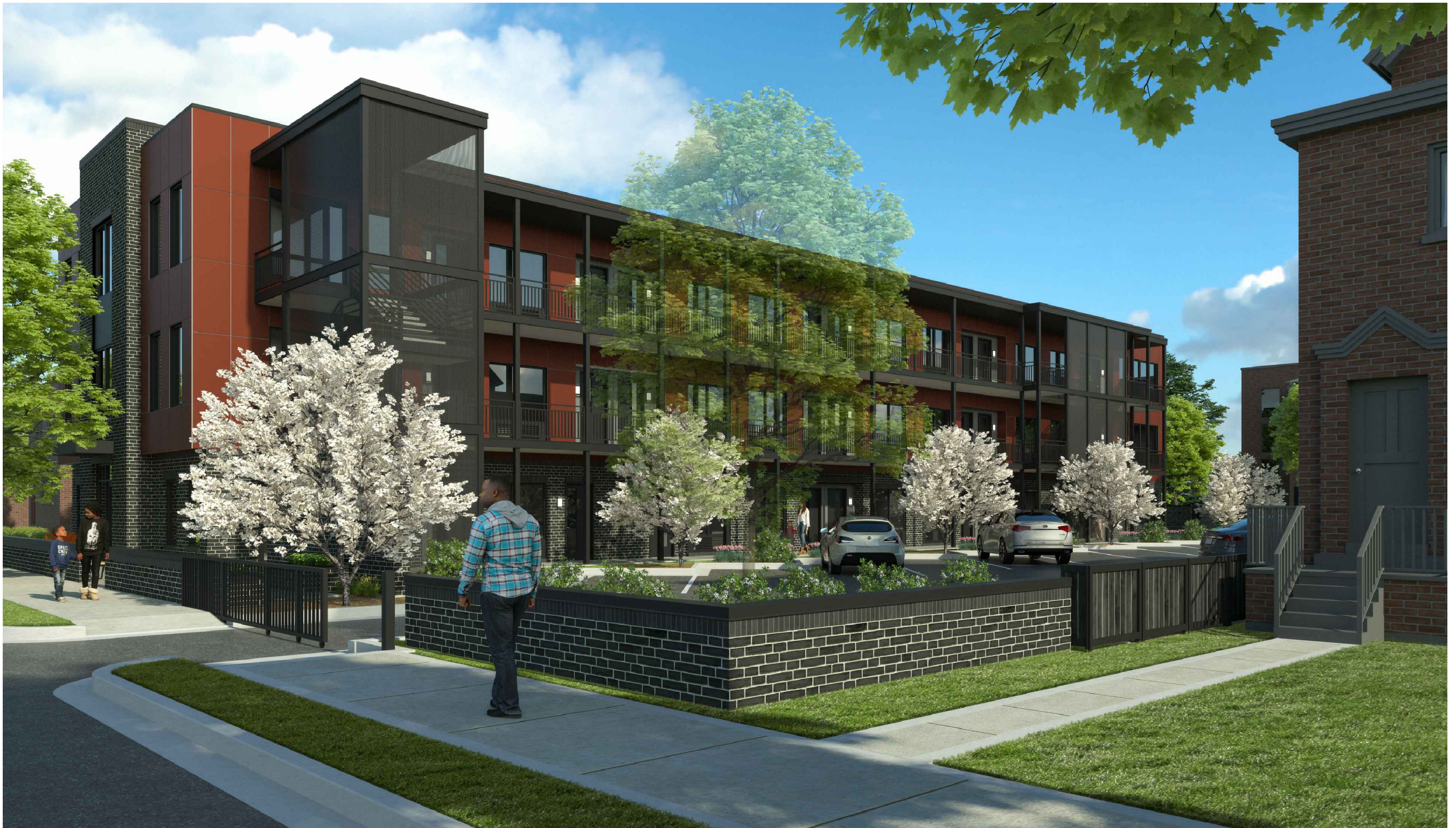
view from the southeast
