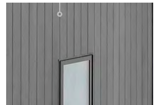
VESTA STEEL PLANK SIDING- IRONSTONE AT UNIT ENTRY ALCOVES
