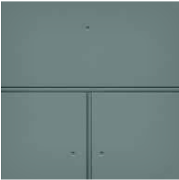
Reveal Exposed Fasteners
