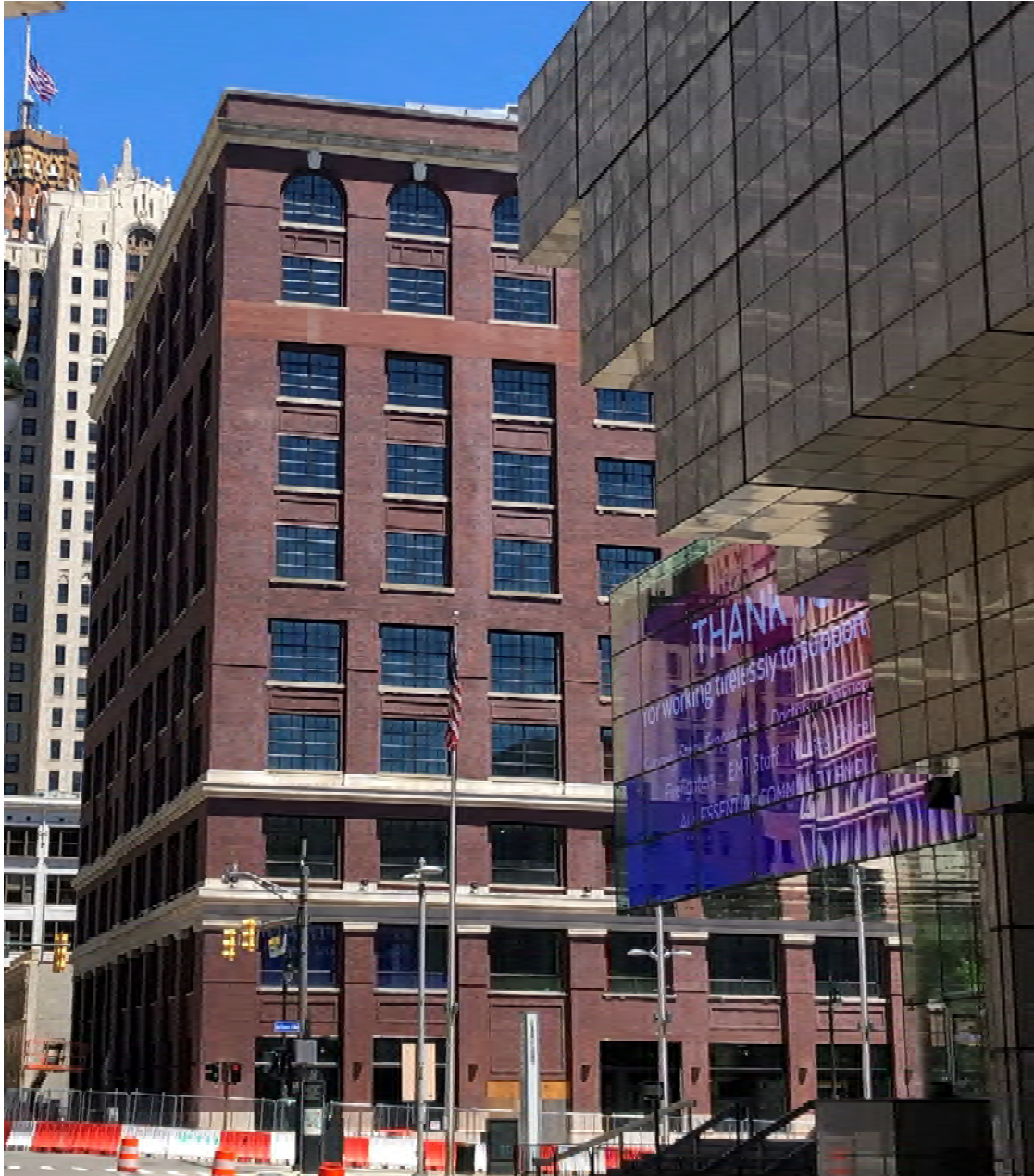
West Elevation looking east during construction.
