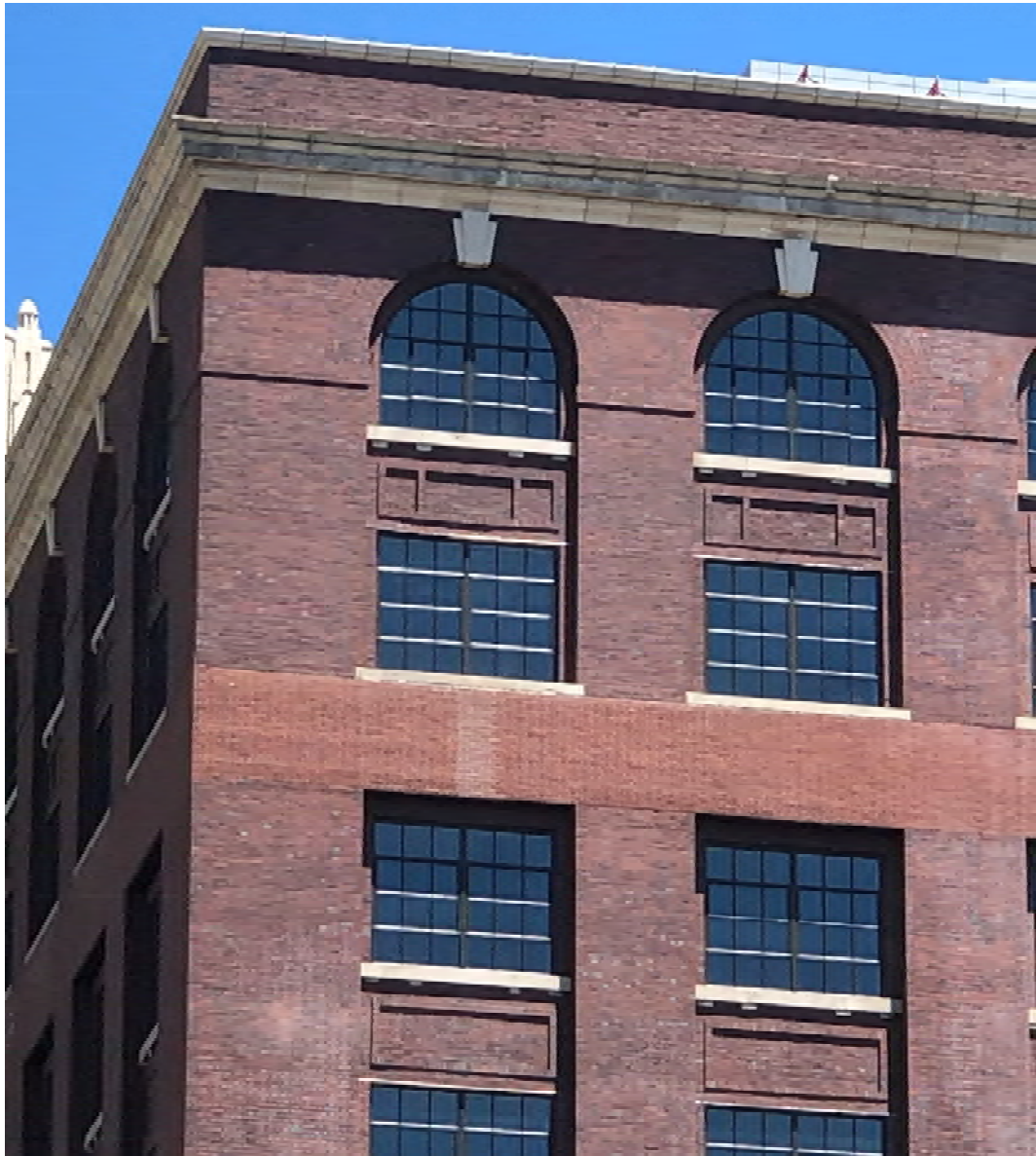
North end of parapet at west elevation during construction.
