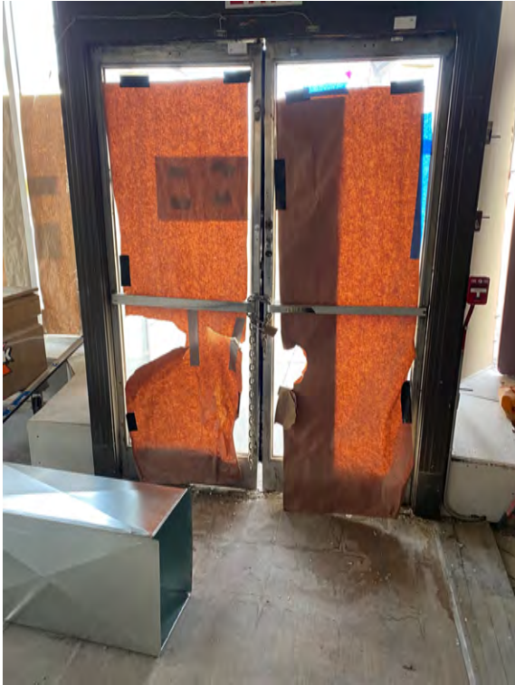
Existing Interior of doors
