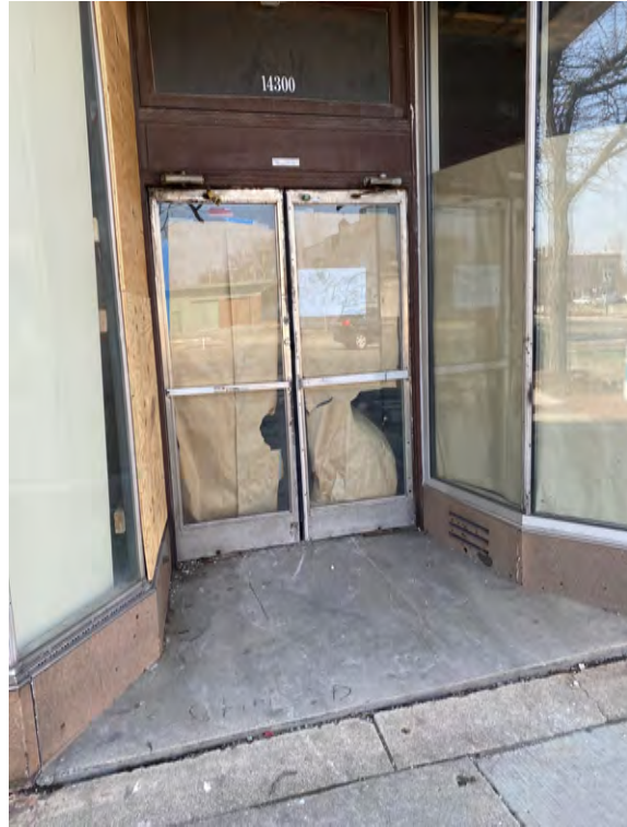
Existing Exterior of doors
