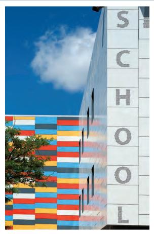
A stunning combination of functionality and aesthetics – the Perforated Panel Series provides necessary airflow and/or shade to a structure without sacrificing style or design. Virtually any shape and pattern can be perforated into the panels and used for a myriad of applications.
