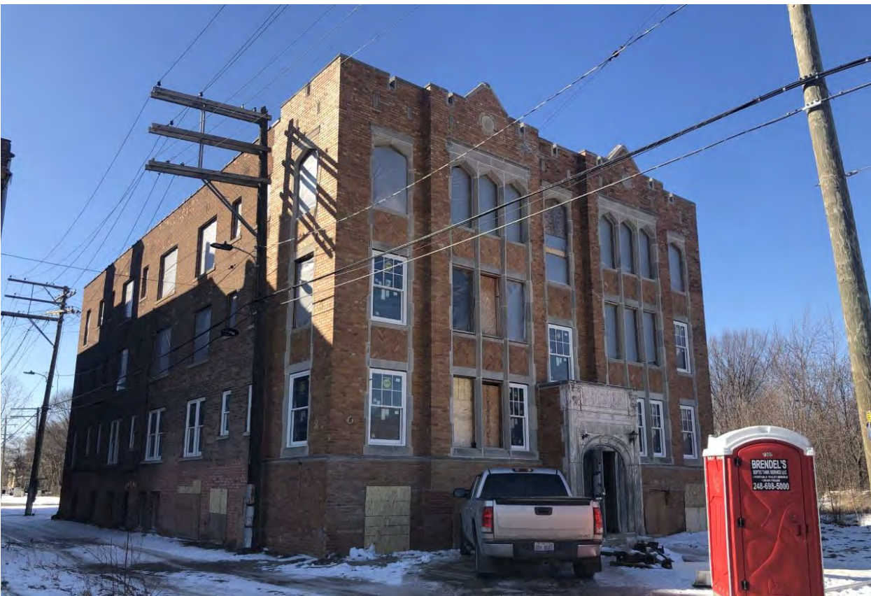
Double-Hung sash installed within the second floor landing should be eight-over-one.
