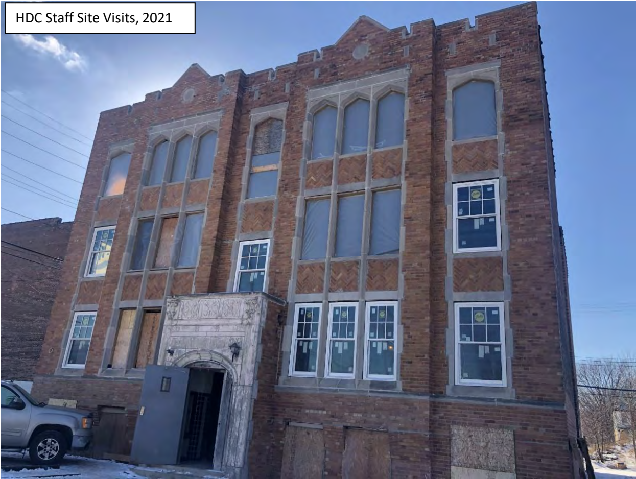
Double-Hung sash installed within the second floor landing should be eight-over-one.
