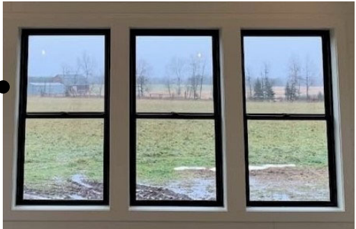
WINDOWS BLACK - SINGLE HUNG @ FIRST FLOOR UNITS
