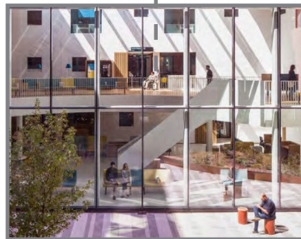
TWO-STORY GLASS CURTAIN WALL
