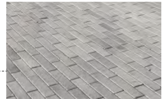
PERVIOUS PLANK PAVERS
