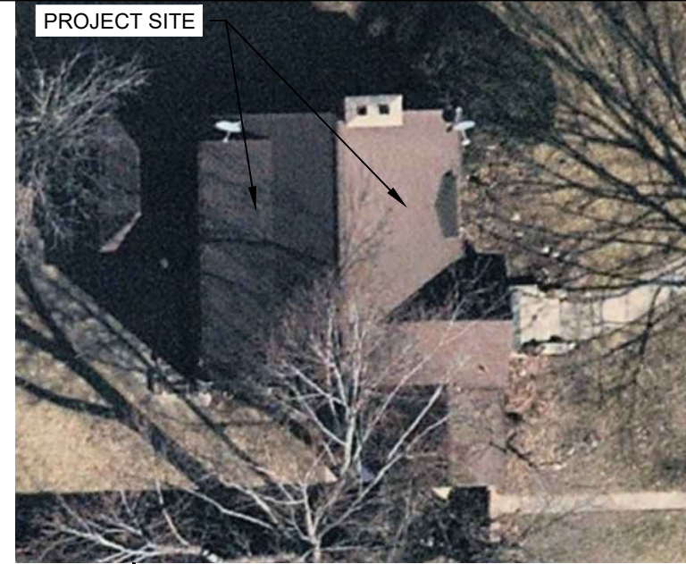
2 HOUSE PHOTO PV-1 | SCALE: NTS
