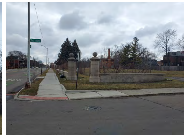
EXISTING STONE WALL AND DECORATIVE COLUMNS
