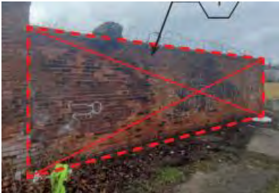
Photograph 3: East Masonry Wing Wall - North
