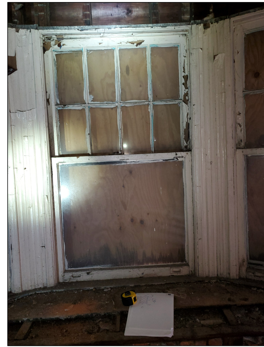
15 5A401 427 HENRY EXISTING PHOTO SCALE AS NOTED
