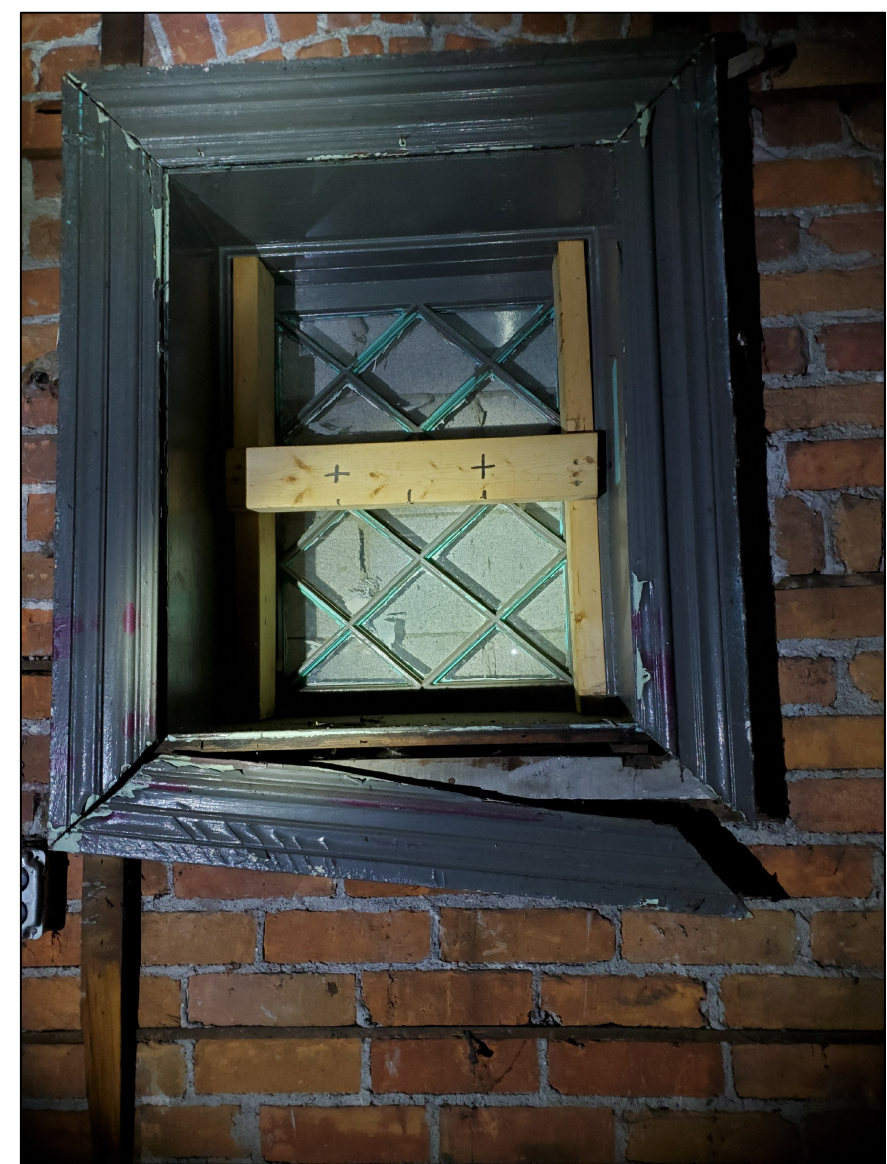
16 5A401 427 HENRY EXISTING PHOTO SCALE AS NOTED
