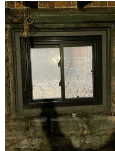
EXISTING BASEMENT VINYL WINDOW 7 (EAST)
