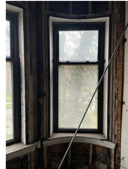
WINDOW 2C - EAST (INTERIOR) VINYL DOUBLE-HUNG
