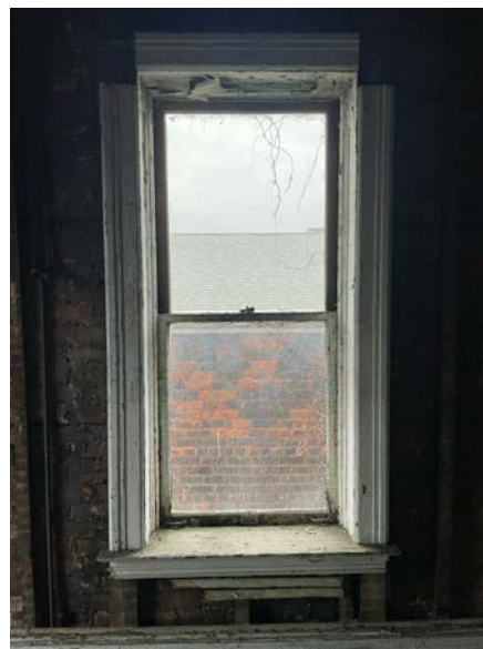
WINDOW 2G - WEST (INTERIOR) WOOD DOUBLE-HUNG
