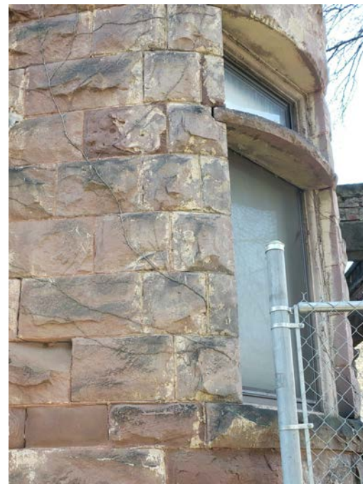
1C EAST - EXISTING EXTERIOR WOOD DOUBLE-HUNG
