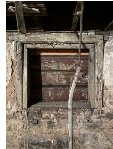
EXISTING BASEMENT WOOD WINDOW 5 (WEST)
