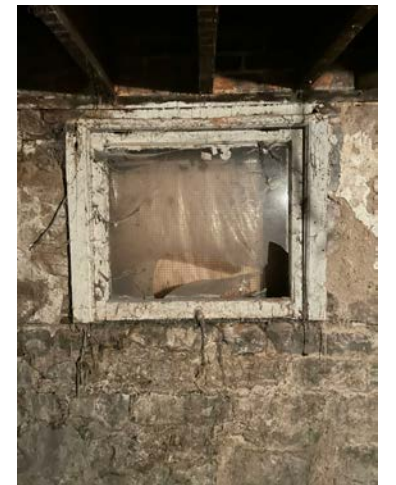
EXISTING BASEMENT WOOD WINDOW 4 (WEST)
