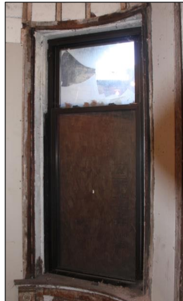
Front Elevation, 1 st Floor, Typical view vinyl replacement windows
