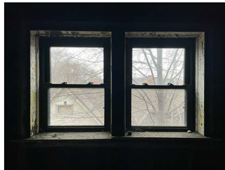
WINDOW 3C - EAST (INTERIOR) (2) VINYL DOUBLE-HUNG
