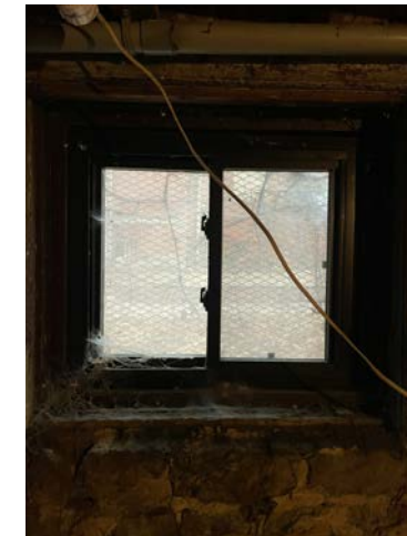
EXISTING BASEMENT VINYL WINDOW 8 (EAST)
