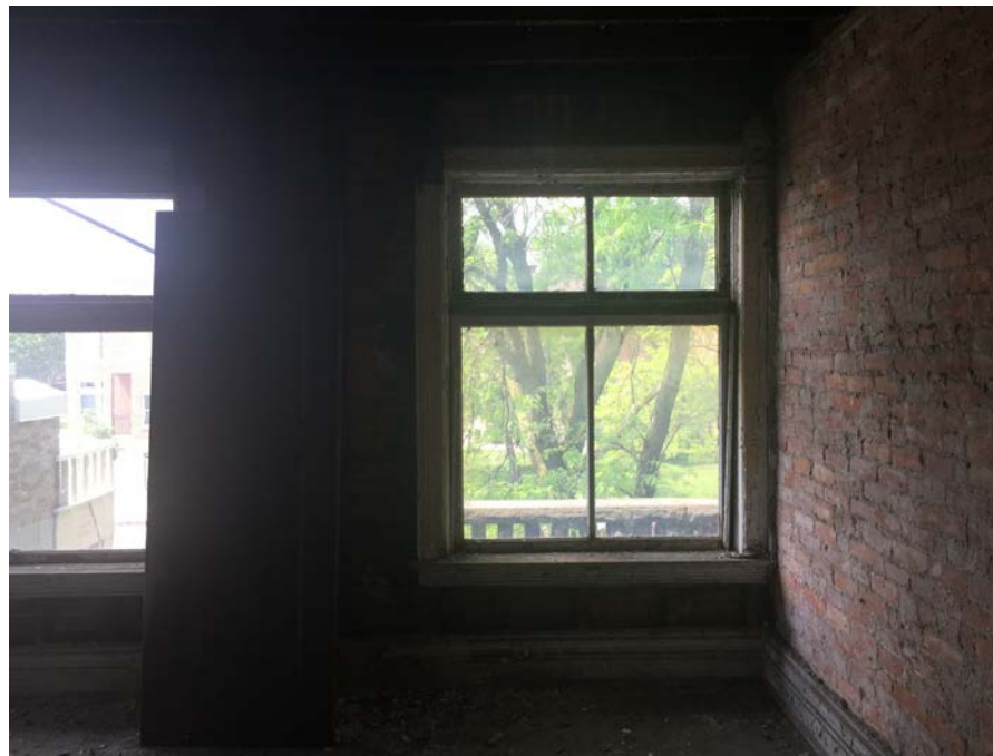
2. EXISTING WINDOW TYPE 2A (WEST)
