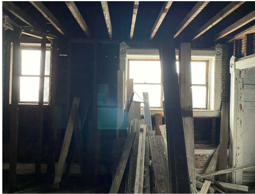
5. EXISTING WINDOW TYPES 3C & 3D (WEST)
