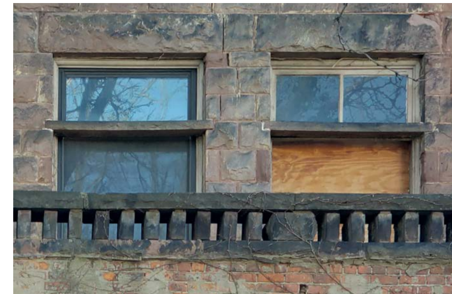
EXISTING WINDOW 2A EAST: VINYL DOUBLE-HUNG
