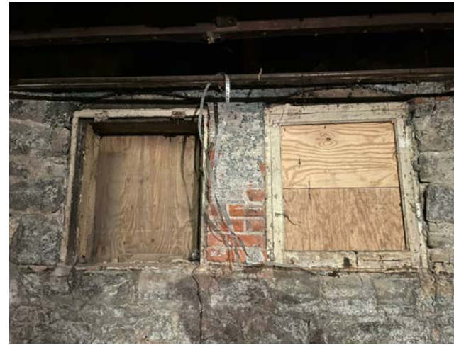
EXISTING BASEMENT WOOD WINDOWS 1 & 2 (WEST)
