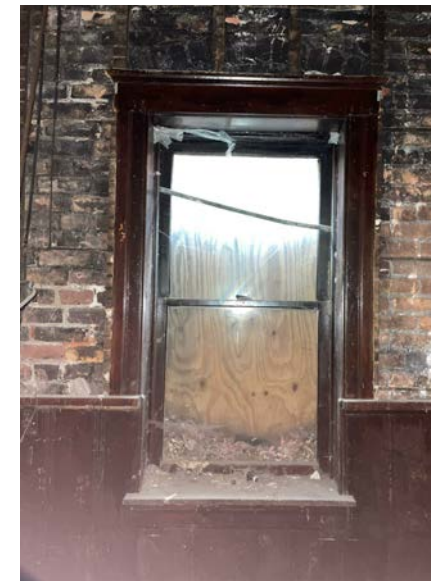
EXISTING WINDOW 1G - WEST WOOD DOUBLE-HUNG
