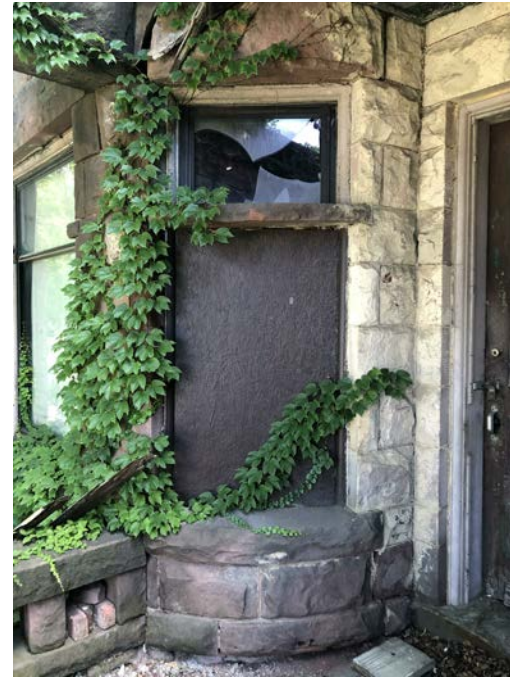
1A EAST - EXISTING EXTERIOR VINYL DOUBLE-HUNG
