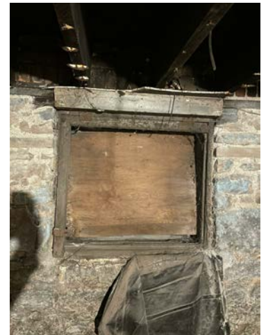
EXISTING BASEMENT WOOD WINDOW 4 (WEST)
