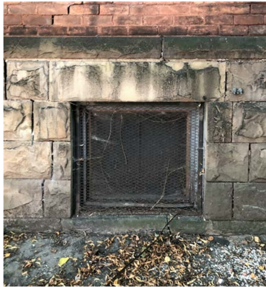
1. TYPICAL BASEMENT WINDOW EXTERIOR (EAST)
