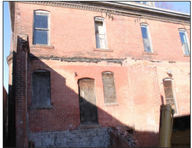
Rear Elevation of 701 W. Canfield
