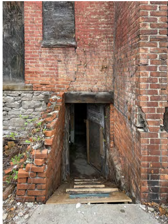
2. CENTER WALL AT SOUTH ELEV.
