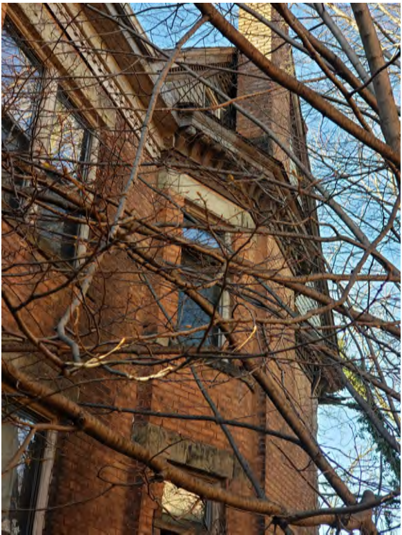
1. EAST ELEV. (TOWARD NORTH)
