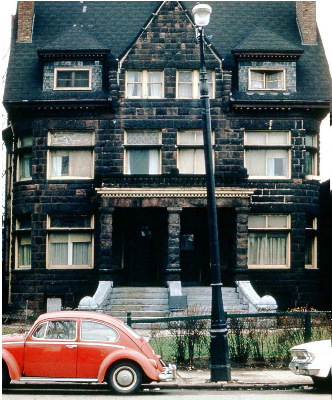
1. PHOTO FROM STREET - CA. 1970
