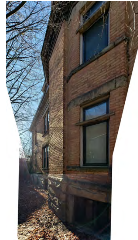
3. EAST ELEV. (TOWARD SOUTH)
