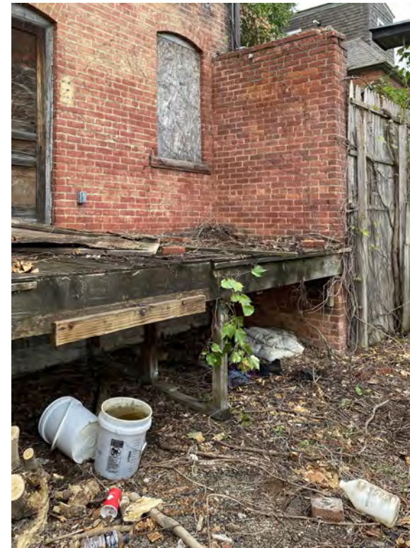
4. SIDE WALL AT SE CORNER
