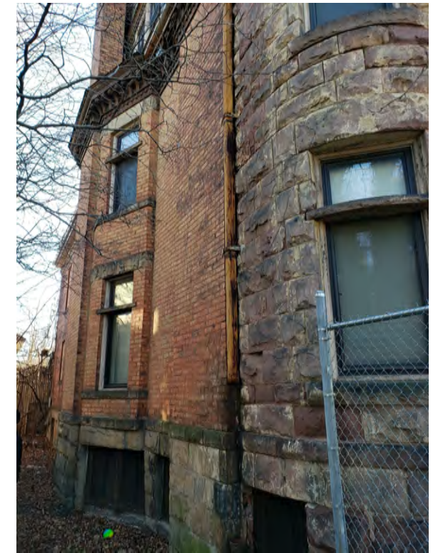
4. EAST ELEV. (TOWARD SOUTH)
