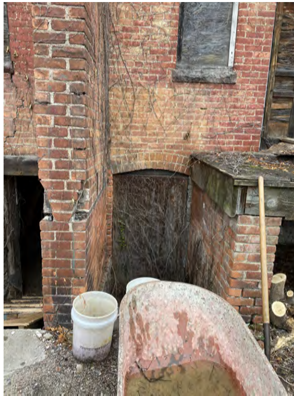
3. CENTER WALL AT SOUTH ELEV.
