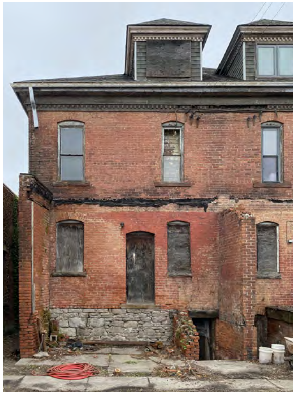
5. SOUTH FACADE - WEST SIDE
