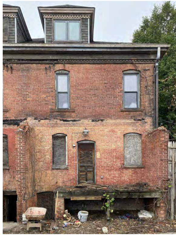
6. SOUTH FACADE - EAST SIDE
