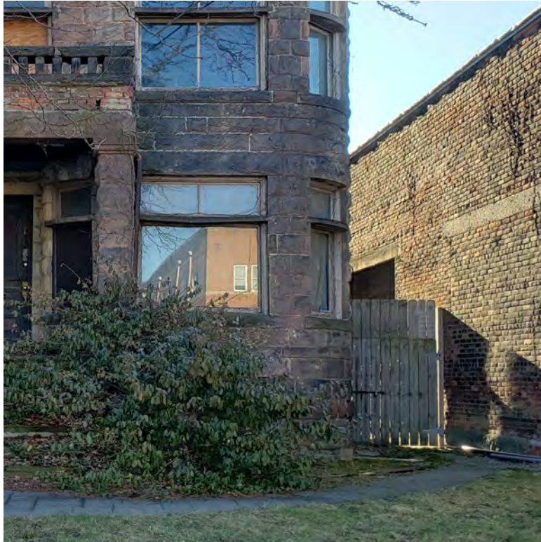
1. EXISTING FENCE AT NORTH (FRONT) FACADE
