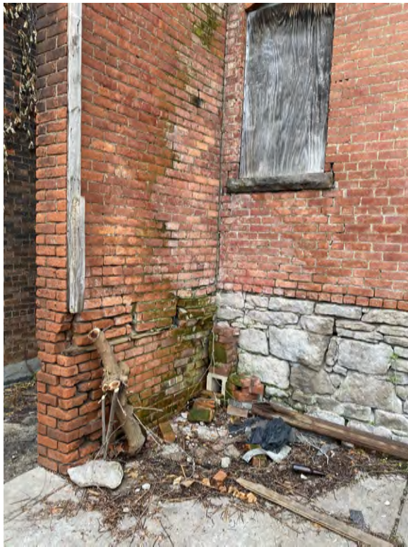
1. SIDE WALL AT SW CORNER
