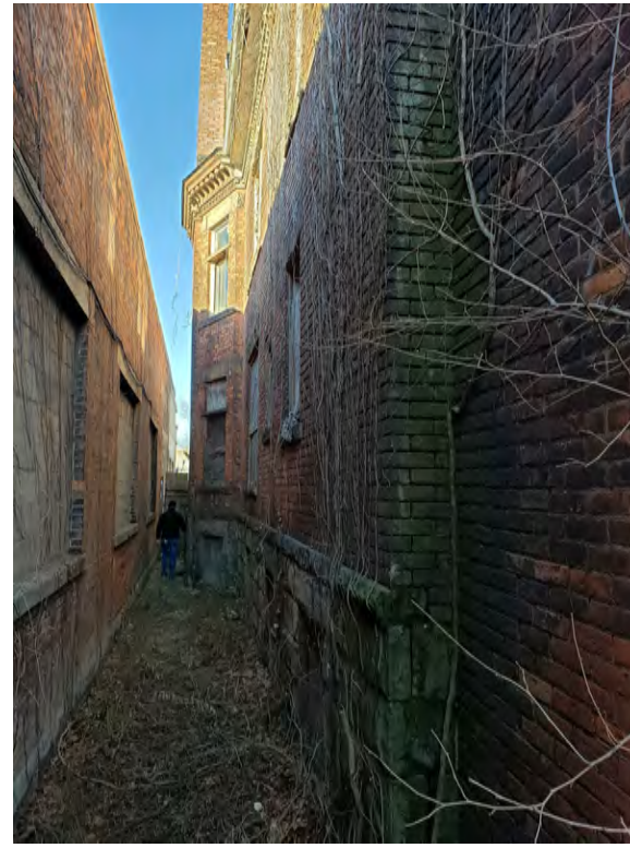
7. WEST ELEV. (TOWARD NORTH)
