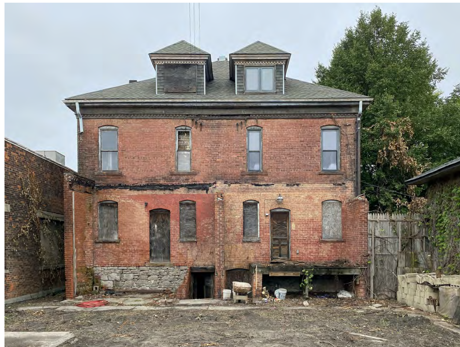
2. PHOTO FROM REAR - EXISTING CONDITIONS
