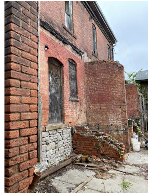
8. SOUTH FACADE - VIEW TO EAST
