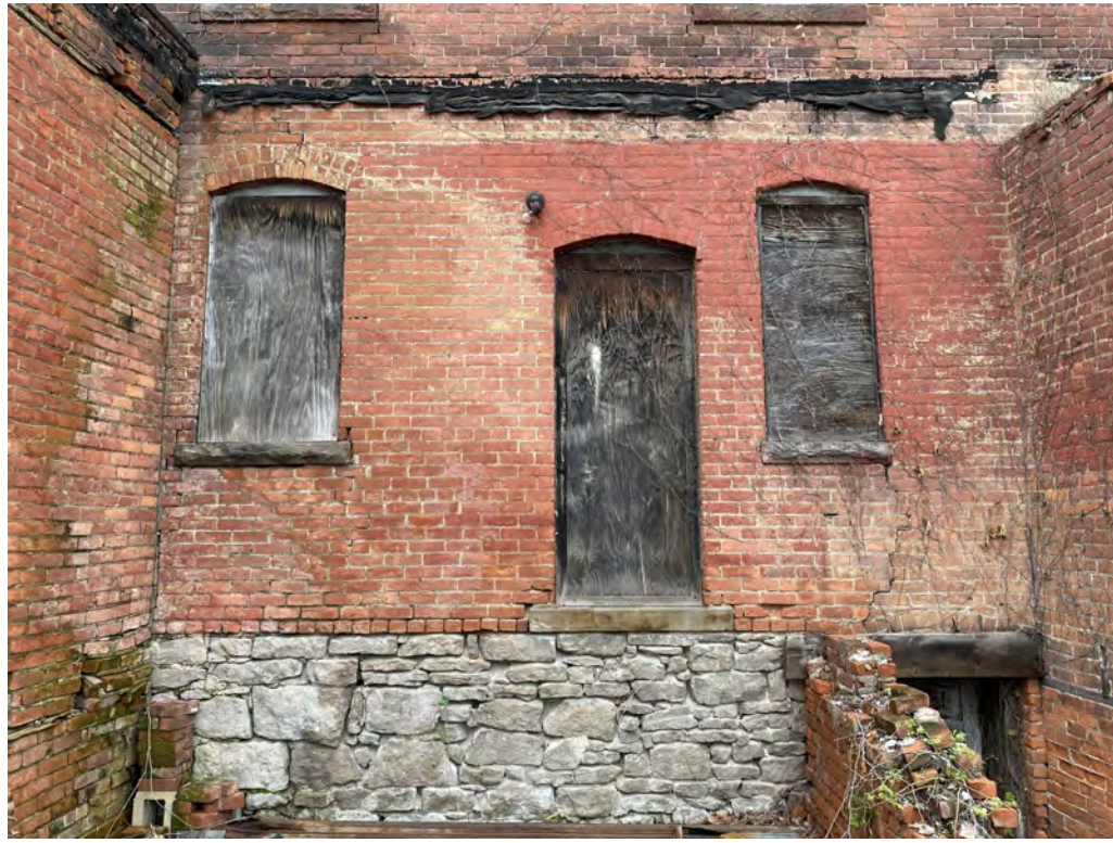
7. PARTIAL SOUTH FACADE - WEST SIDE
