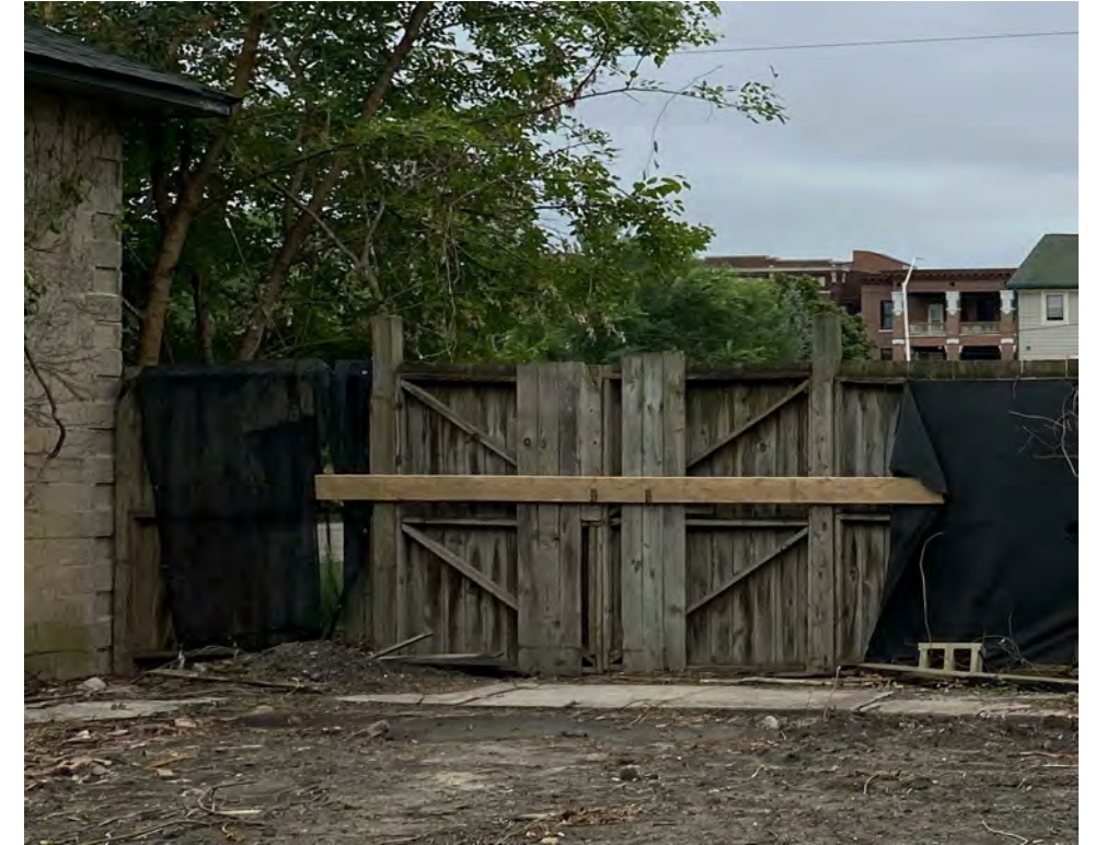
3. DETAIL PHOTOGRAPH OF EXISTING FENCE AT REAR
