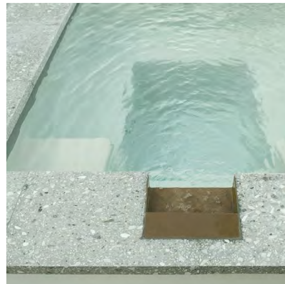
3. PROPOSED POOL EDGE MATERIAL 12" x 1-1/2" PRECAST TERRAZZO - GREY
