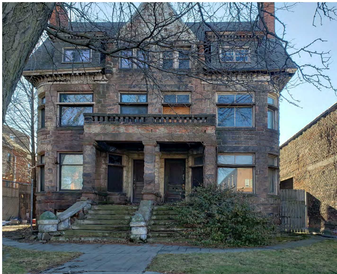
1. PHOTO FROM STREET - EXISTING CONDITIONS
