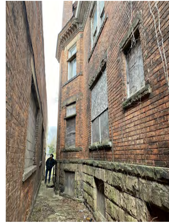
8. WEST ELEV. (TOWARD NORTH)
