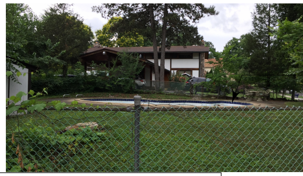
POOL TO BE REMOVED
