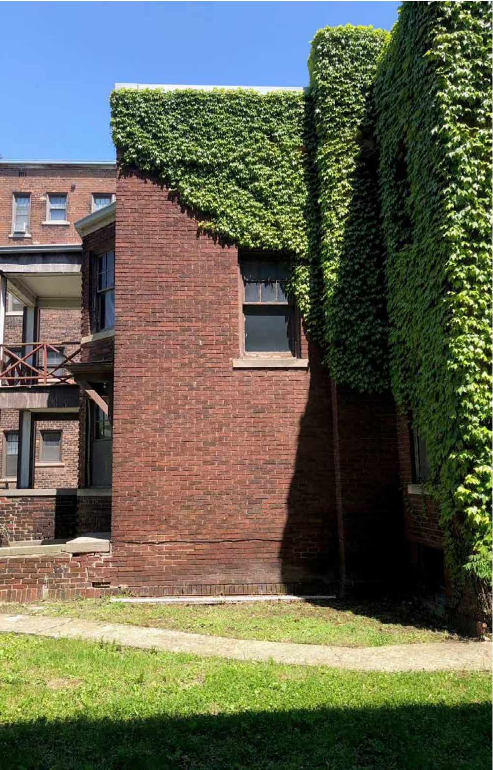
WEST FACADE (SIDE)
