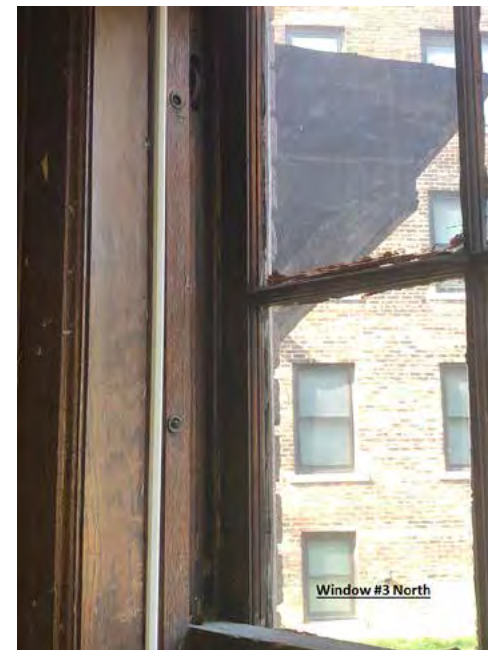
WINDOW F3 INTERIOR
