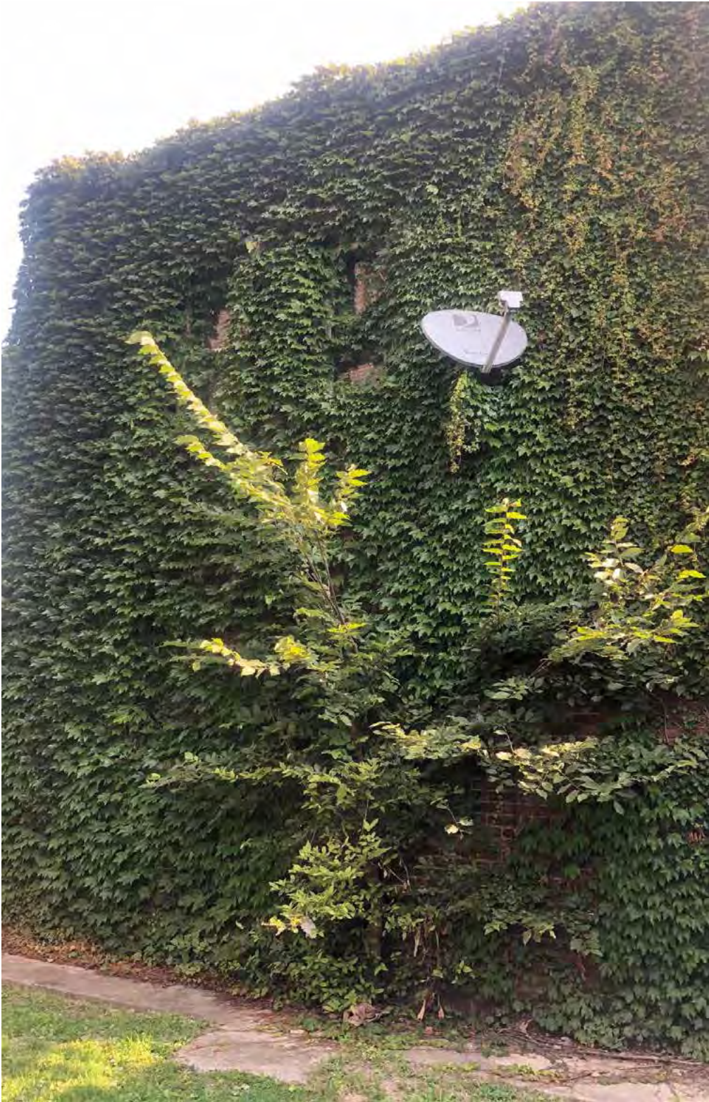
WEST FACADE (SIDE)
