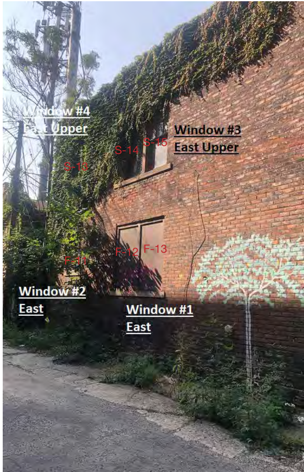
EAST FACADE (BACK)
