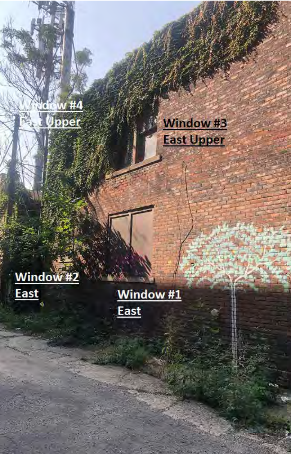
EAST FACADE (SIDE)
